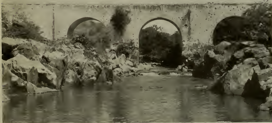
Massive Colonial stone bridge on the historic Borda Stone Highway, between Cuernavaca and Taxco, on the main route from Mexico City to Acapulco. Note shrubbery growing out of the masonry, nourished by heavy seasonal rains. Photograph by the author.
