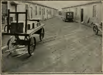
San Francisco Ferry Building Dock—floored with Port Orford Cedar nine years ago. Constant jar and the wear of steel-tired trucks have affected it but little.
