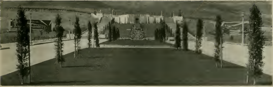
THE MALL AND CASCADE, MIDWICK VIEW ESTATES, MONTEREY PARK, CALIFORNIA Cook, Hall and Cornell, Landscape Architects
