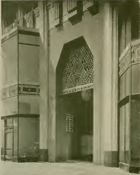
DETAIL OF MAIN ENTRANCE
