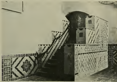
Stairway of Tunisian Tile with Floors and Steps of Fallston Tile Santa Barbara Courthouse Wm. Mooser, Architect
