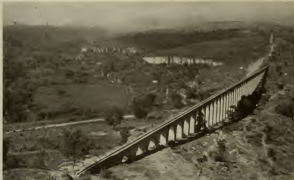
The Aqueduct of Los Remedios, built in 1916 is a vast structure of hard, white volcanic stone. A thousand feet long with fifty arches ranging up to sixty feet high, it spans a saddle between two great canyons. Photograph by author.
