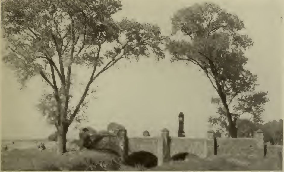
A stone bridge less than one century old, in Spanish Colonial spirit, which spans a creek on the Pachuca Highway. Two great white poplars enframe the structure. Photograph by the author.
