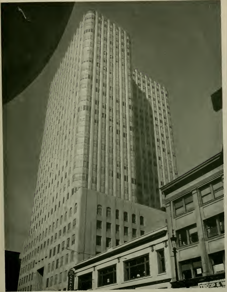
FOUR FIFTY SUTTER, SAN FRANCISCO, CALIFORNIA J. R. MILLER AND T. L. PFLUEGER, ARCHITECTS
