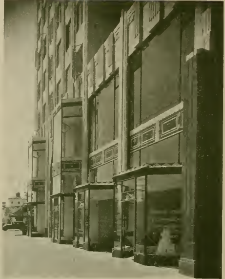
DETAIL OF STORE FRONT
