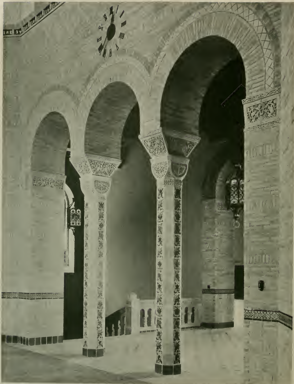
Showing the Possibilities of Decorative Tile with Terra Cotta and Brick
