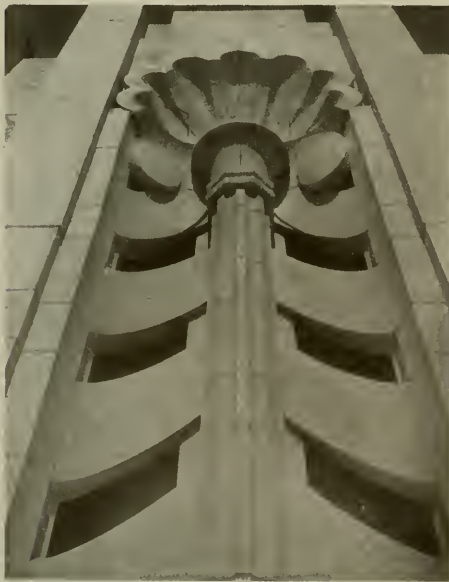
DETAIL OF SPANDREL, SHELL BUILDING Geo. W. Kelham, Architect
