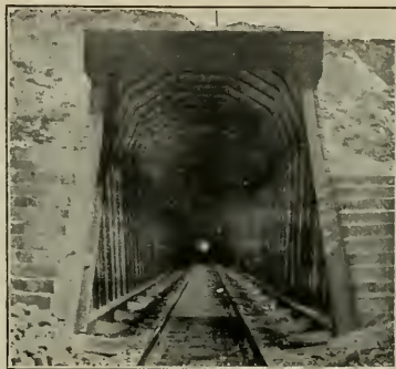
Port Orford Cedar is selected for tunnels of the Western Pacific. This photo shows portals and inside timbers in a tunnel on the line in San Francisco.
