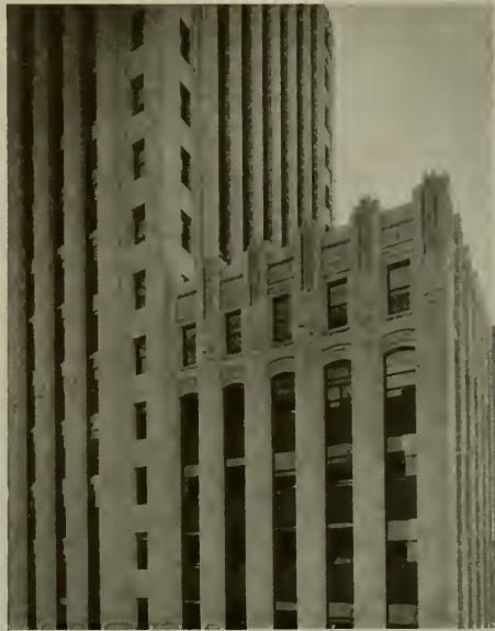
DETAIL, UPPER STORY WING, SHELL BUILDING Geo. W. Kelham, Architect
