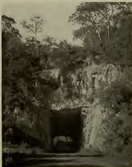
Tunnel cut through solid stone, in wild Zopelote Canyon, in the State of Guerrero, on the major highway from Mexico City to Acapulco, one of the finest natural harbors on the Pacific. Photograph, courtesy of National Highway Commission of Mexico.
