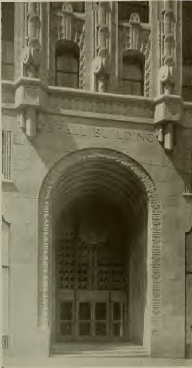
ENTRANCE DETAIL, SHELL BUILDING, SAN FRANCISCO
