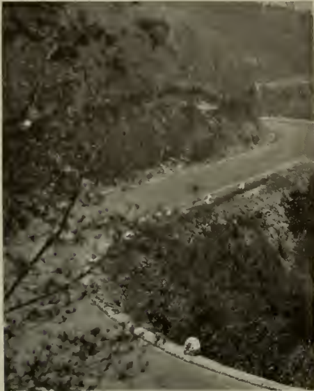
The Puebla Highway, superb engineering through magnificent scenery, on the climb out of the Valley of Mexico, eastward to the mountain divide beyond which lies the Valley of Puebla. Photograph, courtesy of National Highway Commission of Mexico.
