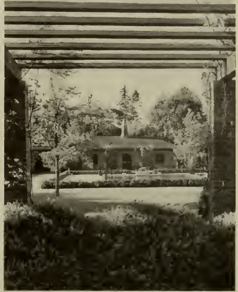
BATH HOUSE, ESTATE OF M. LLOYD FRANK Herman Brookman, Architect
