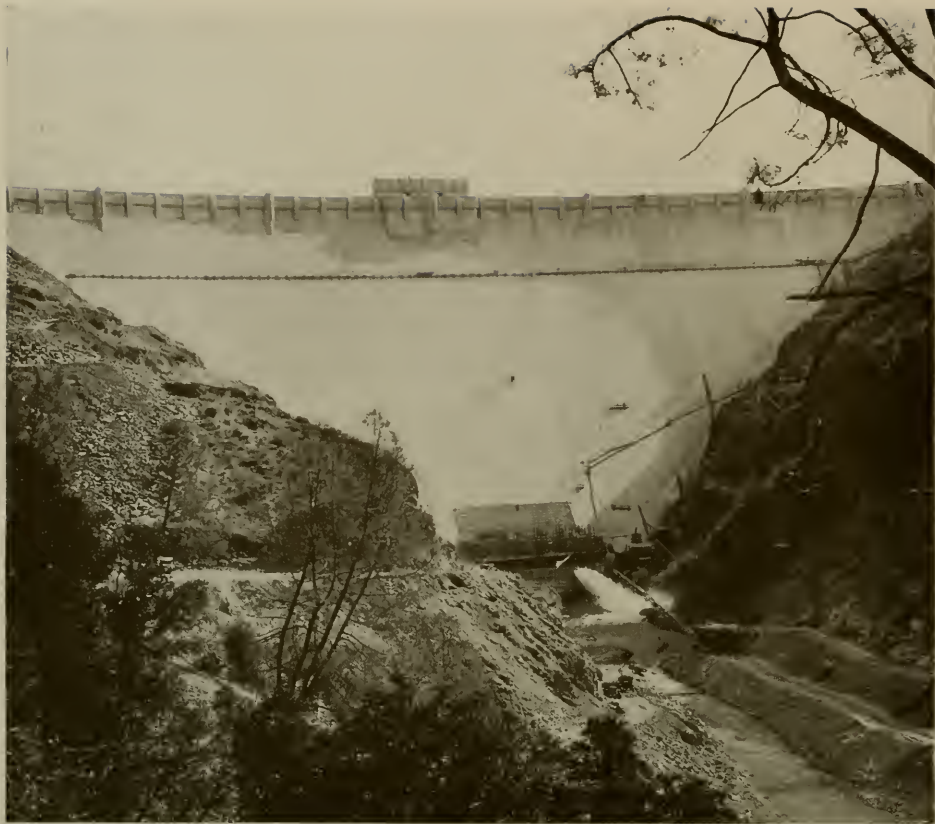
CLOSE-UP OF PARDEE DAM UNDER CONSTRUCTION
