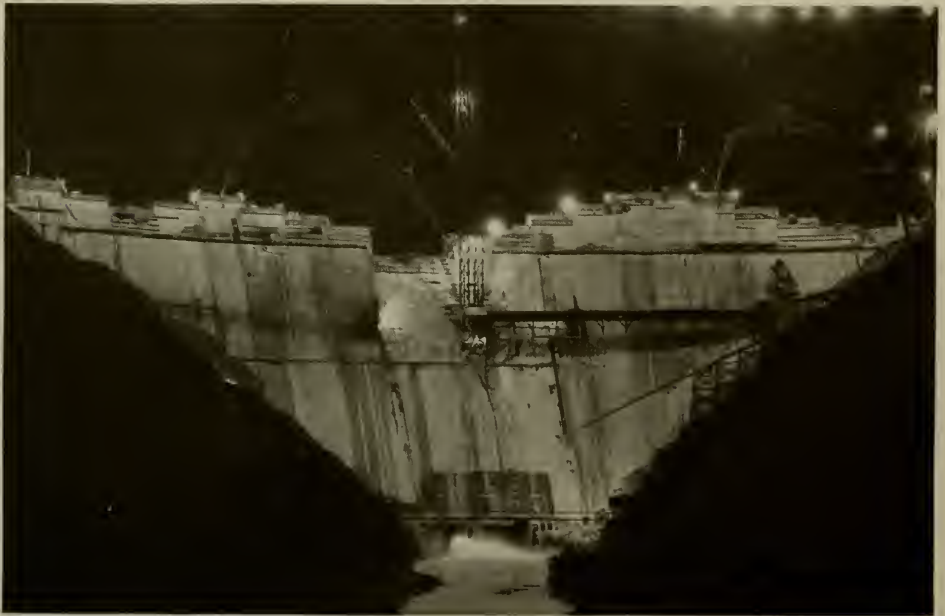
PROGRESS WORK ON PARDEE DAM BY ARTIFICIAL ILLUMINATION
