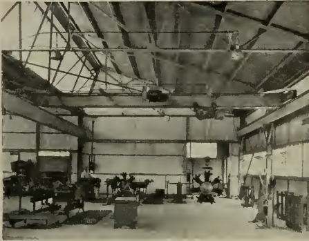
Interior showing wide clearances and ample lighting in CSC industrial steel units
