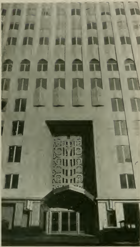
LOWER STORY DETAIL, FOUR FIFTY SUTTER J. R. Miller and T. L. Pfeuffer, Architects
