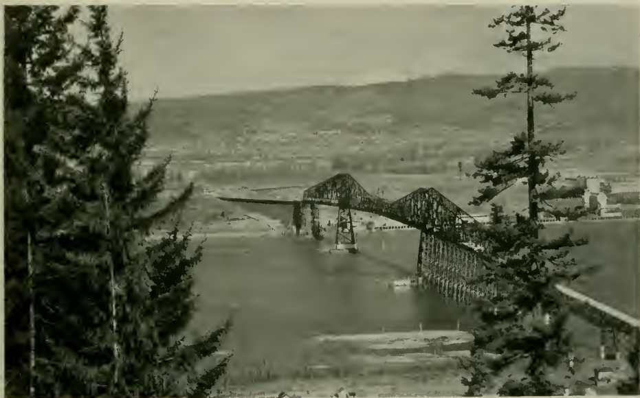
COLUMBIA RIVER LONGVIEW BRIDGE, BUILT AT COST OF $5,800,000 Bethlehem Steel Company, Steel Fabricators
