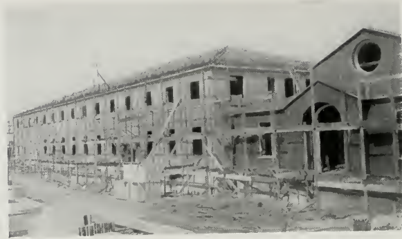
EXTERIOR OF MAIN BUILDING READY FOR PLASTERING
