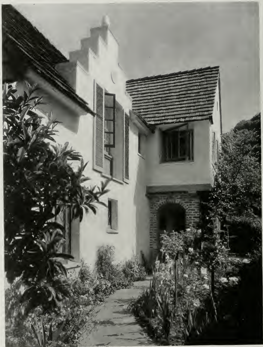
HOUSE OF MR. AND MRS. G. W. LUBOWSKI, BERKELEY, CALIFORNIA W. R. YELLAND, ARCHITECT
