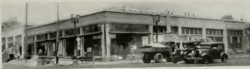
STORE BUILDING OF MRS. MABEL L. BIRELEY, HOLLYWOOD, BEFORE ALTERATIONS
