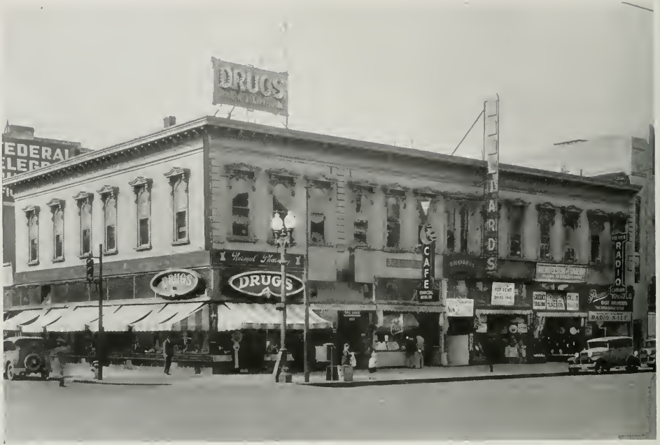
JONAS BUILDING, OAKLAND, CALIFORNIA, BEFORE ALTERATIONS
