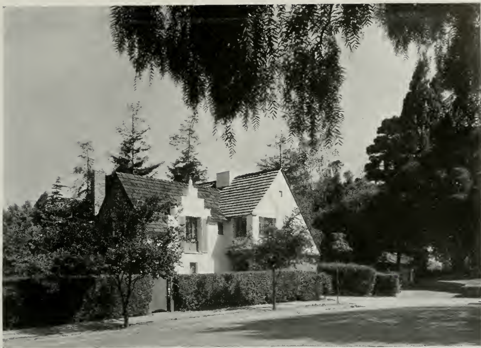
HOUSE OF MR. AND MRS. G. W. LUBOWSKI, BERKELEY, CALIFORNIA W. R. Yelland, Architect
