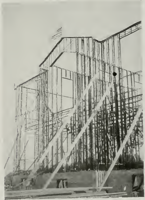
END WALLS COMPLETED AND READY FOR ROOF JOISTS
