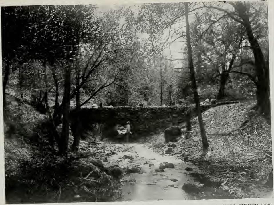
A FOREST GLADE IN BUTTE COUNTY, CALIFORNIA, INTO WHICH THE METAL ARCH AND RUBBLE HEADWALL HARMONIZE WELL
