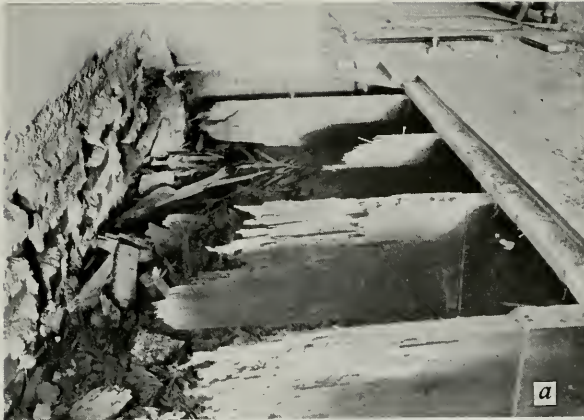
Fig. 26—Work of ground dwelling termites in a building in Fresno, California. a—Joists. b—In flooring and subflooring. The joists were almost on the ground and placed in a masonry wall without proper ventilation.
