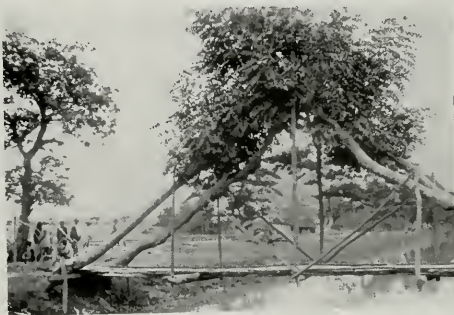
A PICTURESQUE "NATURAL" BRIDGE IN JAVA. The tops of four trees, two growing on each bank, were joined to form the truss.
