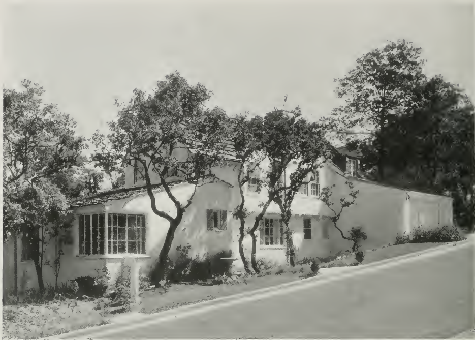
HOUSE OF MR. AND MRS. HERMAN H. BISHOPRIC, WILDWOOD GARDENS, PIEDMONT, CALIFORNIA W. R. Yelland, Architect
