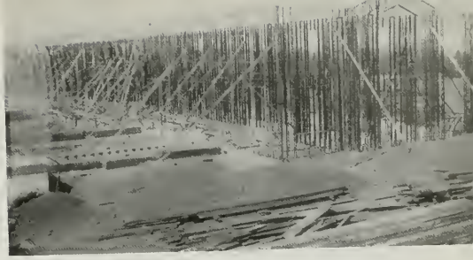
WALL FRAME ERECTED READY TO RECEIVE FLOOR JOISTS
