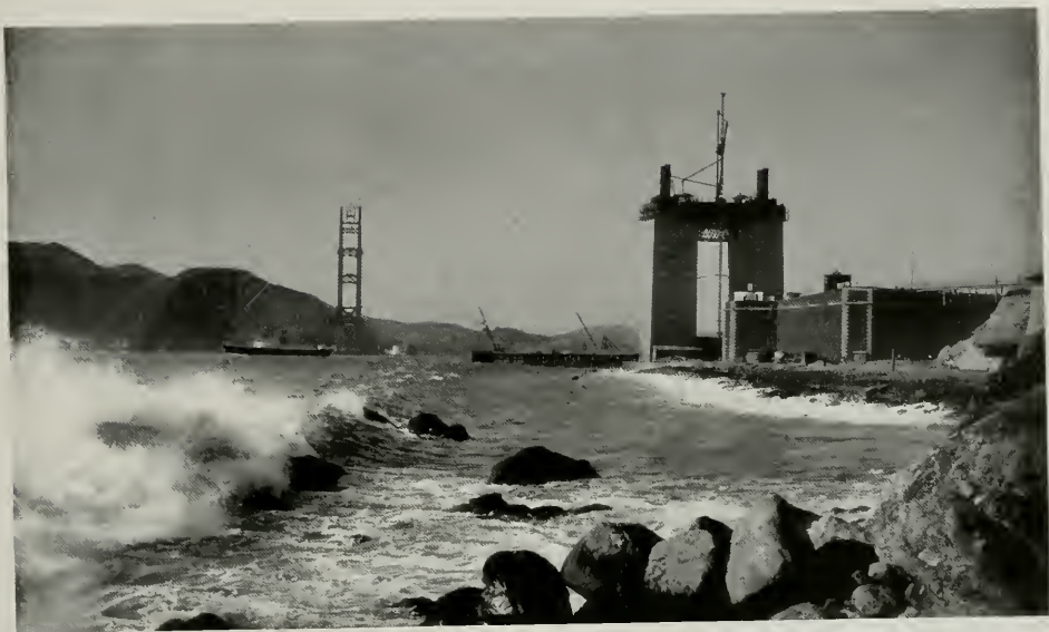
PYLON S 1, FORT POINT, SAN FRANCISCO. MARIN TOWER IN THE DISTANCE
