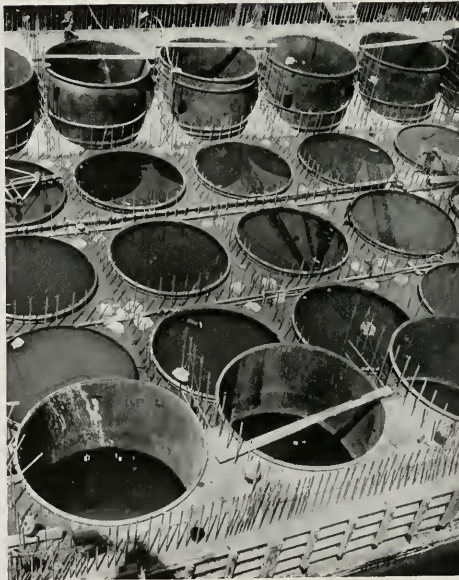
BIRD'S-EYE VIEW OF THE CONCRETE CENTER ANCHORAGE PIER
