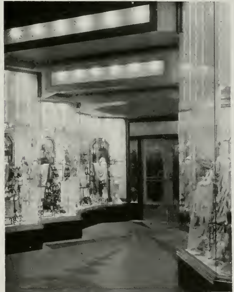
Store front modernized with sandblasted glass entrance doors, transoms, side lights, valances, and mirrors. Valances and transom lights are further decorated with transparent colors.
