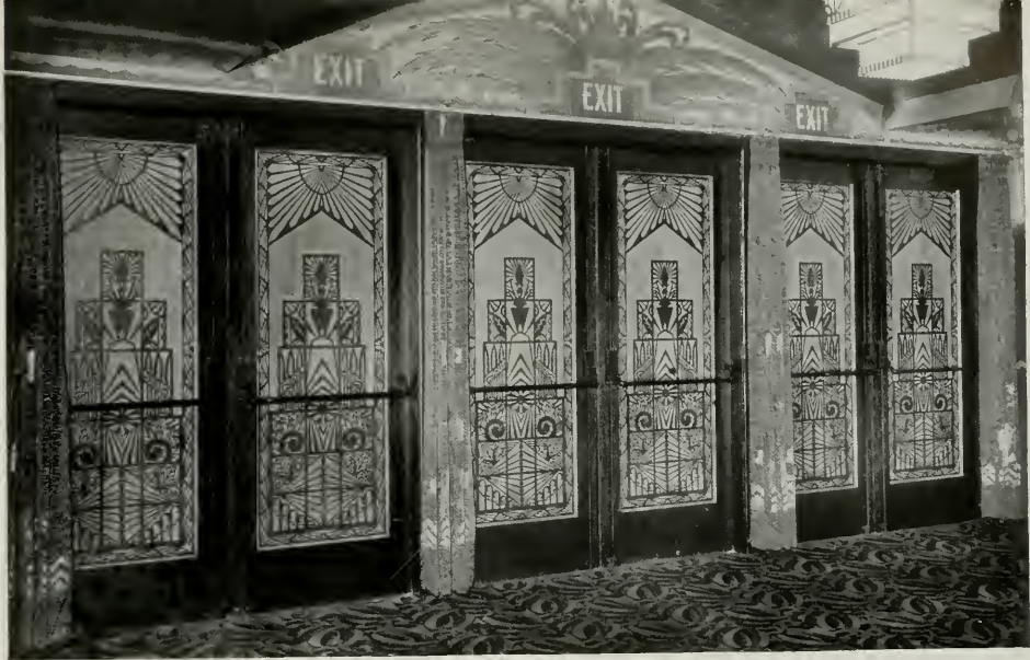
THEATER LOBBY DOORS, STAINED. THEN SANDBLASTED
