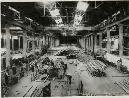
WALL PANELS BEING FABRICATED IN SHOP
