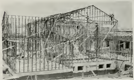
WALL FRAMING IN PLACE FOR KITCHEN
