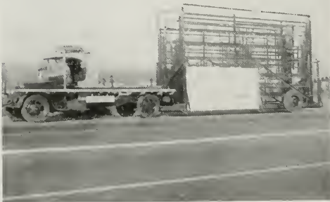
WALL PANELS BEING TRANSPORTED IN SPECIAL TRUCKS DOWN BAYSHORE HIGHWAY
