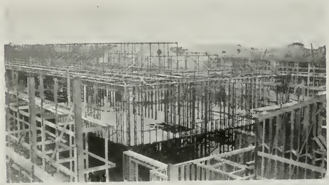
STEEL FRAME COMPLETED READY FOR ROOFING AND LATHING
