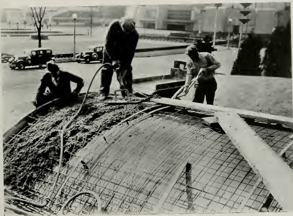
CLOSE-UP OF CONCRETE PLACING. NOTE SPREADING AND VIBRATING, ALSO BAR REINFORCEMENTS
