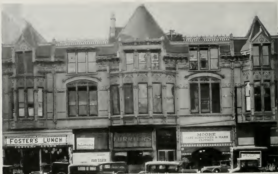
PARK BUILDING, OAKLAND, BEFORE ALTERATIONS
