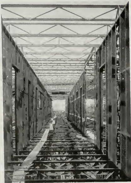
VIEW DOWN CORRIDOR, READY FOR LATHING AND FLOORING
