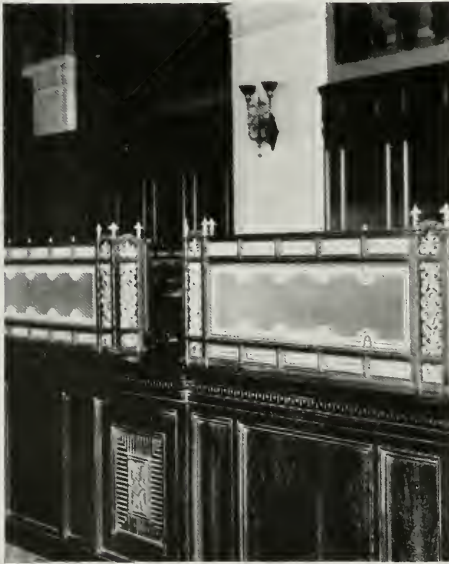
Bank counter screens of tapestry (obscure) plate glass, sandblasted with one deep cut.
