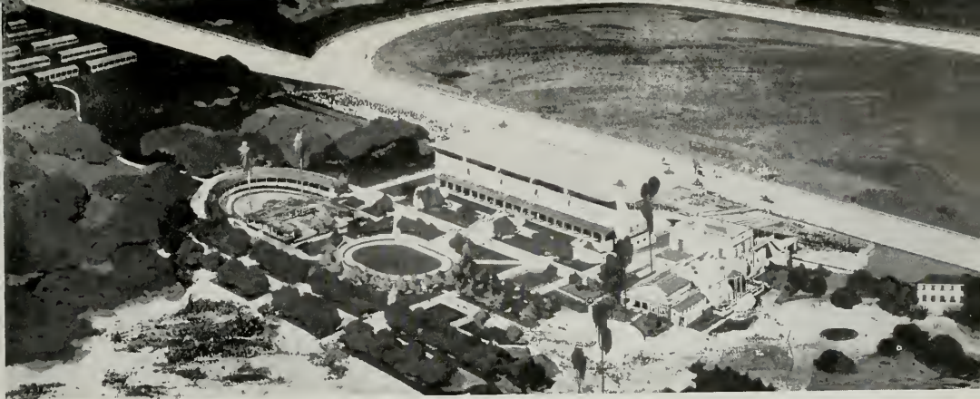
Perspective of racing plant for Los Angeles Turf Club at Santa Anita Park, Arcadia. Administration building shown at extreme right with clubhouse and grandstand along the home stretch. Open air paddock is directly back of stand with saddling stalls arranged in a semi-circle on the left. Stables at extreme left.
