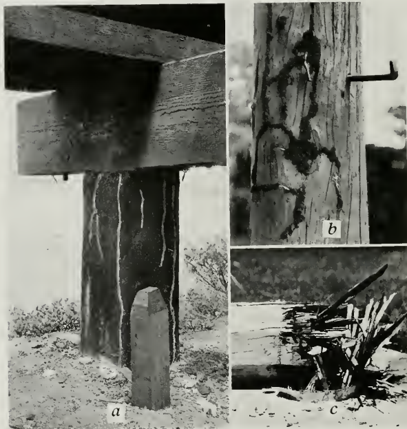
Fig. 29—Covered runways from nest in ground over concrete pile to bridge and rail timbers above. b—Earthen runways on poles. c—Flagpole in school yard set in copper-lined concrete base, which fell as result of damage by ground dwelling termites. Flag poles should be butt treated with a creosote material which protects against termites and fungi but in no way interferes with the color painting of the pole. On December 11th, 1933, a similar flag pole crashed onto the street in Presidio Terrace, San Francisco, during a wind storm. Untreated poles placed in the ground are a constant menace to life and property.
