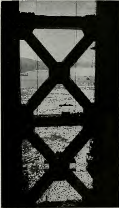
PORTALS OF THE FUTURE. MARIN TOWER, GOLDEN GATE BRIDGE
