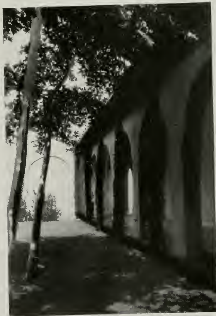
ARCADE, GEORGE S. STONEMAN SCHOOL, SAN MARINO Marsh, Smith and Powell, Architects
