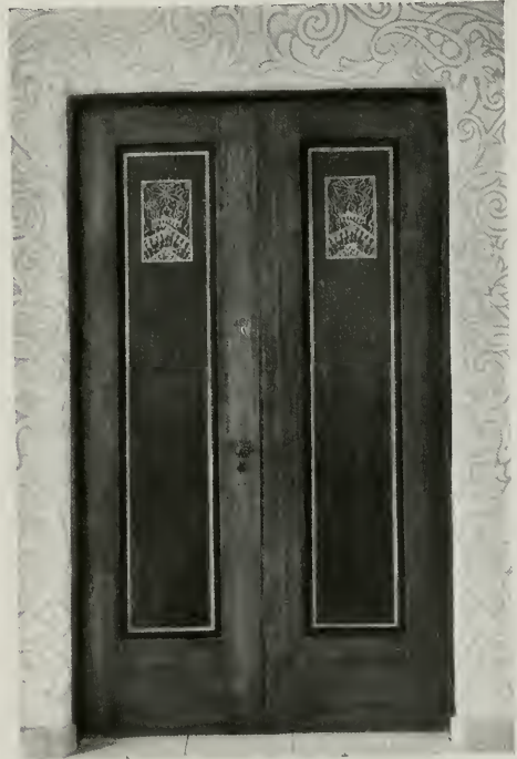
Philippine mahogany doors in private dwelling. Light portion is original surface of door. Panels are shellacked, covered with compound and sandblasted. Background stained, leaving design in light relief.
