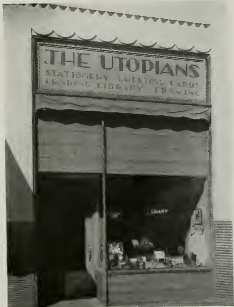
DETAIL OF SMALL SHOP, REMODELED STORE BUILDING, HOLLYWOOD, CALIFORNIA H. Roy Kelley, Architect
