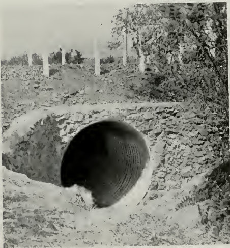
A FULL-ROUND, 105-INCH DIAMETER DRAINAGE Way made of heavy corrugated plates bolted together in the field. The rubble headwall of native stone presents a pleasing appearance.
