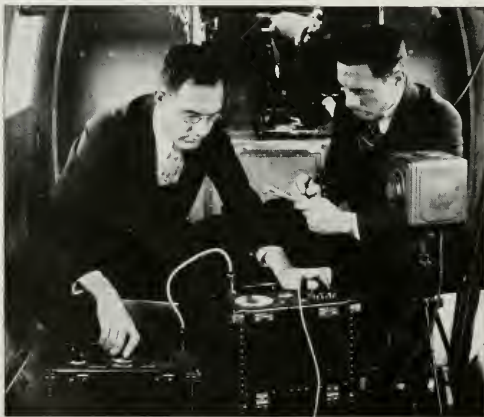
How noise is analyzed during the flight of airplanes. W. O. Osbon, engineer at the left, is conducting a noise analysis on the GA-43, new high speed air liner of the General Aviation Corporation.
