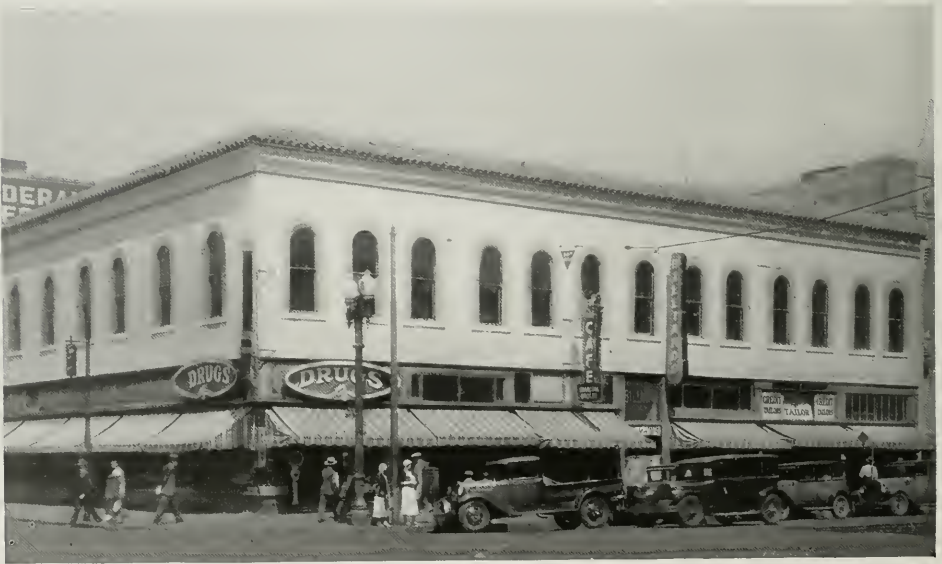
JONAS BUILDING, OAKLAND, CALIFORNIA, AFTER ALTERATIONS Edward T. Foulkes, Architect
