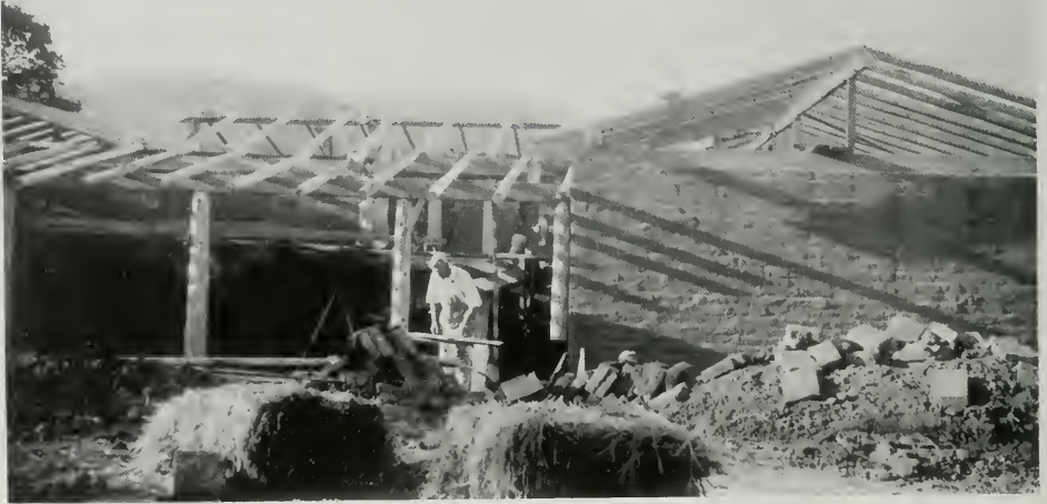
PROGRESS PICTURE, ADOBE HOUSE FOR HARRY HINDMAN. Hardman & Russ, Architects
