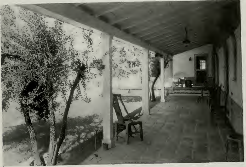
HOUSE OF MR. AND MRS. ARMSTRONG, LOS ANGELES Harold O. Sexsmith, Architect
