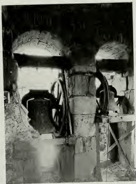
DETAIL OF BELL TOWER. San Carlos Presidio Church, Monterey
