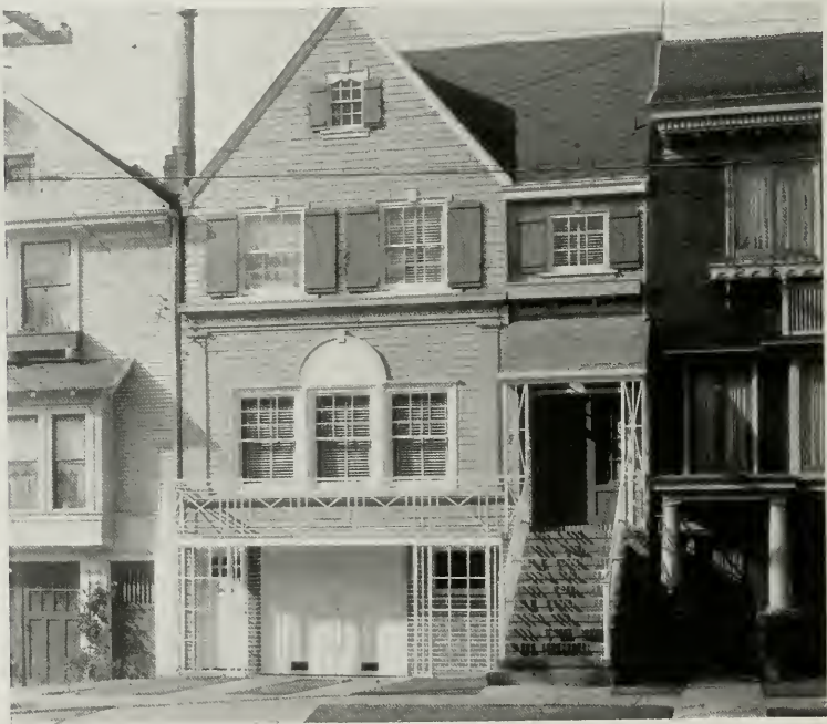
ABOVE—HOUSE AT 69 5TH AVENUE, SAN FRANCISCO, BEFORE ALTERATIONS
