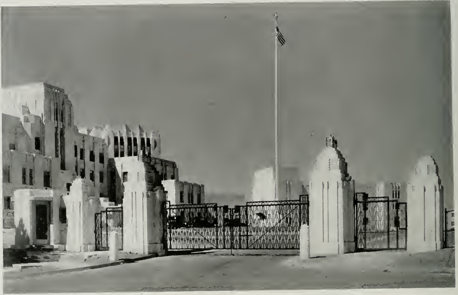
ENTRANCE TO VETERANS ADMINISTRATION FACILITY, FORT MILEY, SAN FRANCISCO
