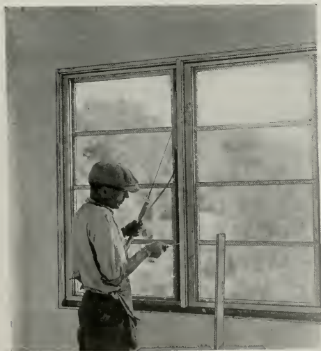
Sash come glazed and installed in frame, ready for quick, one-man installation after plastering has been completed.
