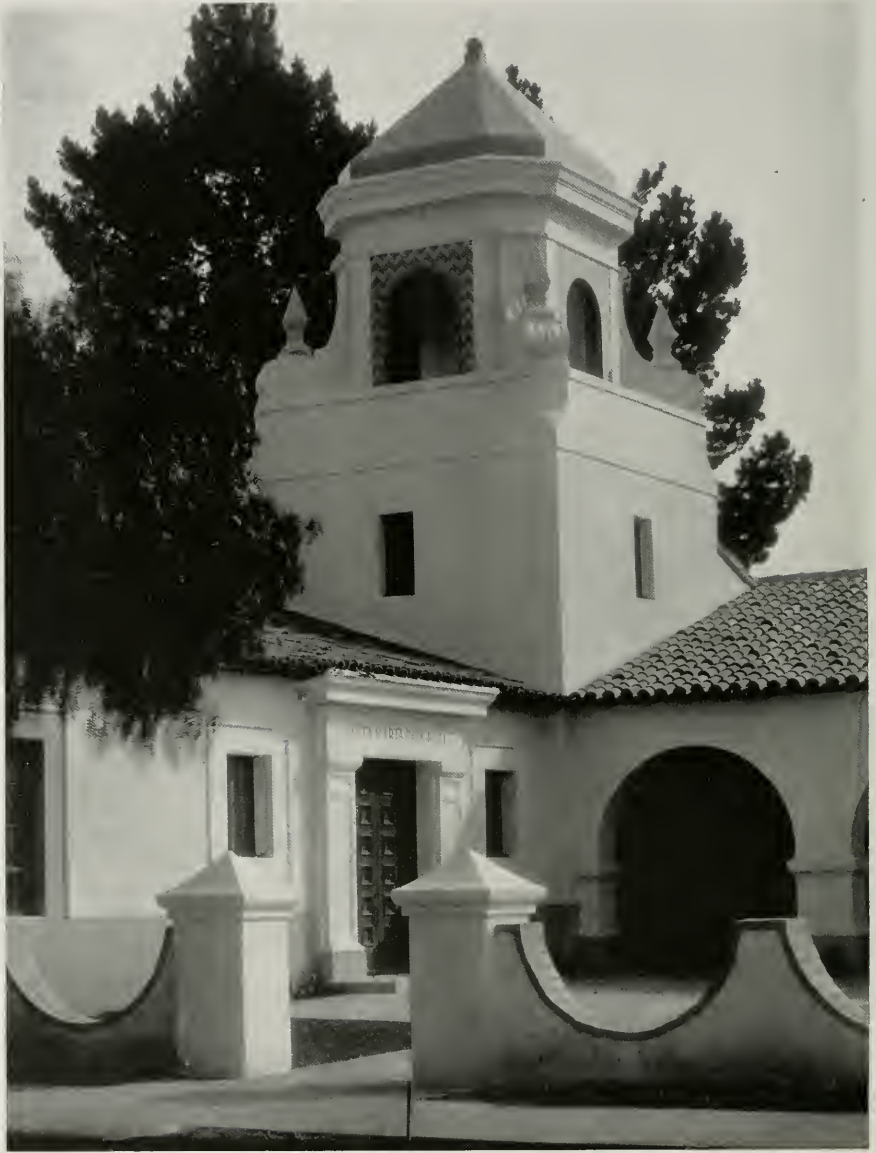
THE TOWER. CITY HALL, SANTA ROSA, CALIFORNIA LOUIS N. CRAWFORD, ARCHITECT
