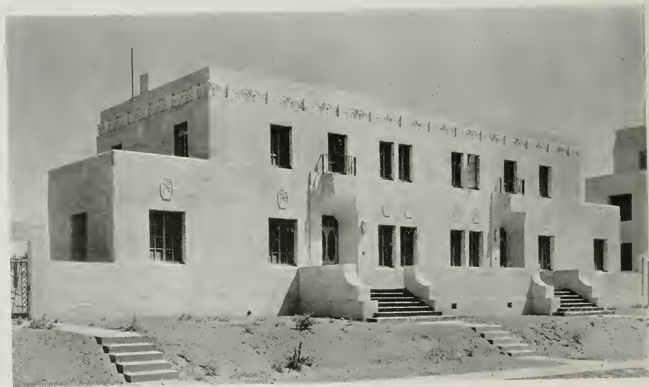
NURSES' QUARTERS, VETERANS ADMINISTRATION FACILITY, FORT MILEY, SAN FRANCISCO
