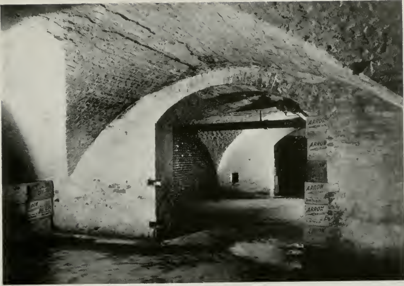
ALTHOUGH NEARLY 200 YEARS OLD, THESE VAULTS IN GLOBE BREWERY, BALTIMORE, ARE STILL IN SPLENDID CONDITION
