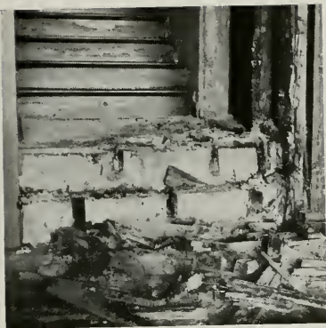
Fig. 1—There was no visible evidence of the presence of termites until the floor in the foreground was punctured by a high heel.
