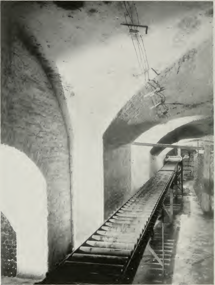
THESE WELL PRESERVED VAULTS IN THE GLOBE BREWERY, BALTIMORE, WERE BUILT IN 1744 OF BRICK BROUGHT HERE FROM ENGLAND. ENGINEERS TODAY HAVE PRONOUNCED THEM MODELS OF CONSTRUCTION
