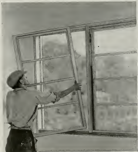
Carpenter attaches metal frame to simple wood sub-frame using ordinary wood-screws. Removable strip makes weights easily accessible.
