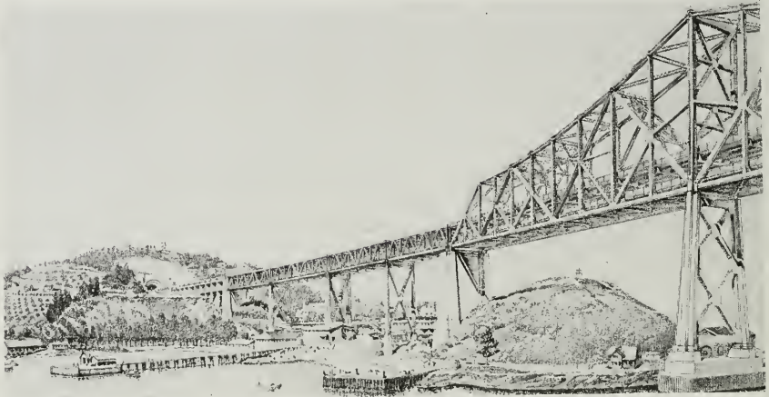
BAY BRIDGE, ENTERING YERBA BUENA ISLAND, AS SEEN FROM THE EAST SIDE
