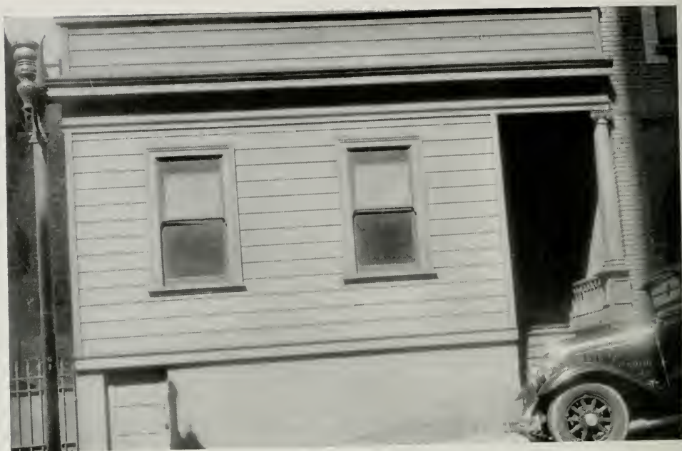
HOUSE AT 611 JONES STREET, SAN FRANCISCO, BEFORE ALTERATIONS
