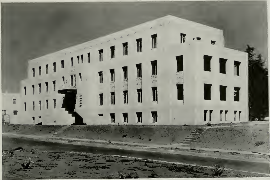
NURSES' QUARTERS, VETERANS ADMINISTRATION FACILITY FORT MILEY, SAN FRANCISCO
