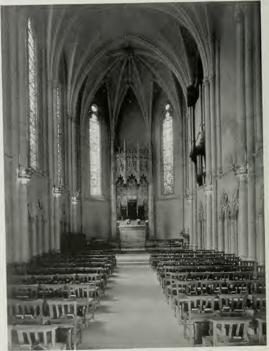
GRACE CHAPEL, GRACE CATHEDRAL, SAN FRANCISCO LEWIS P. HOBART, ARCHITECT
