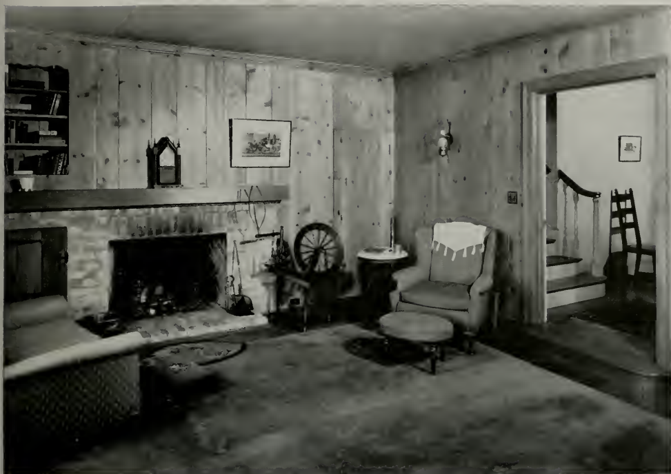
LIVING ROOM, RESIDENCE OF DR. AND MRS. H. H. ANDERSON, SAN FRANCISCO F. Frederic Amandes, Architect
