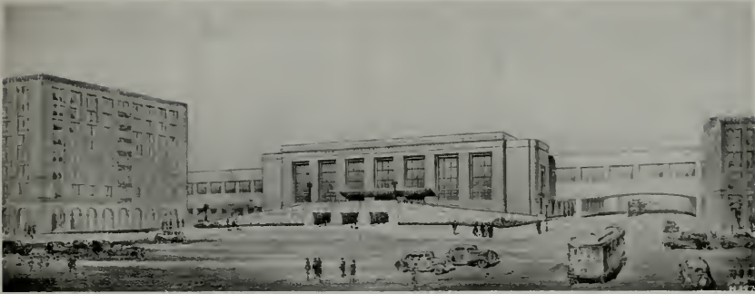
FRONT OF SAN FRANCISCO TERMINAL, showing elevated ramp for three tracks of street cars. The building provides a waiting room 135 feet wide by 220 feet long
