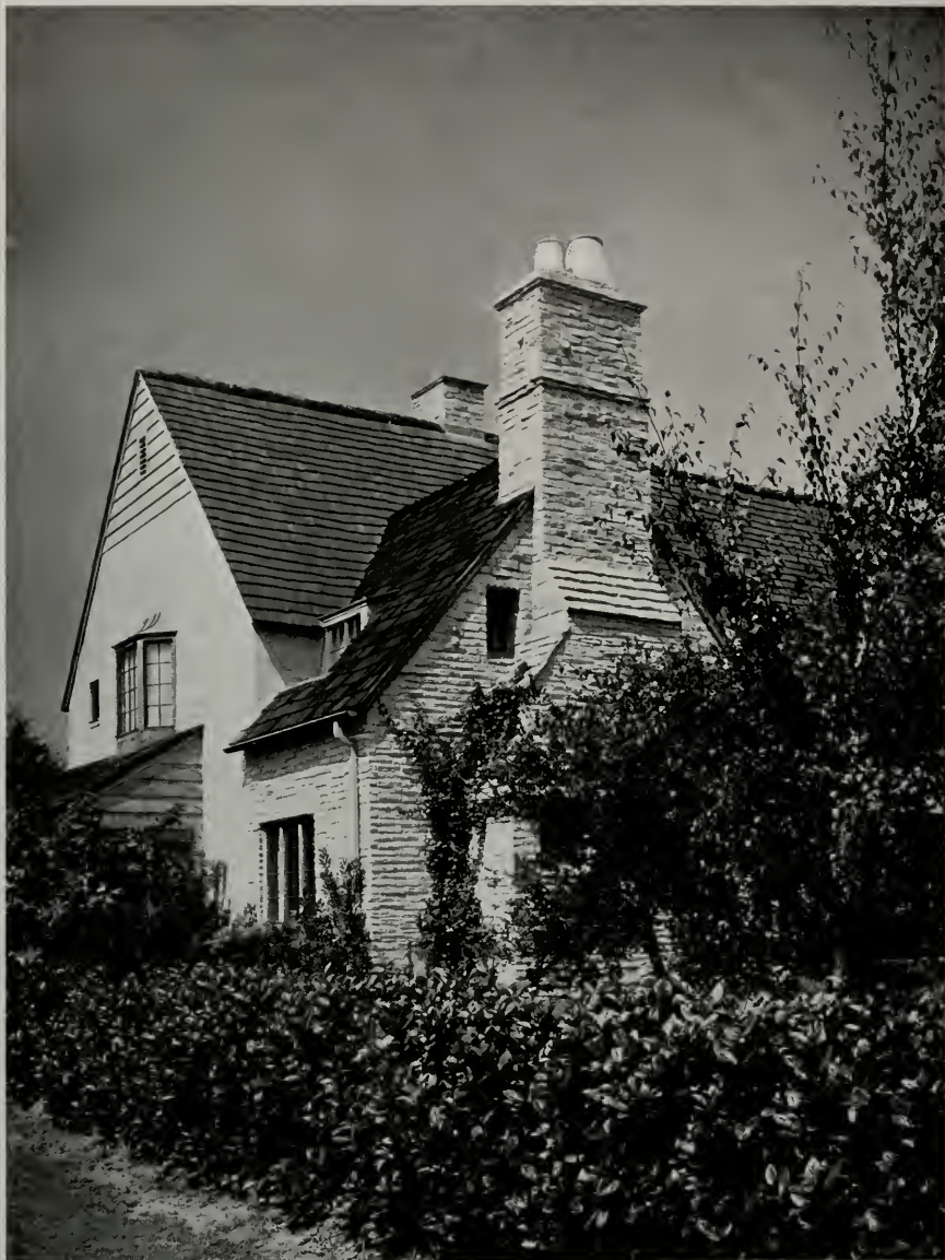
CHIMNEY DETAIL, RESIDENCE OF THEODORE OFF, HOMBLY HILLS H. ROY KELLEY, ARCHITECT
