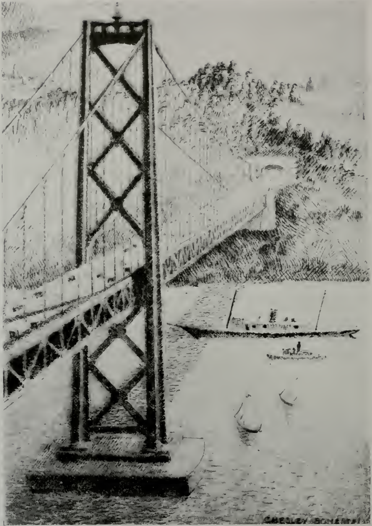
EASTERLY TOWER OF SUSPENSION SECTION OF SAN FRANCISCO BAY BRIDGE, 1110 FEET WEST OF YERBA BUENA ISLAND, SHOWING ENTRANCE TO TUNNEL.
