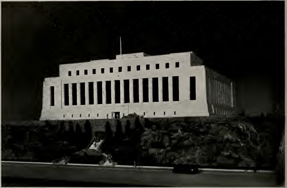
UNITED STATES MINT, SAN FRANCISCO, OFFICE OF SUPERVISING ARCHITECT GILBERT S. UNDERWOOD, ARCHITECT
