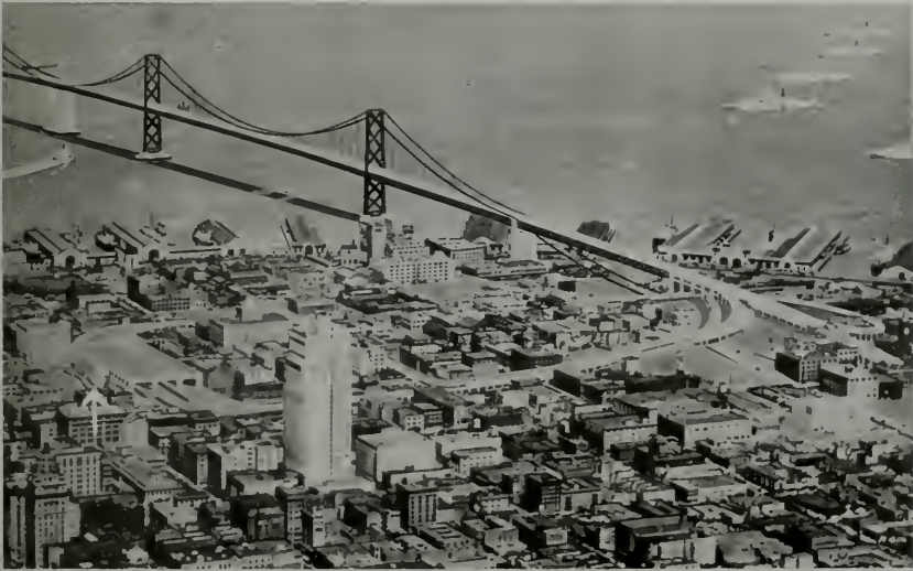
SAN FRANCISCO TERMINAL of Bay Bridge as it will appear when completed is indicated by white arrow. The building will accommodate six tracks of the interurban railway loop Illustrations Courtesy California Highways and Public Works
