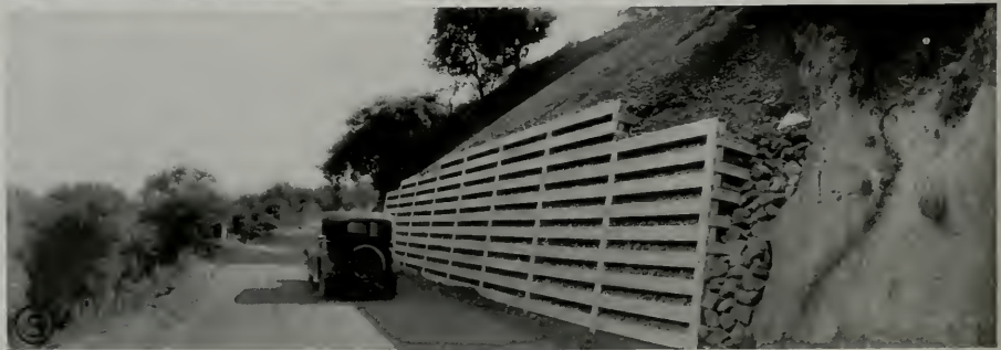
METAL CRIBBING PROVIDES EXCELLENT RETAINING WALL FOR COUNTY HIGHWAY NEAR MORAGA, CALIFORNIA 1—Preliminary excavation for the wall. 2—Placing the first course of cribbing units on correct line and batter. 3—Assembling or erecting the cribbing courses. 4—Cribwall complete, ready for the remainder of the backfill. 5—Completed job. The roadway above at the right can be visualized.
