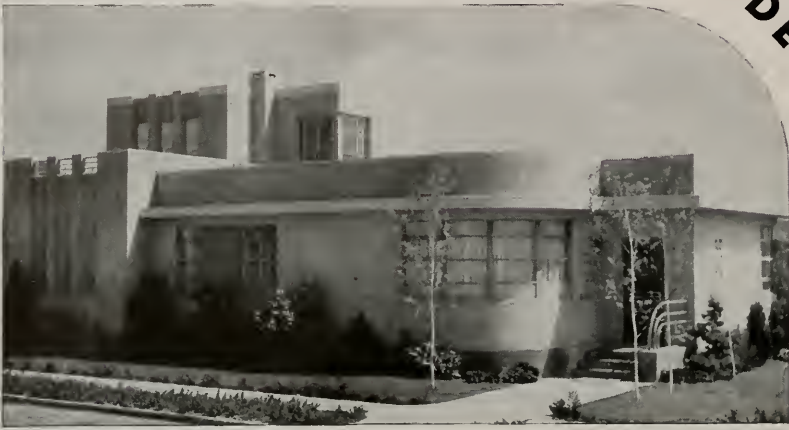
Office, Dr. S. N. Weil, Rodeo, Calif. Architects: Hertzka & Knowles San Francisco
