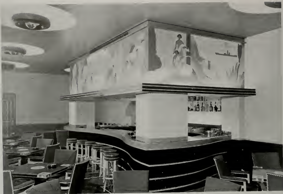
COCKTAIL LOUNGE IN HOTEL PORTAGE, AKRON, OHIO, SHOWING RUBBER MURALS, TIRE CHANDELIERS, RUBBERIZED UPHOLSTERING, ETC.
