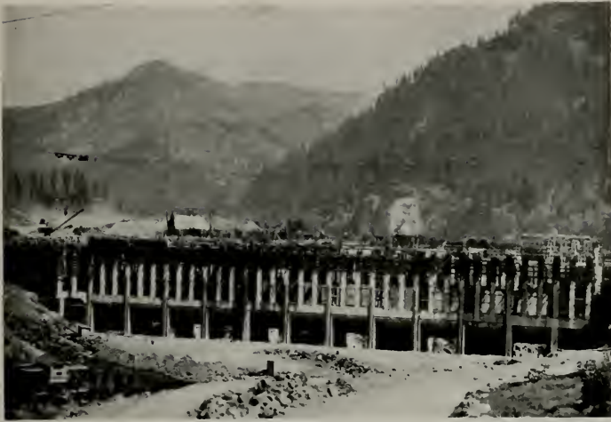
The power-house dam as seen from the downstream side. Over the roads in the foreground constantly roll Standard Oil trucks with fuel and lubricants used by the contractors. When the project is completed, these roads will be buried beneath water flowing through the power-house above the dam.
