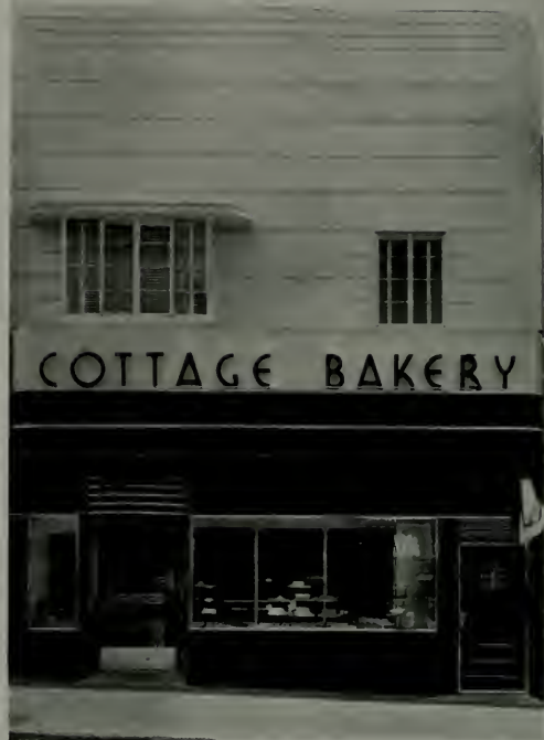
Upper picture shows Cottage Bakery in Hayward, Calif., before the architects, Miller and Warnecke, undertook to modernize the structure. Picture on the right indicates a remarkable transformation by using a dark maroon Ferro-porcelain for the first story while the upper portion is finished in plaster with painted wood strips to relieve the flat surface. The sign has a cream background with maroon letters. Stainless steel snap-on moulding was used at the top of the first story while the door leading to the bakery proper has a Ferro-porcelain panel relieved with small strips of stainless steel.
