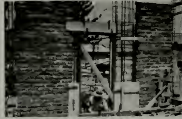
BUILDING WITH BRICK AND HOLLOW TILE IN SAN SALVADOR
