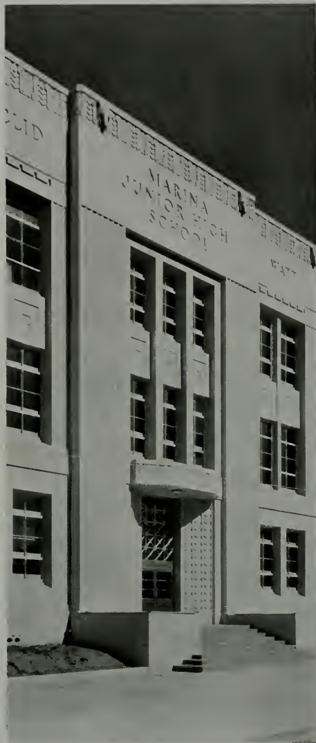
DETAIL, MARINA JUNIOR HIGH SCHOOL, SAN FRANCISCO Geo. W. Kelham and W. P. Day, Architects
