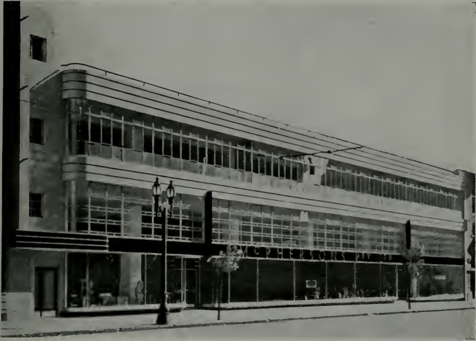
McPHERSON'S BUILDING, MELBOURNE, AUSTRALIA Reid & Pearson and Stuart P. Calder, Joint Architects
