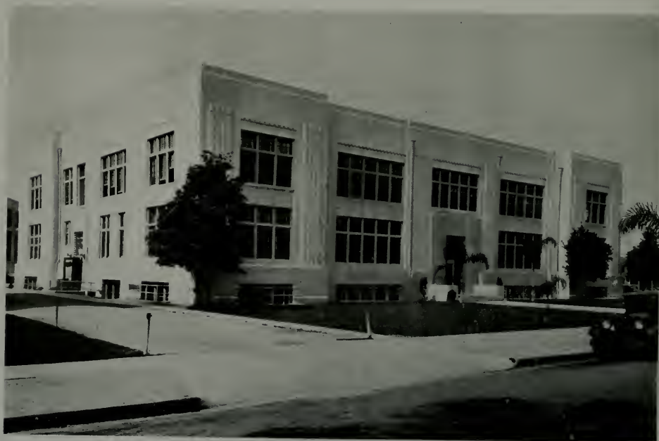
AFTER ALTERATIONS—COMPLETED 1936 FINE ARTS BUILDING, INGLEWOOD UNION HIGH SCHOOL, INGLEWOOD, CALIFORNIA T. C. Kistner, Architect
