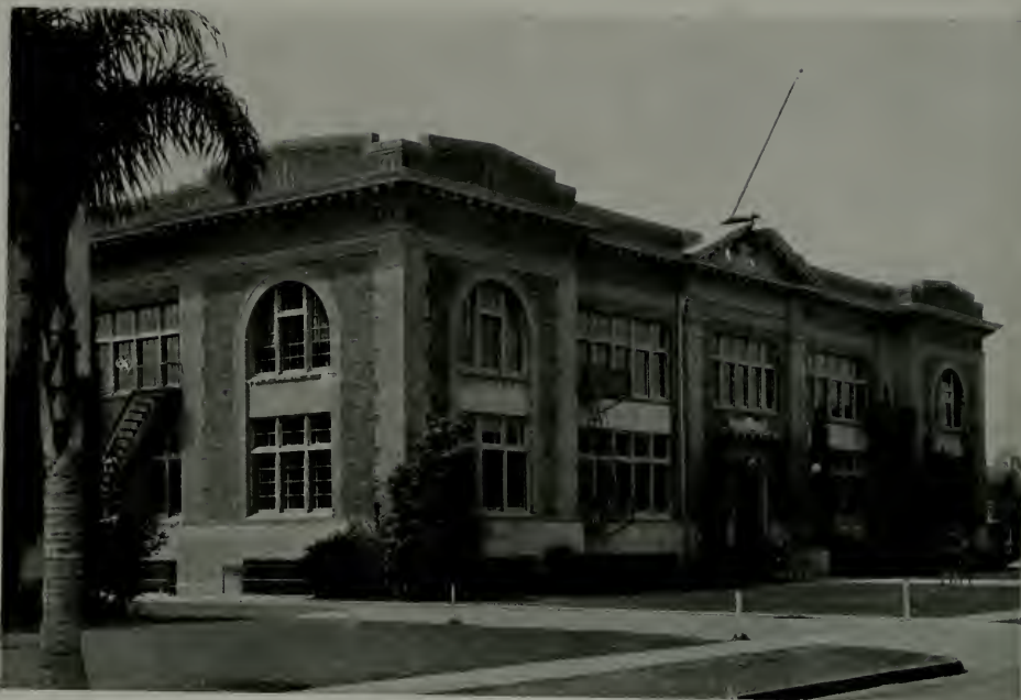
BEFORE ALTERATIONS—BUILT IN 1924 FINE ARTS BUILDING, INGLEWOOD UNION HIGH SCHOOL, INGLEWOOD, CALIFORNIA
