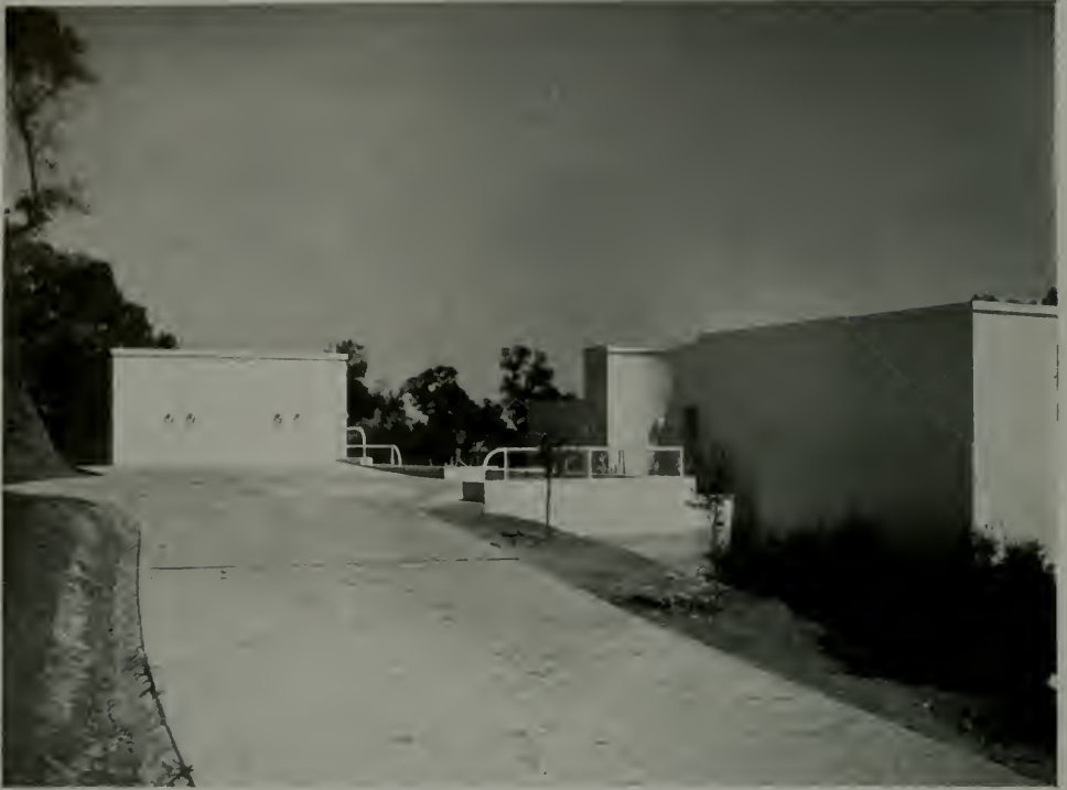
ROAD ELEVATION, RESIDENCE OF DR. AND MRS. SAXTON T. POPE, BURLINGAME, CALIFORNIA
