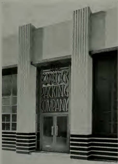
DETAIL OF ENTRANCE, BUILDING FOR GARLOCK PACKING COMPANY, SAN FRANCISCO
