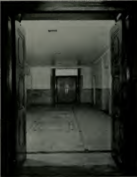
LOBBY, COURT ROOM FLOOR
