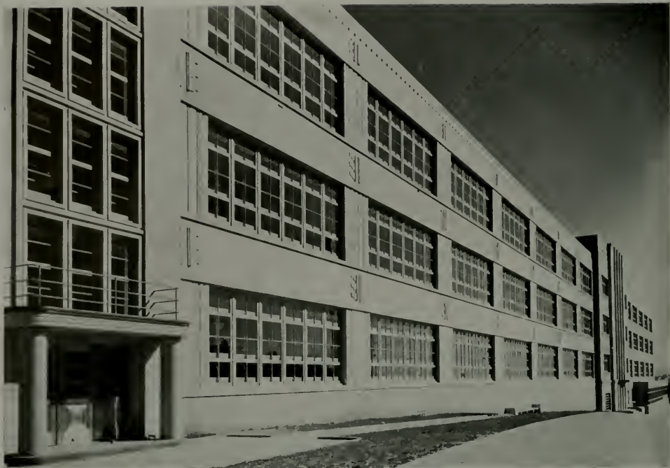
GEORGE WASHINGTON HIGH SCHOOL, SAN FRANCISCO, CALIFORNIA J. R. Miller and T. L. Pflueger, Architects View gives a splendid idea of the great length of the building—487 feet.
