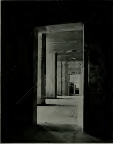
MAIN ENTRANCE LOBBY FROM SUPERVISORS' STAIRWAY
