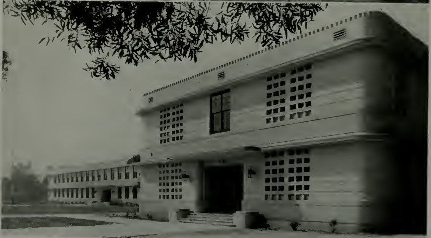
MANUAL ARTS HIGH SCHOOL GROUP, LOS ANGELES, CALIFORNIA JOHN PARKINSON AND DONALD B. PARKINSON, ARCHITECTS
