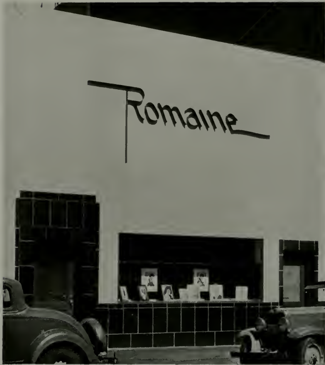
THEATRICAL PICTURE STUDIO, SAN FRANCISCO Bliss and Fairweather, Architects Exterior white and black unit tile
