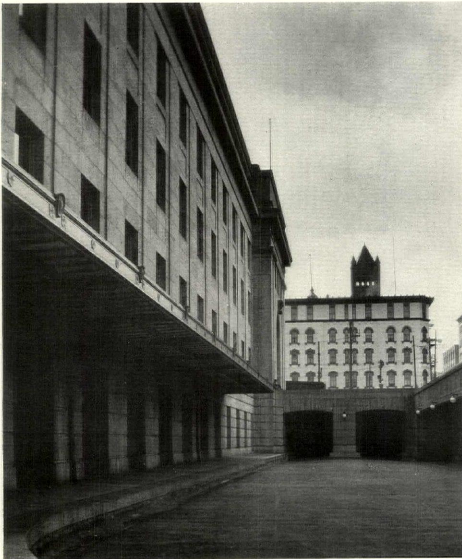
Cab Entrance, Lower Level, Looking toward Arches to Ramp
