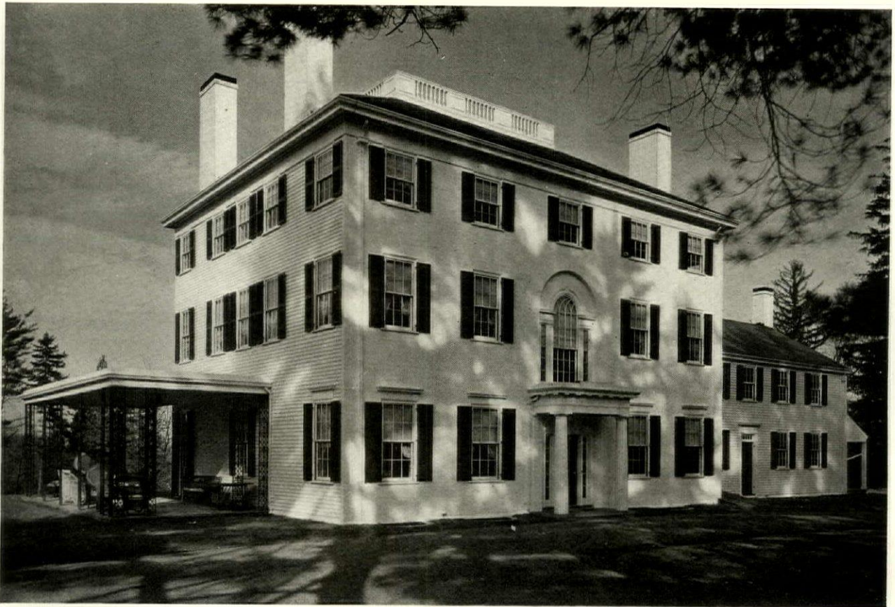
GENERAL VIEW OF ENTRANCE FRONT
