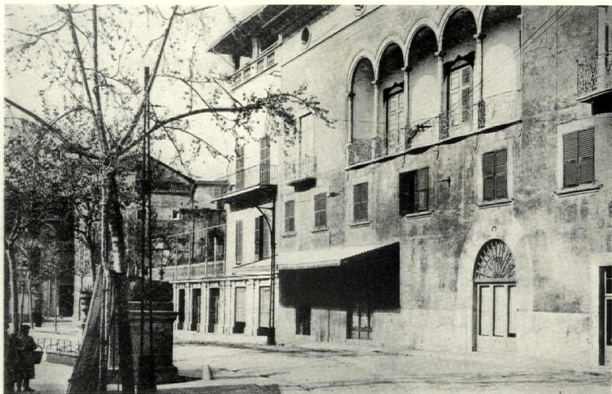
Street Facade of Casa del Marques de Sollerich, Palma, Majorca
