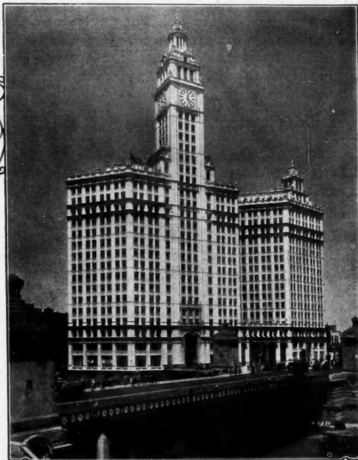
WRIGLEY BUILDING, CHICAGO, ILL.
