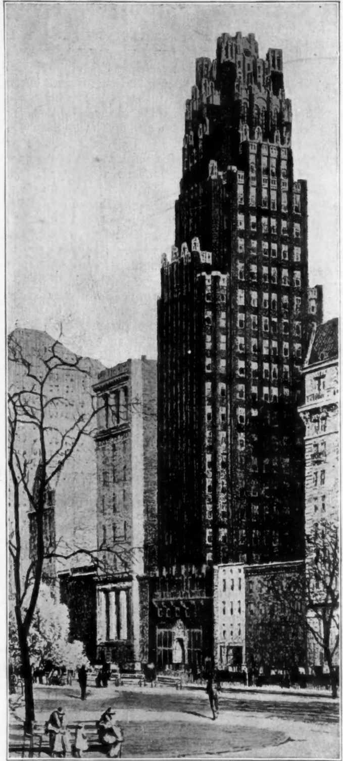
This striking new building of the American Radiator Co., on 40th Street, facing Bryant Park, New York, is completely equipped with Whale-Bone-Ite toilet seats, model 21-96, in ebony. The building is finished in black and gold, with stone facing, and has created considerable comment recently. The architect was Raymond M. Wood.
