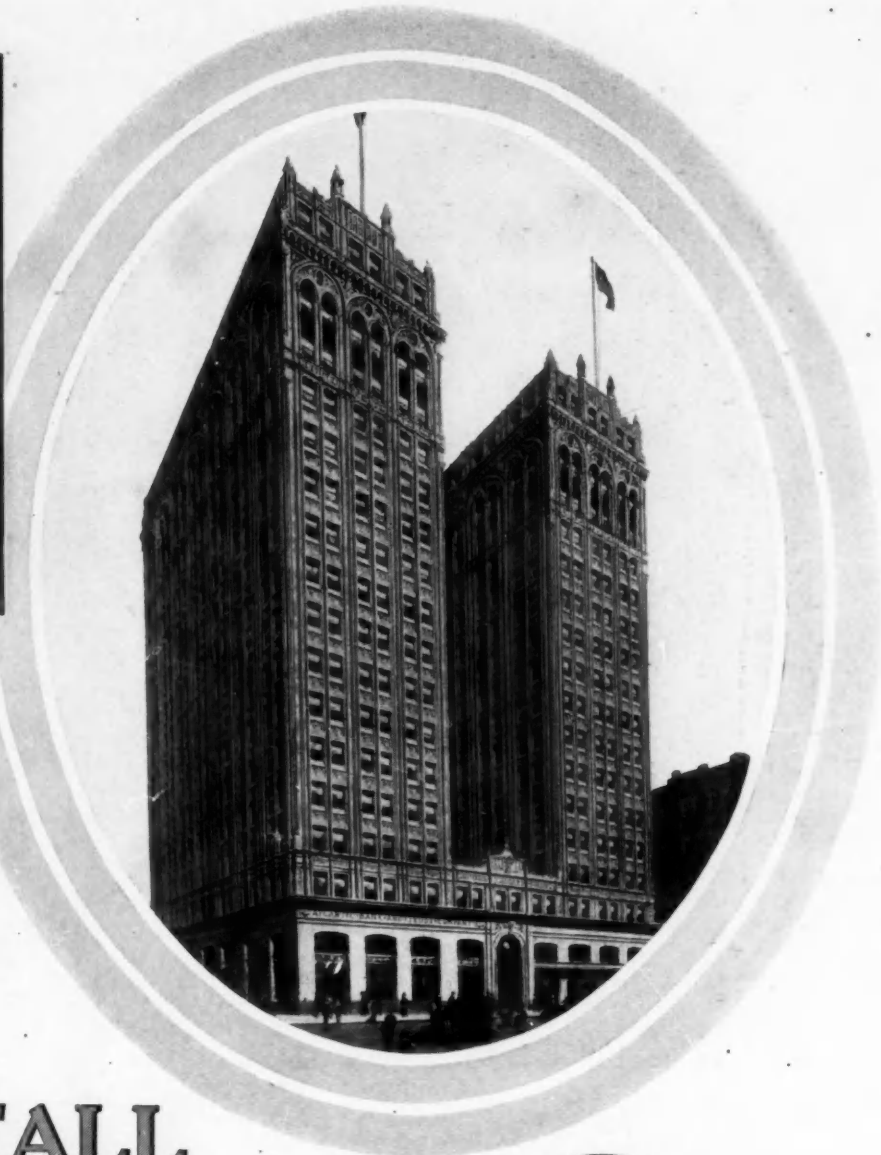
Crittall Reversible Windows are used in the Jefferson Standard Building, Greensboro, N. C., illustrated at right. Chas. C. Hartmann, Architect
