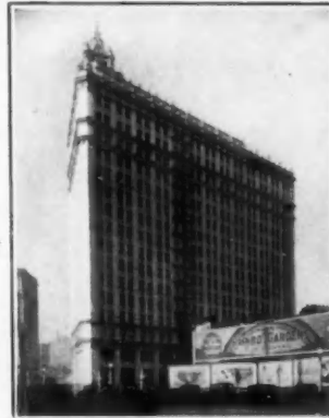
North Section of Wrigley Bldg. Chicago, Ill.
