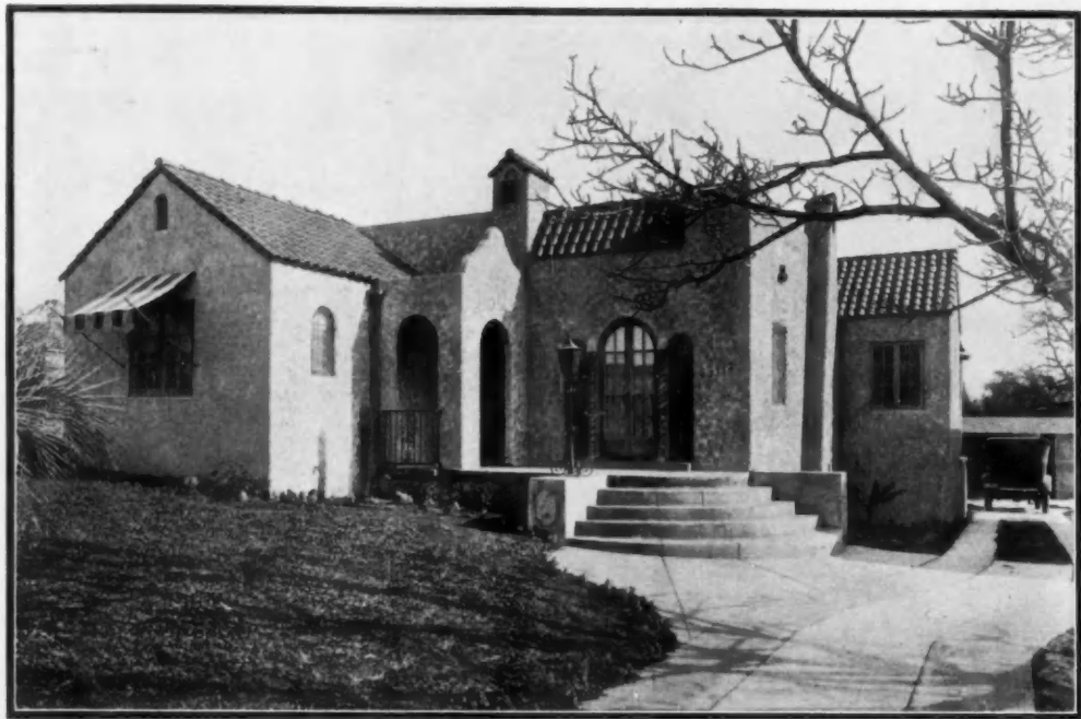
Residence of E. S. Brooks, 1112 Hacienda St., Los Angeles, Cal. Bishopric Stucco over Bishopric Base on all exteriors
