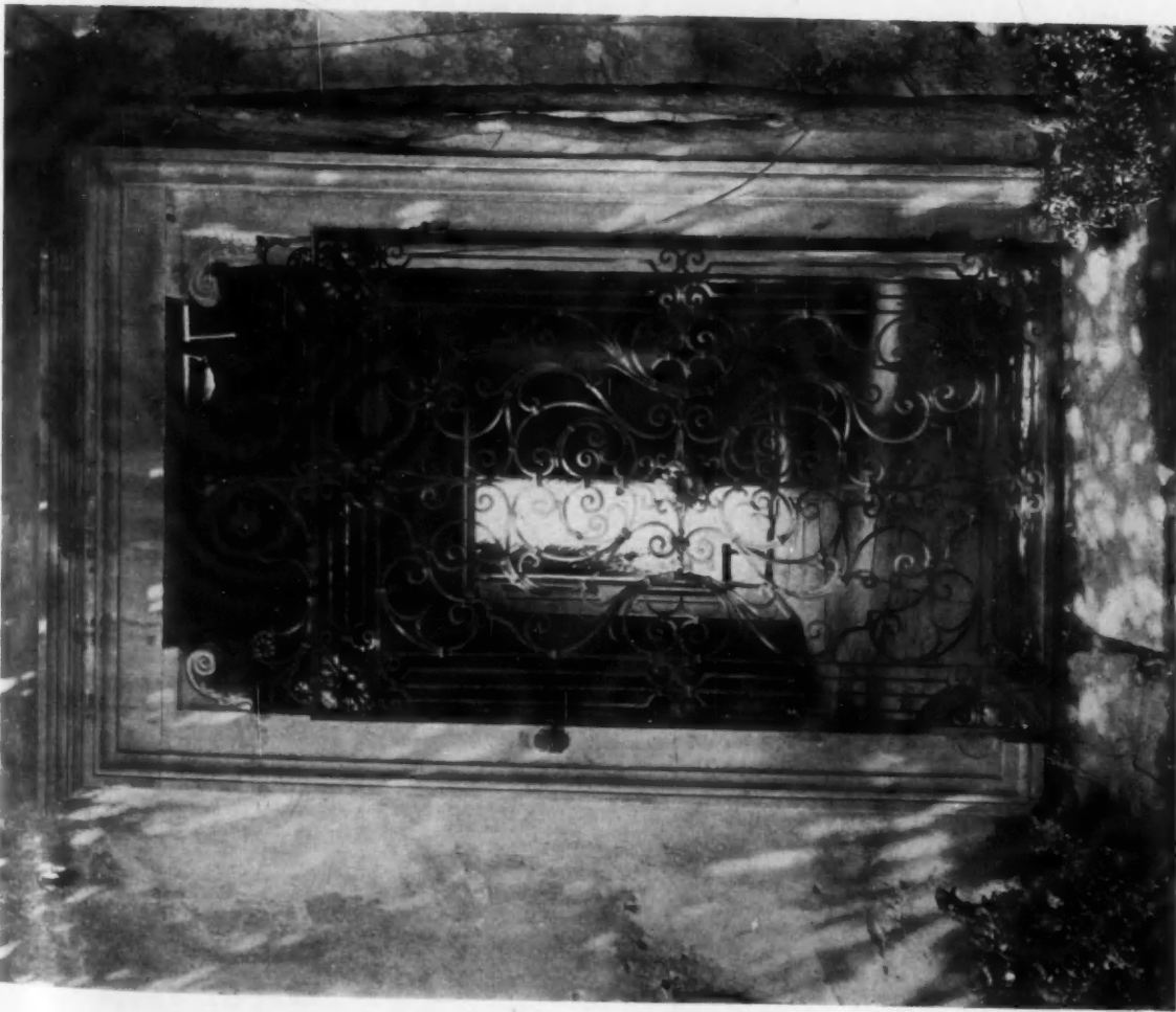
WROUGHT IRON GATE FROM THE LOGGIA INTO THE TOOL HOUSE
