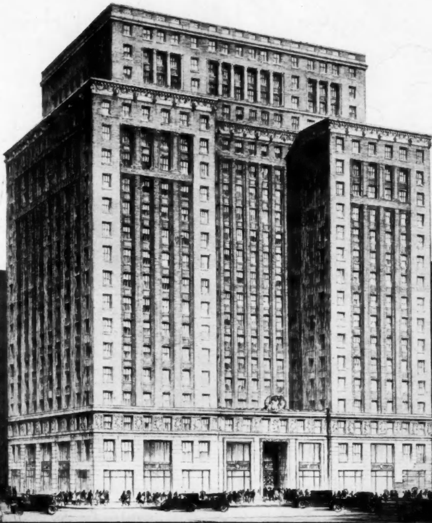
POSTUM OFFICE BUILDING 250 BAKER AVENUE NEW YORK
