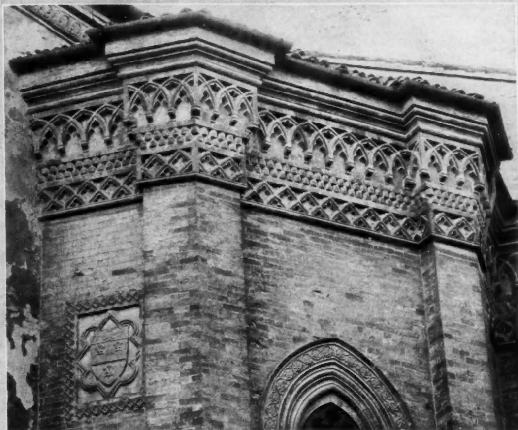
Terra Cotta Cornice of Small Chapel, Cathedral at Parma, Italy (From a revised and enlarged edition of "Color in Architecture" published by the National Terra Cotta Society)
