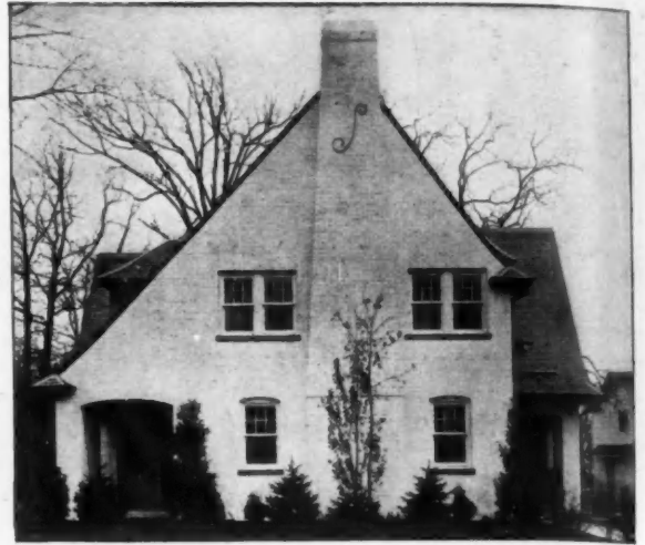
Common brick walls finished with Cabot's Old Virginia White; roof stained with Cabot's Creosote Shingle Stain, Lichen Green. F. A. Cooper, Architect, Chicago
