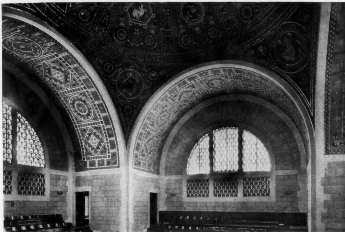
NATIONAL ACADEMY OF SCIENCE BUILDING
