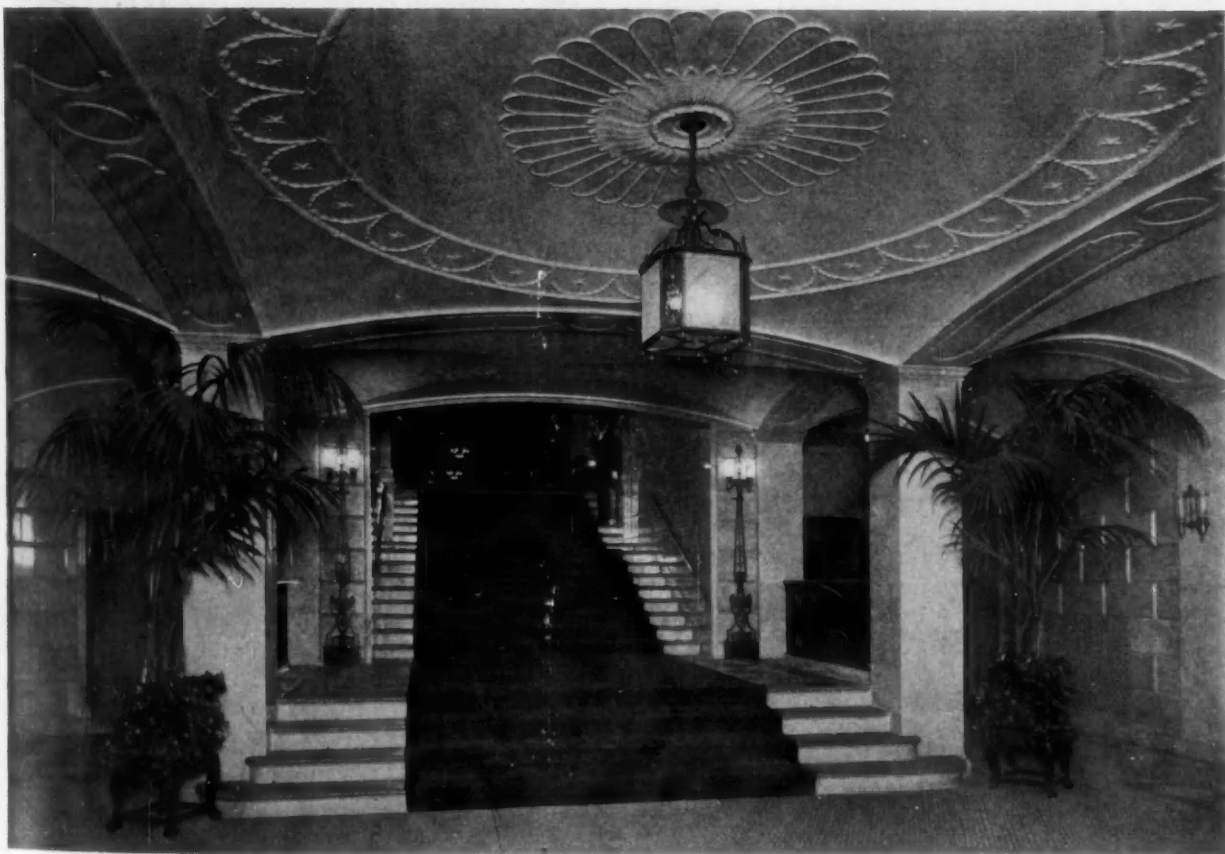
A Monumental Stairway Leads from the Entrance Vestibule to the Main Lobby
