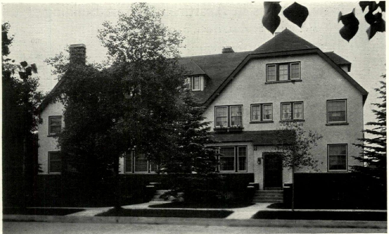
Apartment Building at Laramie, Wyo. Wilbur A. Hitchcock, Architect
