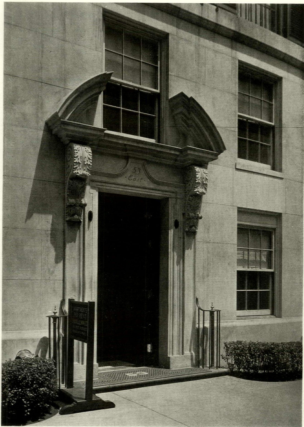
DETAIL, ENTRANCE DOOR NO. 53 EAST 66TH STREET, NEW YORK MOTT B. SCHMIDT, ARCHITECT
