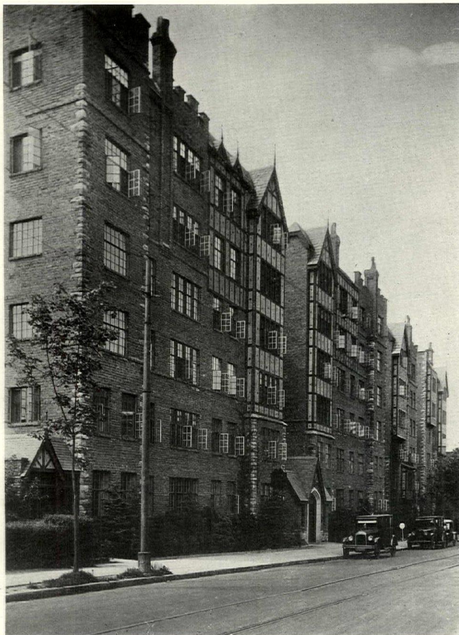
"Peldean Court" and "Pelbrook Hall," Pelham, N. Y.
