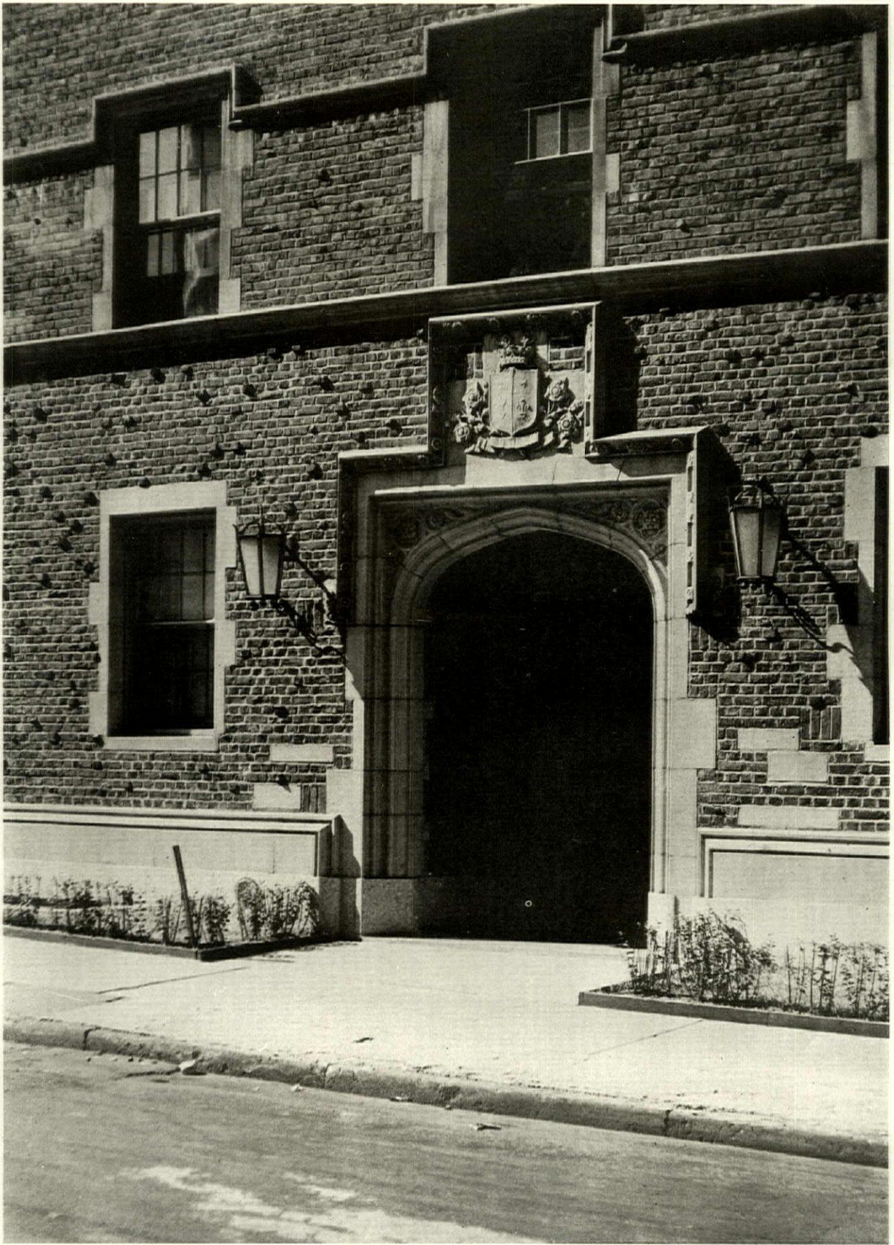
DETAIL, BROOKLYN HEIGHTS APARTMENTS, BROOKLYN DANIEL D. MERRILL, ARCHITECT
