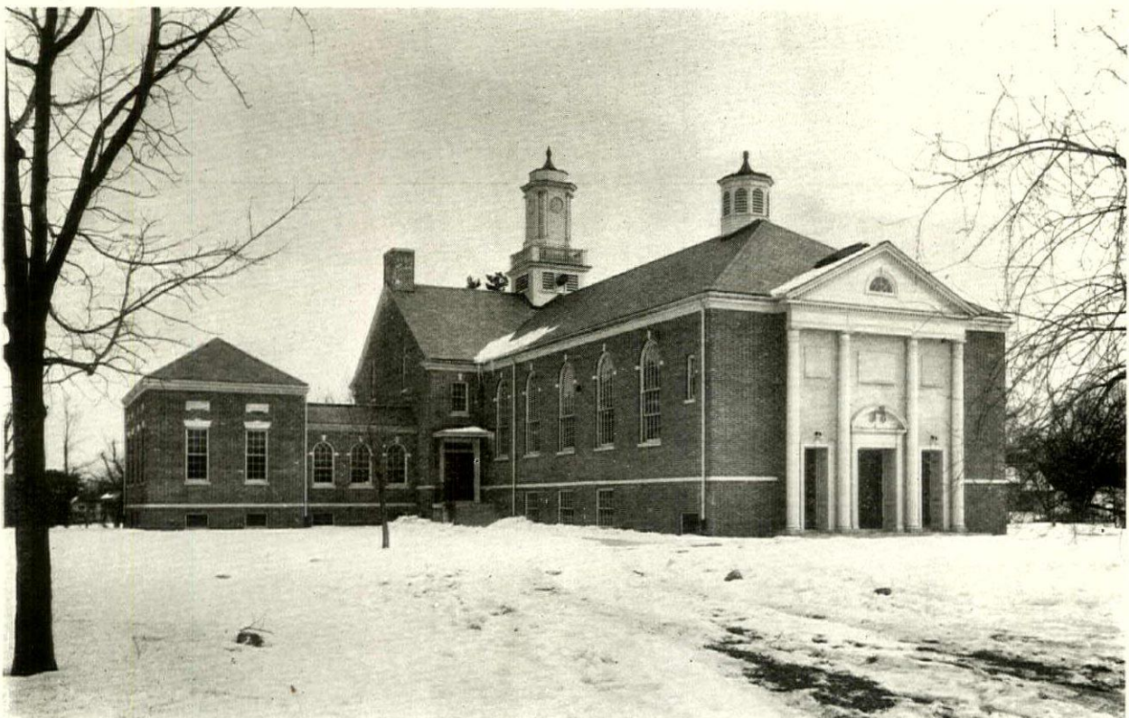
Rear View Showing the Auditorium Wing
