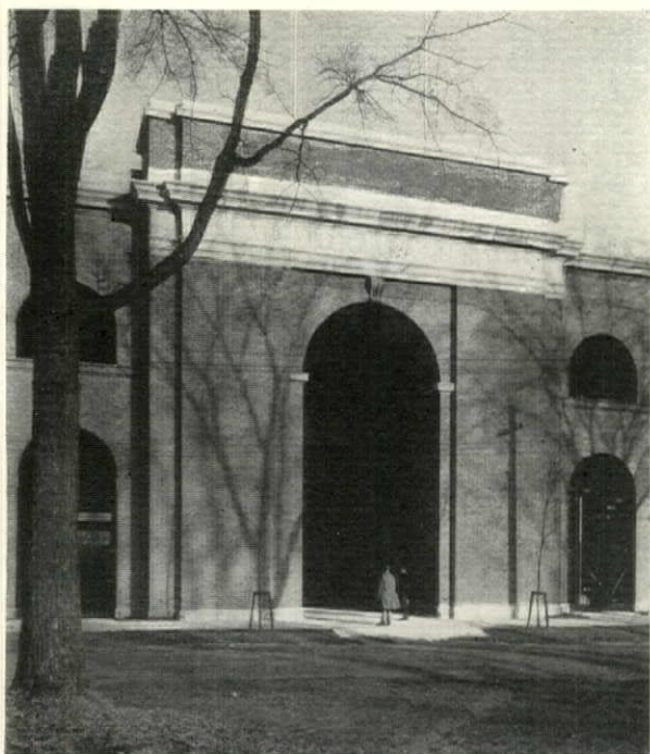
Entrance, Memorial Field, Dartmouth College, Hanover, N. H. Larson & Wells, Architects
