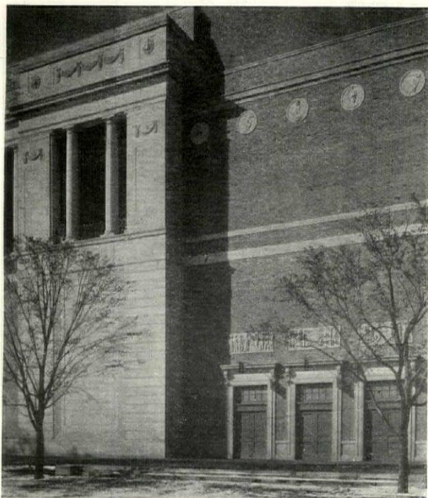
Detail, Stadium, University of Illinois Holabird & Roche, Architects
