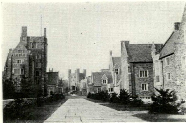
Looking Toward Blair Arch, New Dormitory Group, Princeton University
