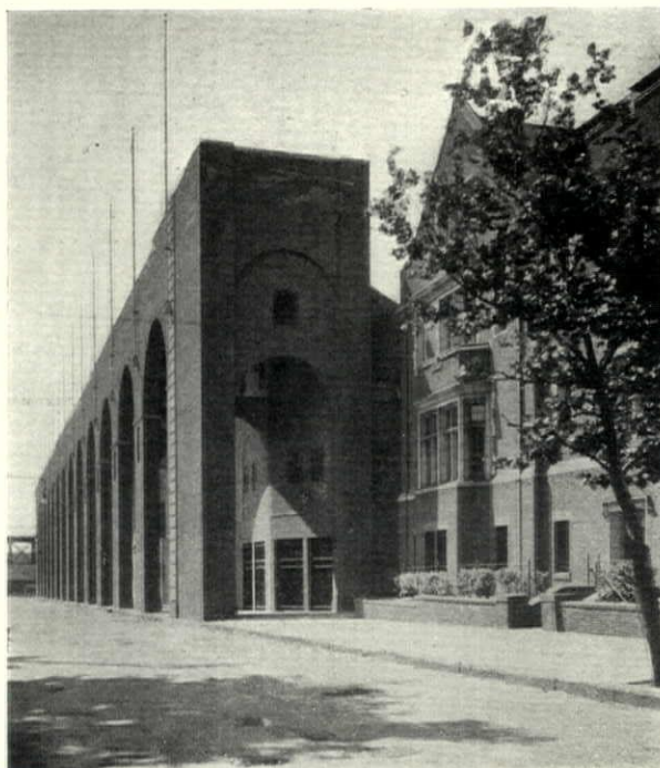
Detail, Franklin Field Stadium, University of Pennsylvania, Philadelphia Day & Klauder, Architects
