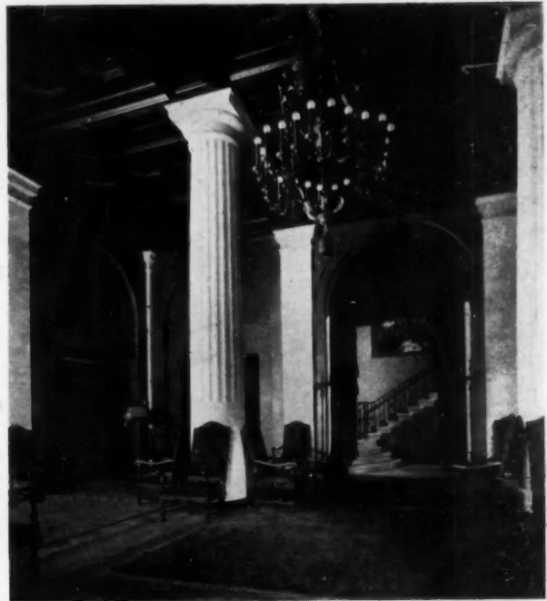
Detail, Lobby, Buffalo Athletic Club Edward B. Green & Sons, Architects
