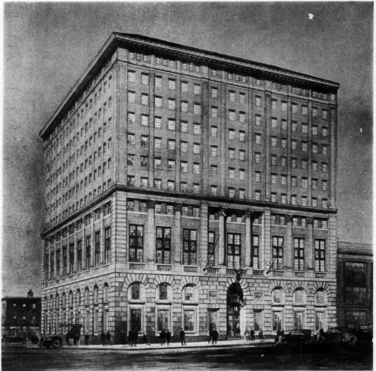
Perspective, New Building for Elks' Lodge No. 22, Brooklyn McKim, Mead & White, Architects
