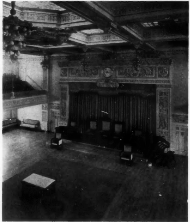
Lodge Room, Elks' Club, Elmhurst, N. Y. The Ballinger Co., Architects
