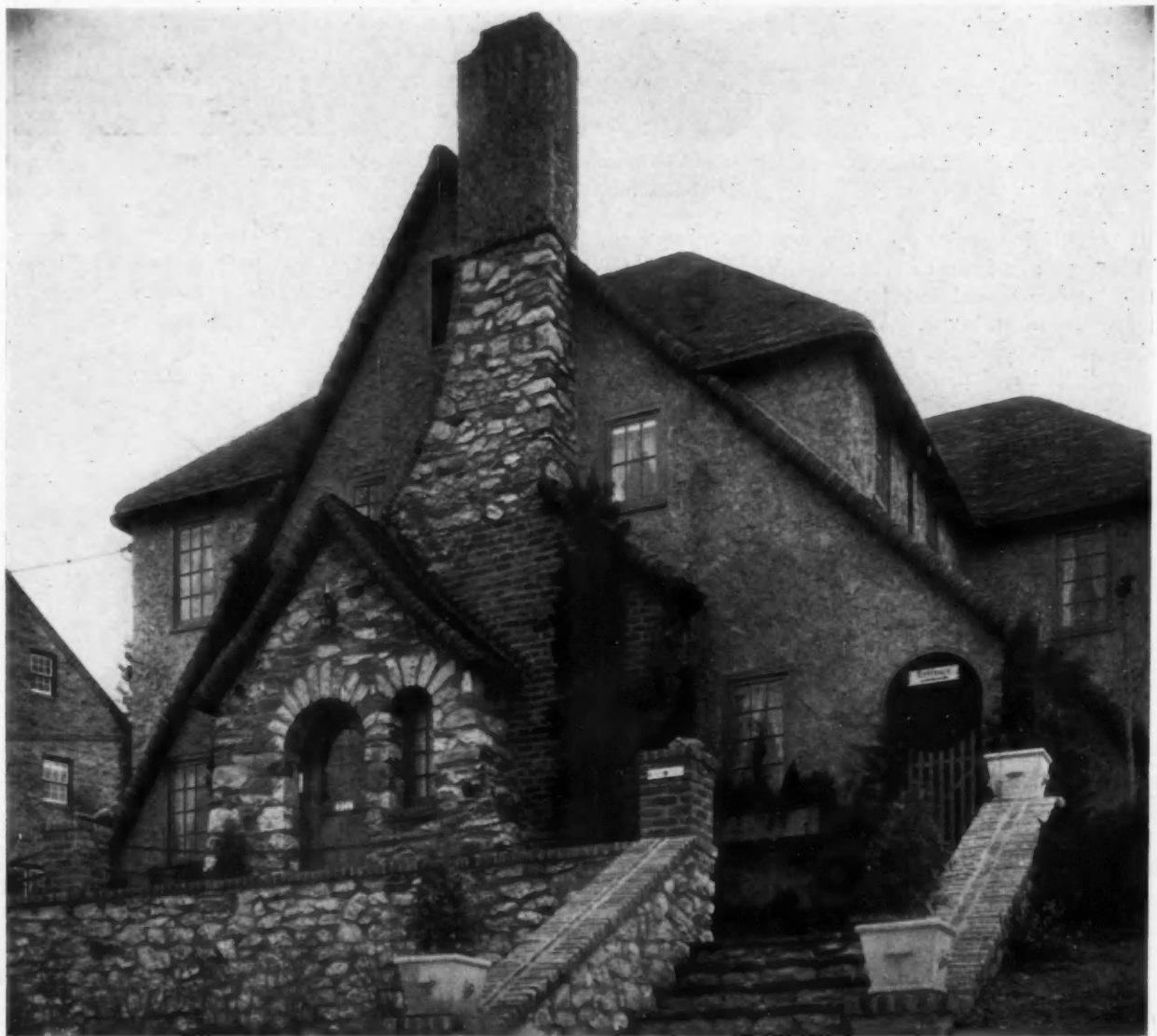
Office and House of Thomas J. Good, Pelham Manor, N. Y. Arthur Purdy, Architect
