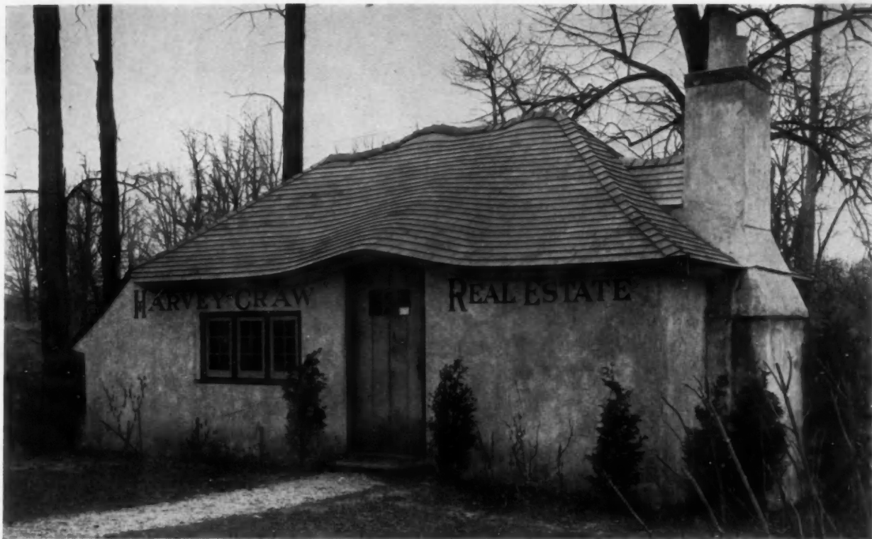
REAL ESTATE OFFICE AT GREAT NECK, N. Y. FRANK J. FORSTER, ARCHITECT
