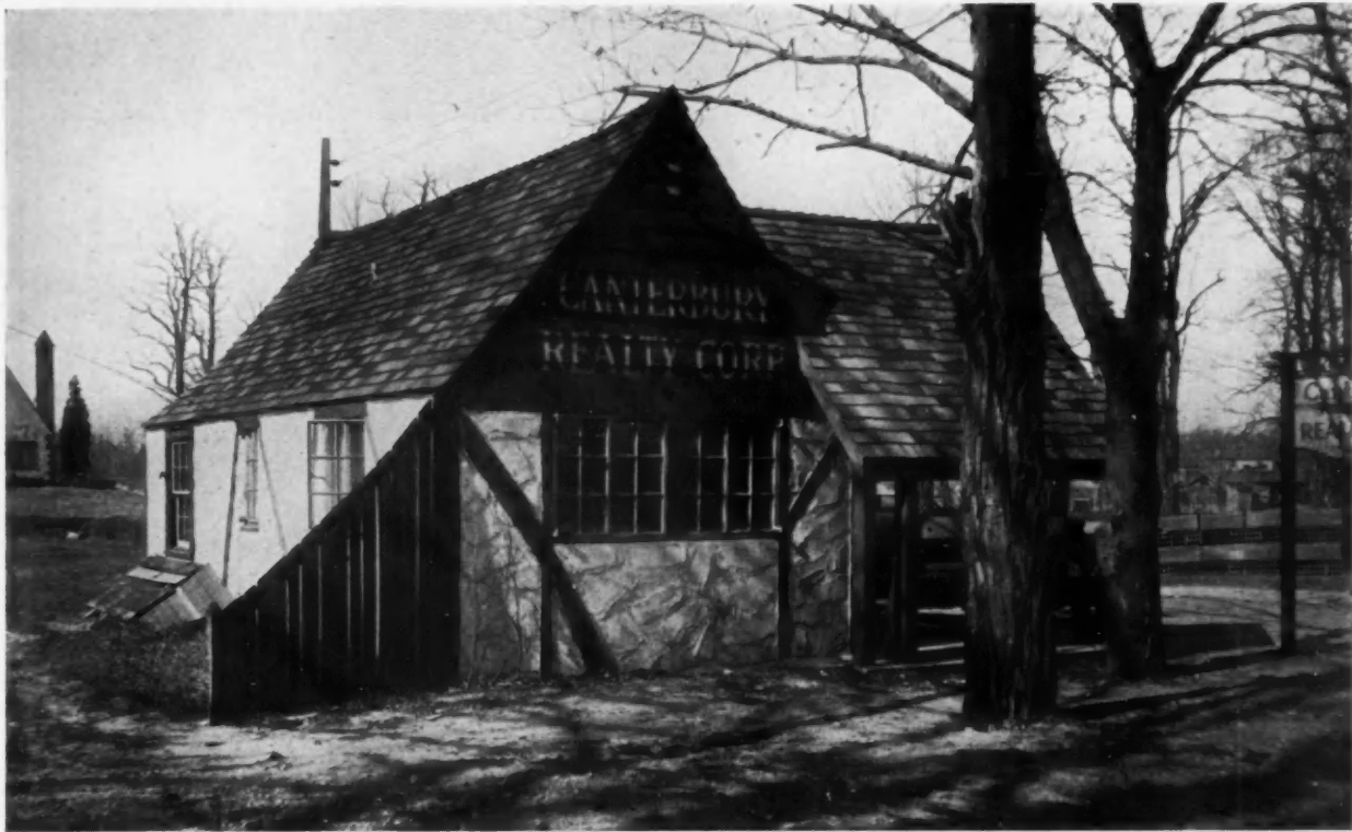
BUILDING FOR CANTERBURY REALTY CORPORATION, GREAT NECK, N. Y. JAMES MACPHERSON, ARCHITECT
