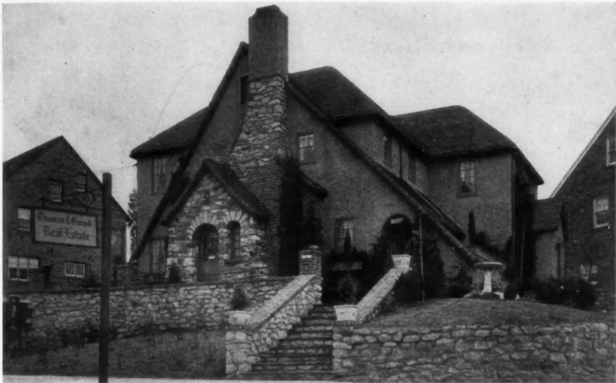
OFFICE AND HOUSE OF THOMAS J. GOOD, PELHAM MANOR, N. Y. ARTHUR PURDY, ARCHITECT
