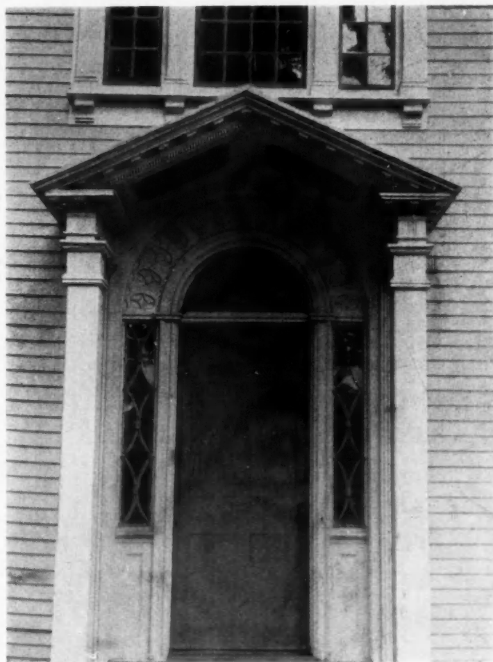
ENTRANCE PORCH, THE WHEELER-BEECHER HOUSE, BETHANY, CONN.; BUILT IN 1805
