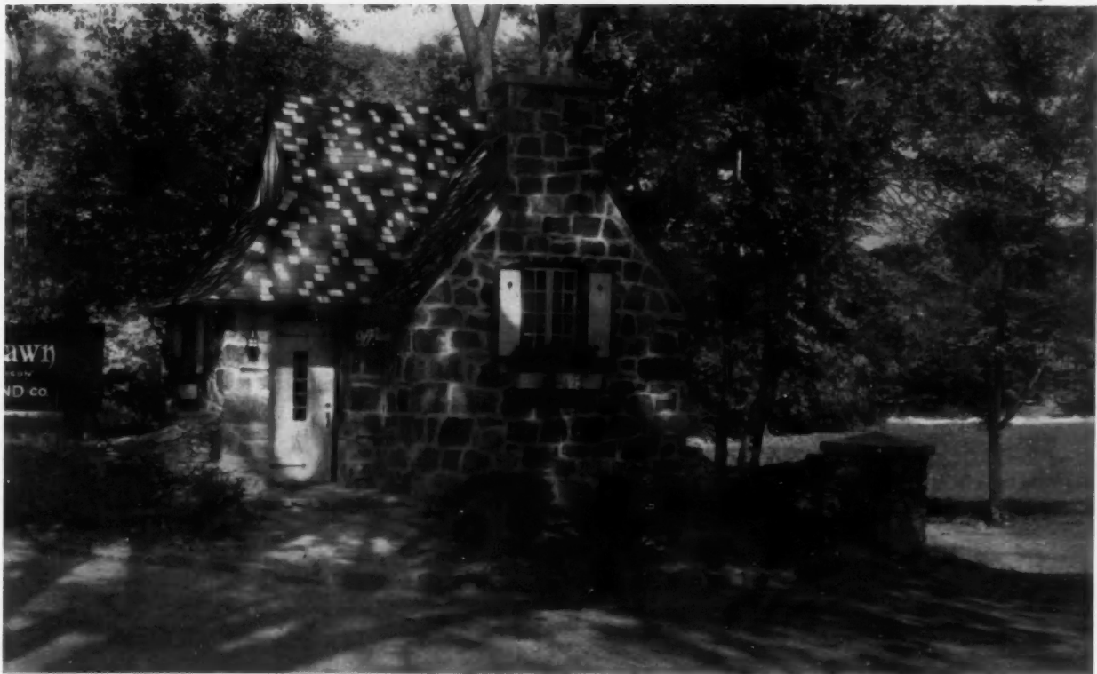
OFFICE OF THE HOMELAND COMPANY, HASTINGS, N. Y. JOSEPH EMMETT KELLY AND WILLIAM CAIN, ARCHITECTS
