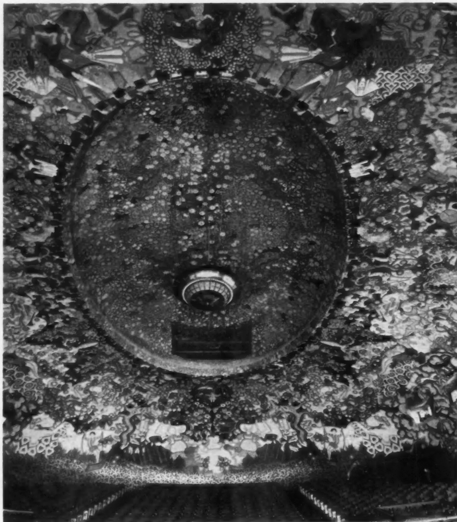
Detail of Ceiling, Ziegfeld Theater, New York Joseph Urban & Thomas W. Lamb, Architects
