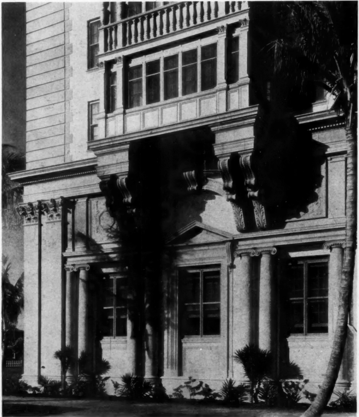
Detail of Minor Facade, The Breakers, Palm Beach
