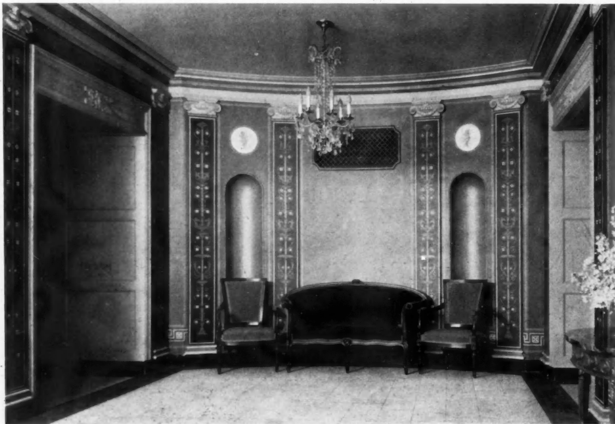
Pompeian Room, Stevens Hotel, Chicago Holabird & Roche, Architects
