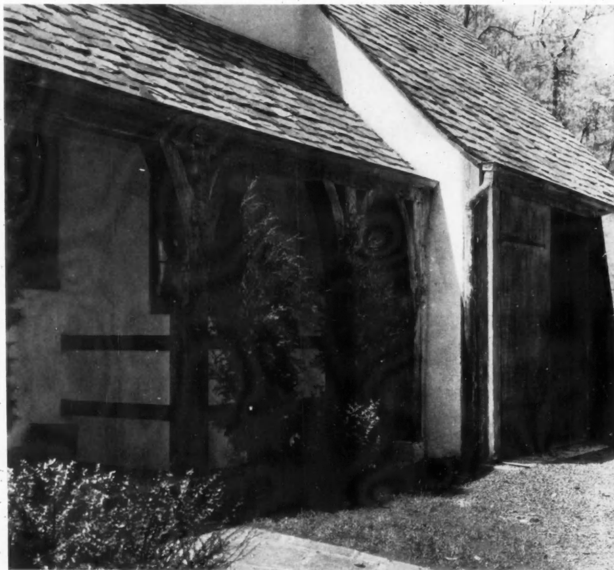
Detail, Garage of Gerald M. Lauck, Esq., Upper Montclair, N. J. Frank J. Forster, Architect
