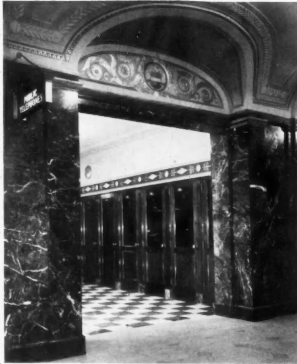
Telephone Lobby, Stevens Hotel Holabird & Roche, Architects
