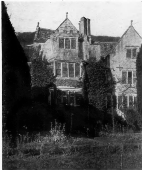
Detail of Main Facade, Owlpen Manor House
