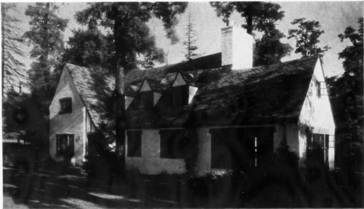
House of Wilbur Brundage, Esq., Douglaston, N. Y.
