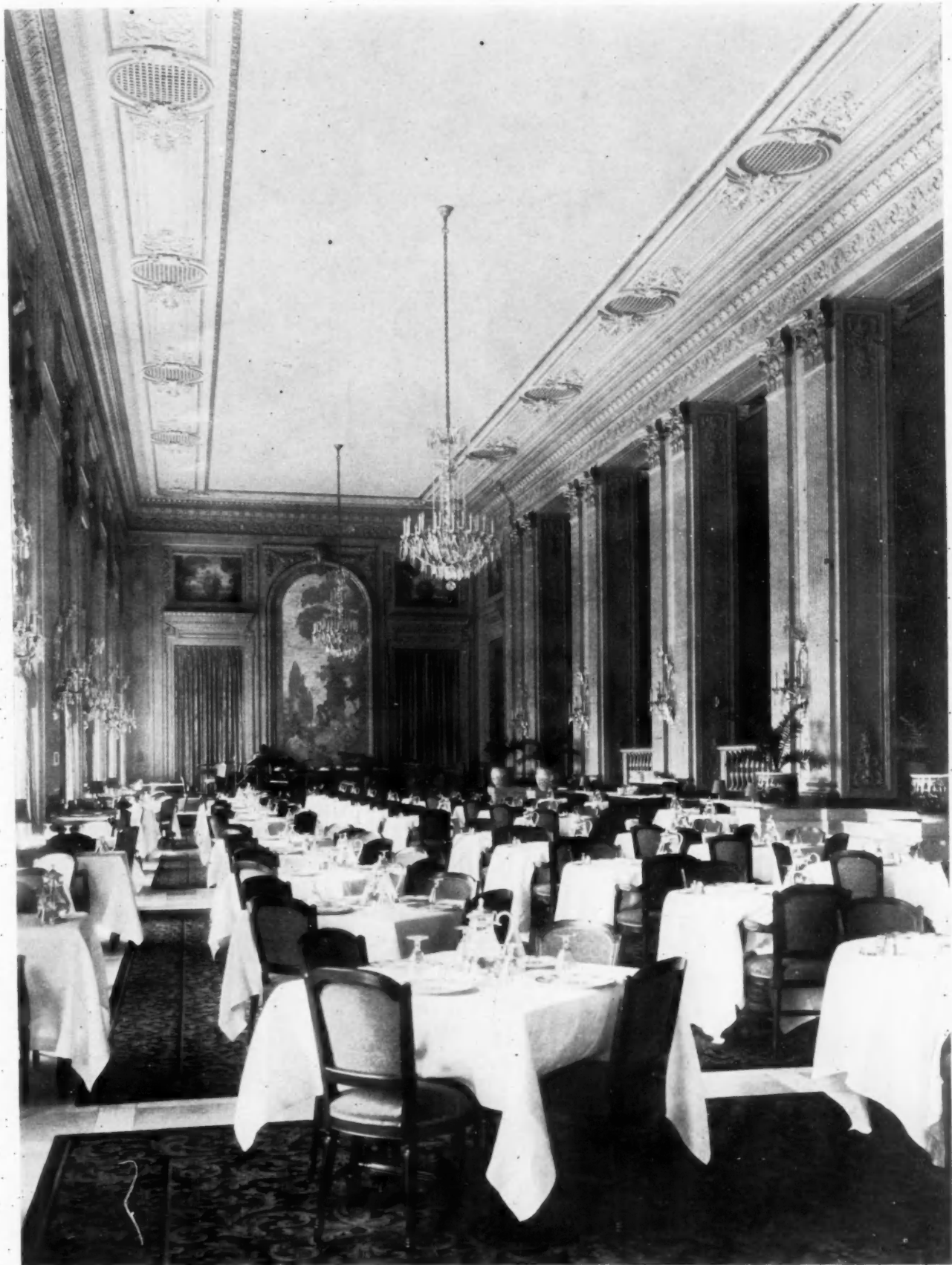
MAIN DINING ROOM STEVENS HOTEL, CHICAGO HOLABIRD & ROCHE, ARCHITECTS
