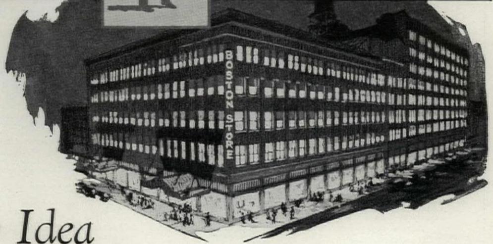
Boston Store, Milwaukee, Wis. 270 Cremax Globes were used in relighting two departments. Installation by Julius Andrae & Sons Company.
