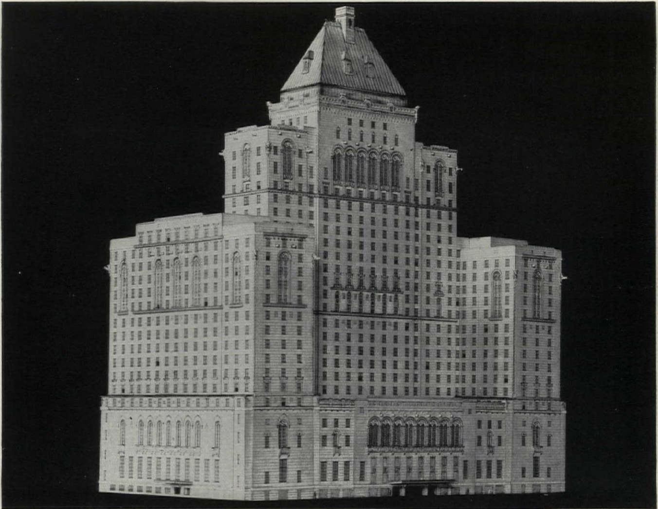
Royal York Hotel, Toronto. Ross & MacDonald, Architects. VARIEGATED Indiana Limestone
