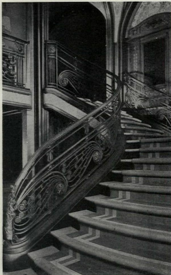
Stair Rail, S. S. Paris, French Line R. Bourvens de Boijen, Architect
