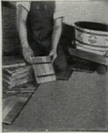
A complete unit of four flooring strips, splined together
