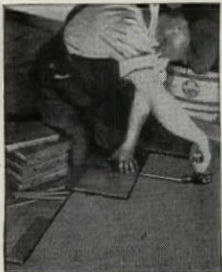
Driving in the wooden slip tongue
