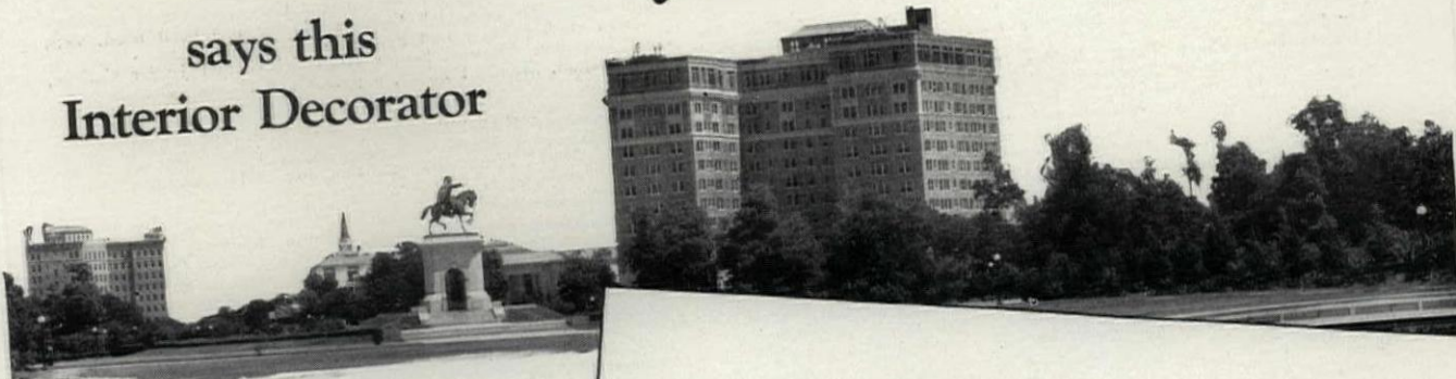
For interiors at the Warwick, fine apartment hotel of Houston, Texas, almost 200 gallons of Barreled Sunlight were used
