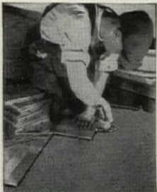
Slight tapping quickly fixes the block in position
