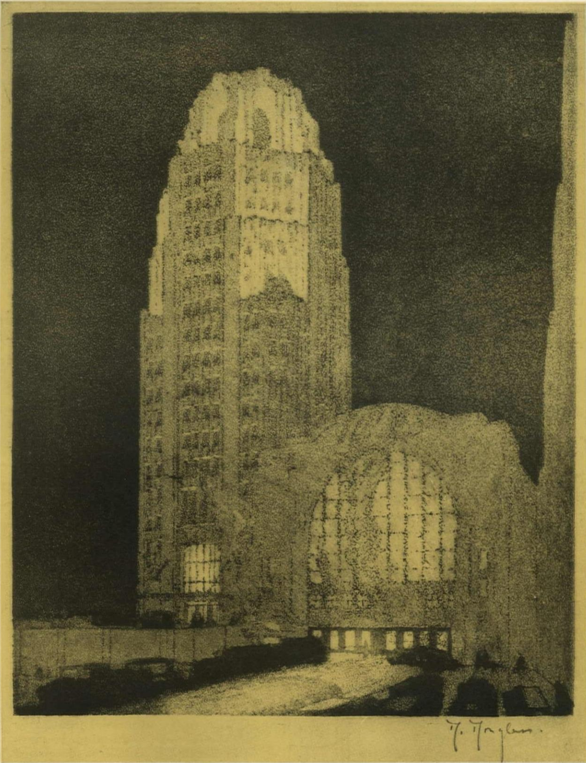
A Donald Douglass Aquatint study of the New York Central Railroad Station, Buffalo, N. Y. ~ Alfred Fellheimer and Steward Wagner, New York, Architects ~ Walsh Construction Co., Syracuse, N. Y., General Contractor ~ Chippewa Plumbing Co., Buffalo, N. Y., Plumbing Contractor ~ William E. Shattuck, Buffalo, N. Y., Heating Contractor . . . Jenkins Valves were selected for the plumbing and heating of this station Jenkins Bros. ~ New York ~ Boston ~ Philadelphia ~ Chicago . . . Jenkins Bros. Ltd. ~ Montreal ~ London.
