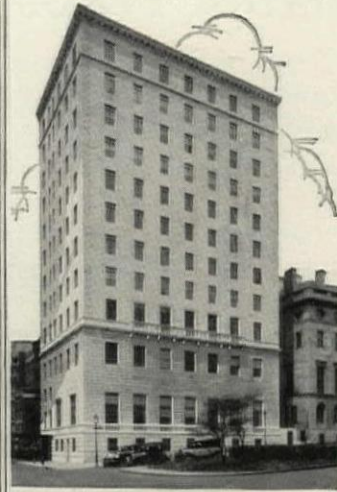
Second award in the "over six stories" class to York & Sawyer, Architects, for 660 Park Avenue — a cooperative building.
