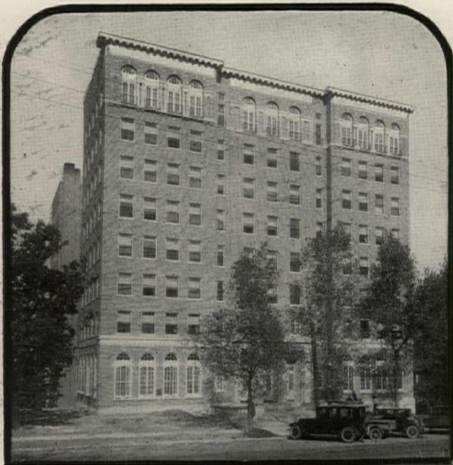
HIGHLAND PLAZA APARTMENTS, BIRMINGHAM, ALA., protected by Genasco Standard Trinidad Built-up Roofing. Architects: Denham, Van Kuren & Denham, Birmingham. General Contractors: Smallman-Brice Construction Co., Birmingham. Roofing Contractors: Concrete Products Co., Birmingham.
