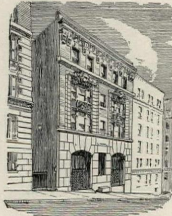
Interborough Rapid Transit Co. Sub-Station 606 West 143rd St., N. Y. C.
