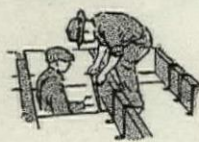
Hanging ceiling slabs
