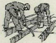
Grouting ceiling slabs
