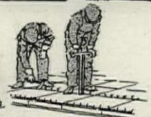
Tying the reinforcement together.
