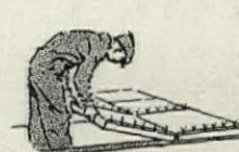
Laying Gypsteel floor slabs
