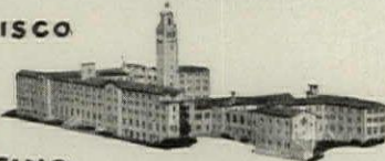
St. Joseph's College, Cupertino, Cal. Architect: L. J. Devlin, San Francisco.
