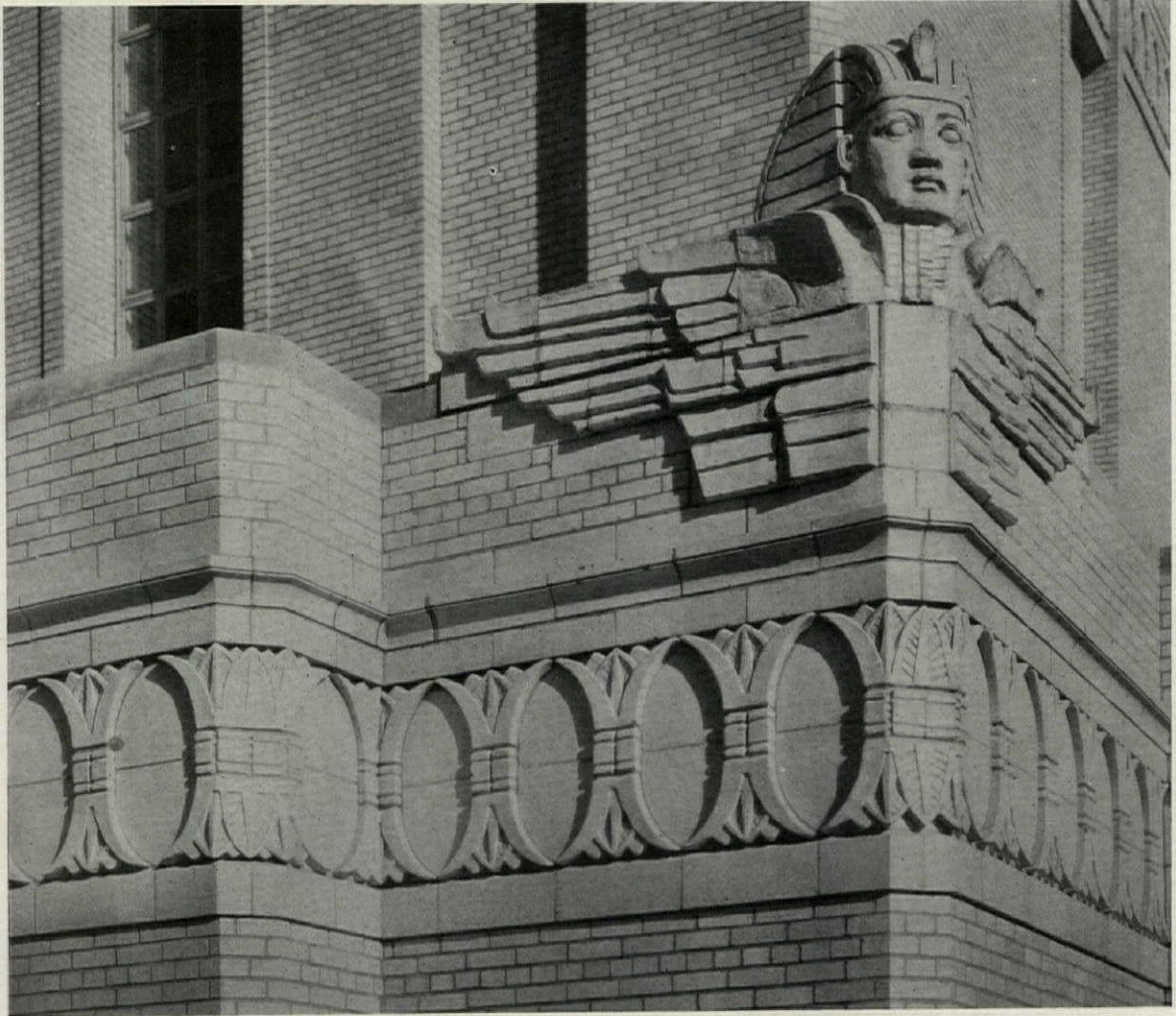
Corner Detail. Chase National Bank Building, New York Graham, Anderson, Probst & White, Architects
