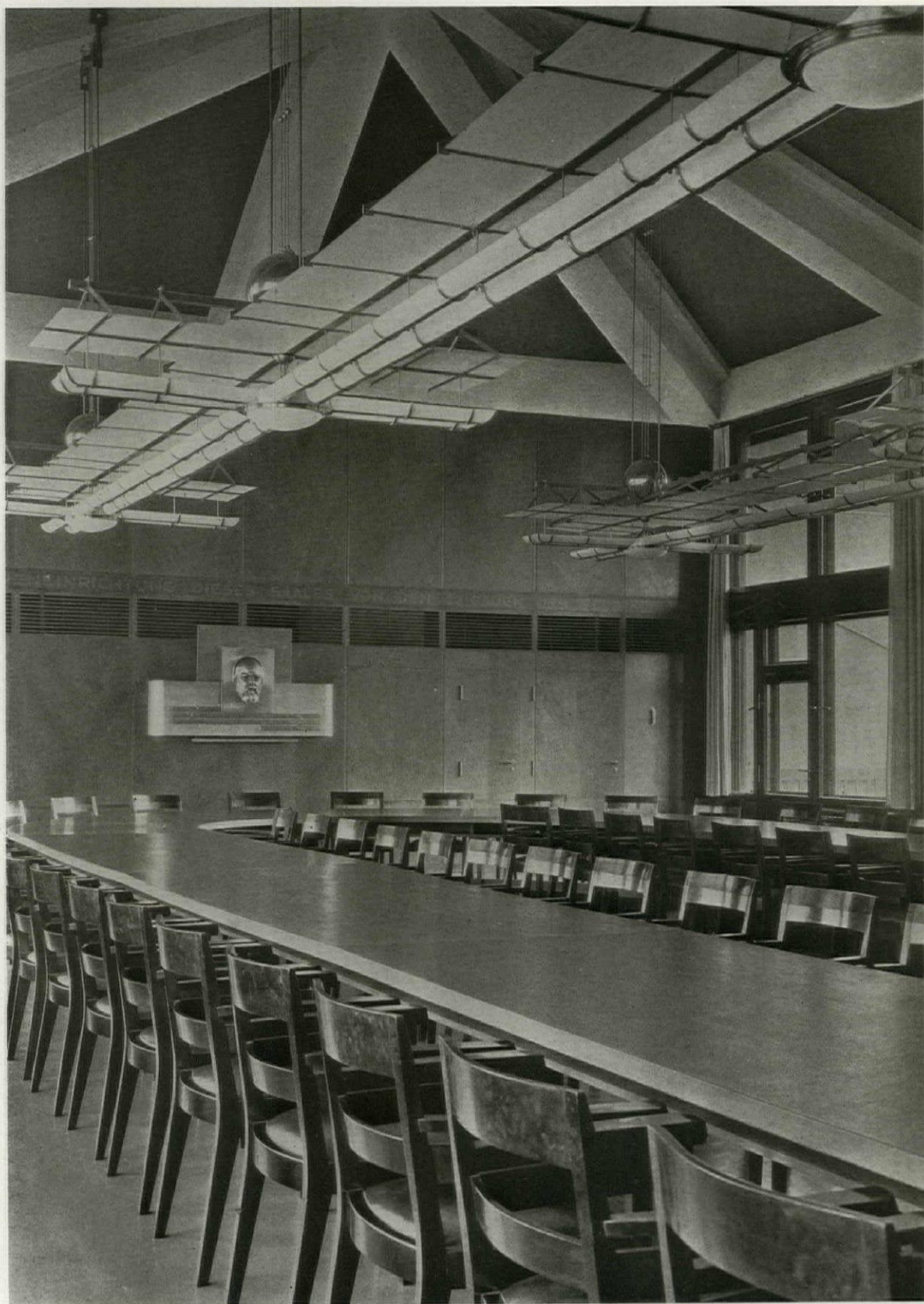
BOARD ROOM. BOOKPRINTERS' LABOR UNION MAX TAUT, ARCHITECT
