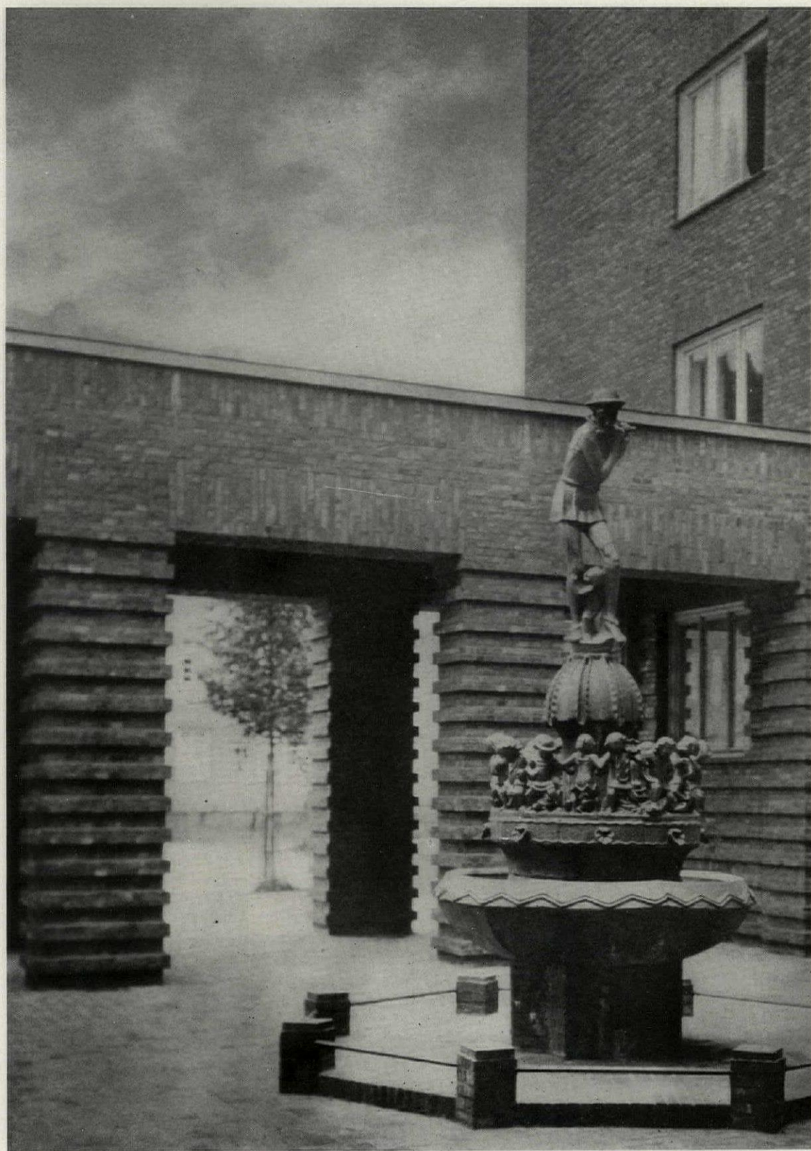
COURT, APARTMENT HOUSE, HAMBURG
