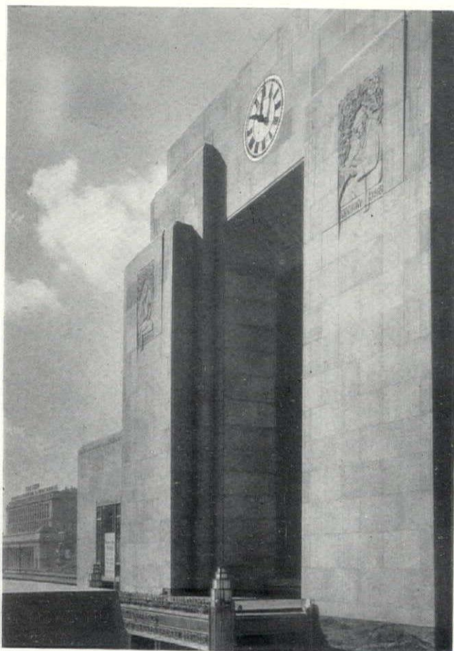
SOUTH WING, EAST TERRACE AND MADISON STREET ENTRANCE CHICAGO DAILY NEWS BUILDING HOLABIRD & ROOT, ARCHITECTS
