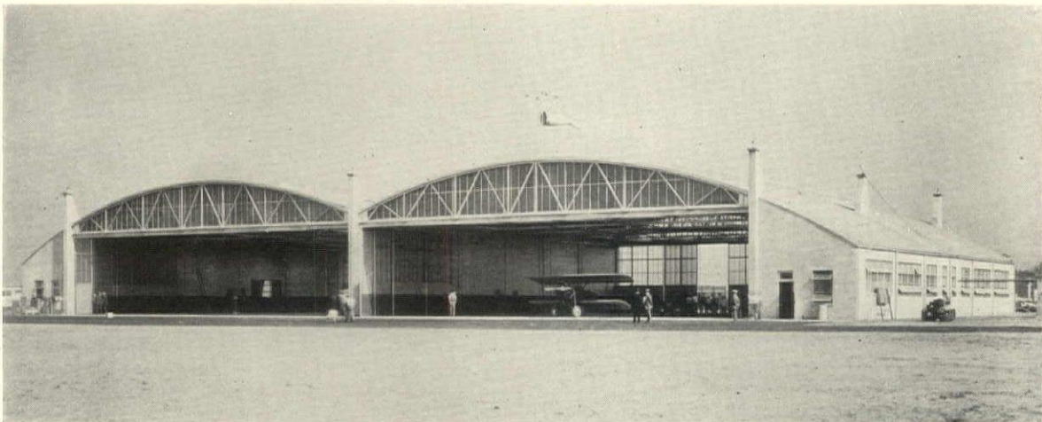
Fireproof Hangars at the Central Airport, Camden, N. J., Fifteen Minutes From the Center of Philadelphia
