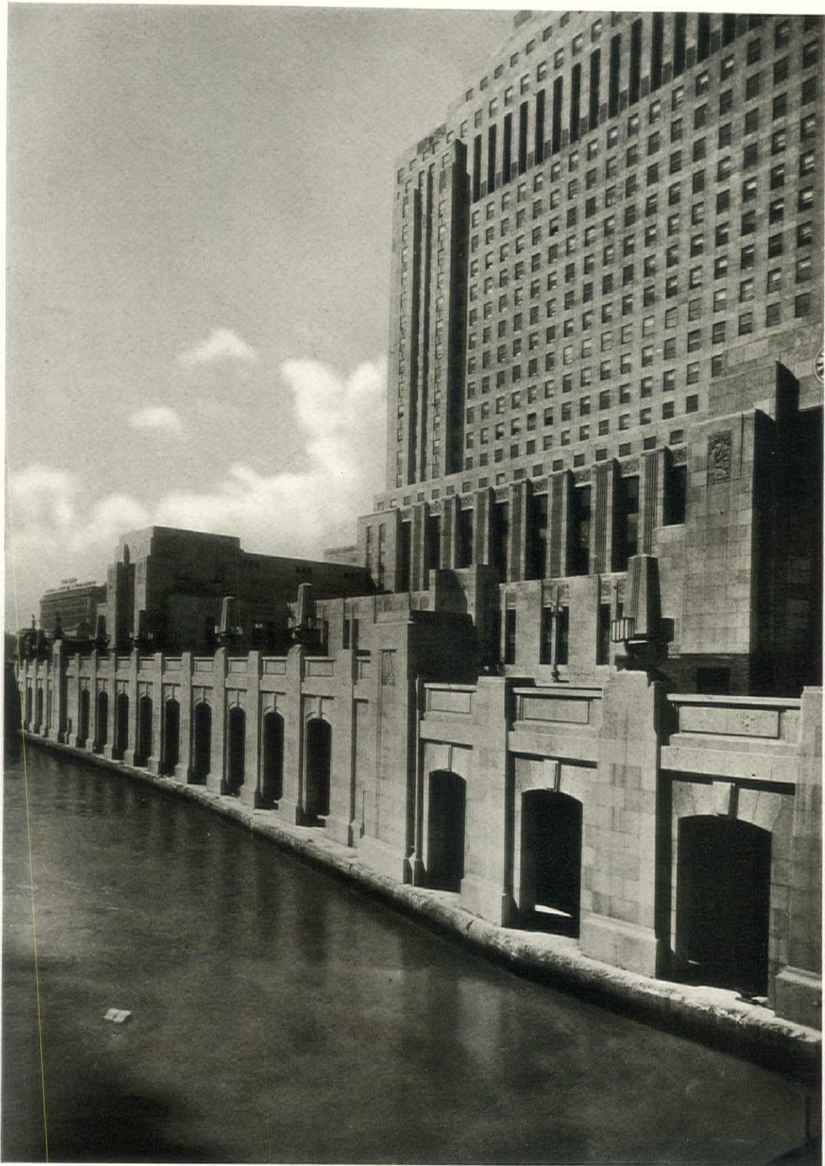
TERRACE CONCEALING RAILROAD CHICAGO DAILY NEWS BUILDING HOLABIRD & ROOT, ARCHITECTS
