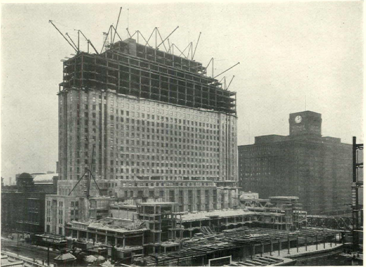
The Chicago Daily News Building Under Construction
