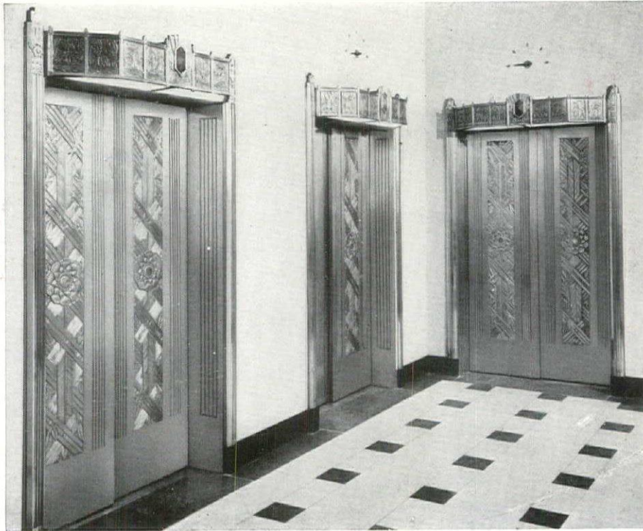
Chicago Daily News — Elevator Doors, nickel silver. Architects: Holabird & Root.
