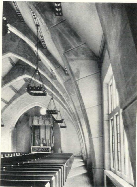
A view of the finished interior. The arches are concrete but the window jambs and muntins are of stone. Below—a progress photograph, showing the main arch forming
