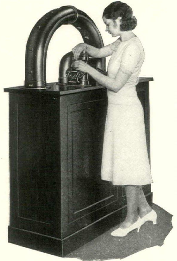
Oval leather carriers are used wherever the material to be transported, because of bulk or nature, more conveniently fits this shape. Destination of contents indicated by movable numerals in cover. Home station of carrier is usually painted on its side.
