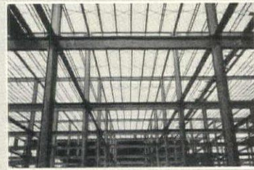
Rigid Bridging accurately spaces Kalmantruss Joists
