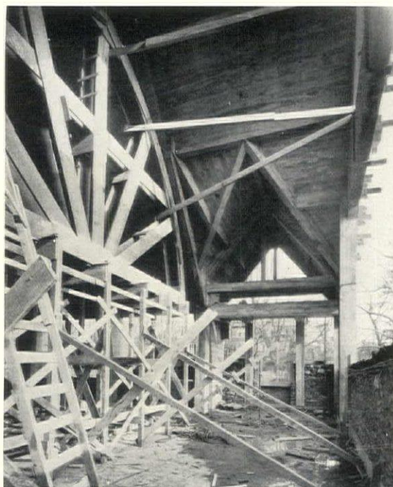
A view of the finished interior. The arches are concrete but the window jambs and muntins are of stone. Below—a progress photograph, showing the main arch forming
