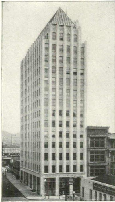
Protective Life Insurance Co. Building, Birmingham, Alabama Warren, Knight & Davis, Architects. Nailcrete used as nailing base for copper roof.
