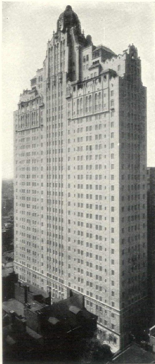
Drake Apartment Building, Philadelphia, Pennsylvania, is equipped with Frigidaire. Ritter & Shea, Architects, Murphy-Quigley, Builders.
