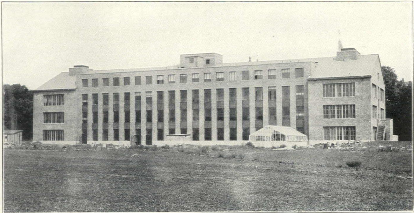
In this General Science Building of Antioch College, Yellow Springs, Ohio, 28 tons of 16, 18, and 22 gage galvanized INGOT IRON was used for the duct work, which eliminates moisture and corrosive chemical fumes from 27 laboratories. INGOT IRON was chosen on the strength of its eminent past performance under all kinds of corrosive conditions, a service record embracing a quarter century.
