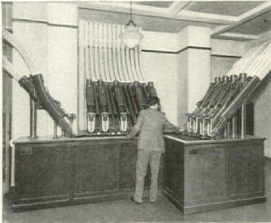
Central Tube Station, State Mutual Life Assurance Co., Worcester, Mass. Parker, Thomas & Rice, Archts. Like in a telephone switchboard, lines reach out to provide communication to all departments.
