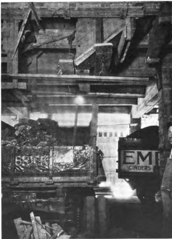
Truck loaded with refuse received from chute that led into a heavily reinforced bin on second floor
