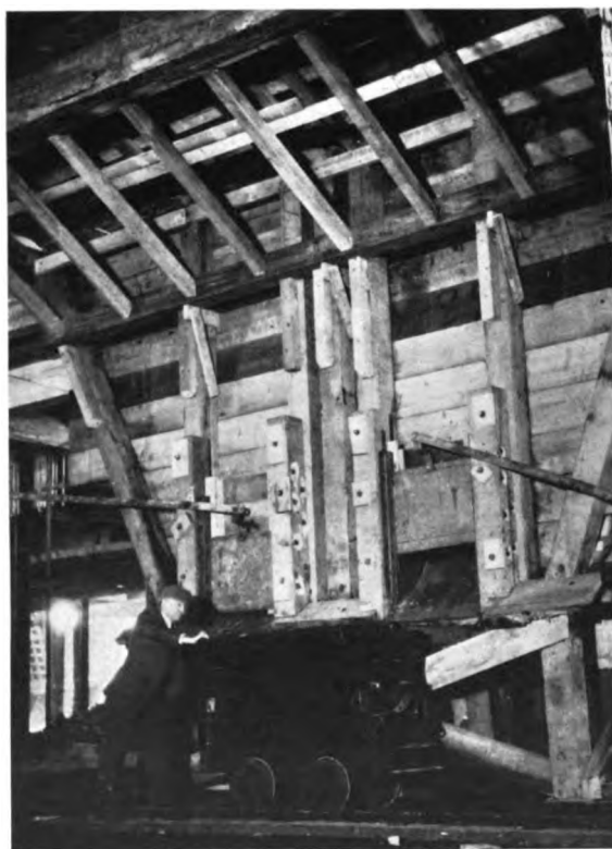
Carload of brick being pushed away on industrial tracks from large brick hopper in first basement
