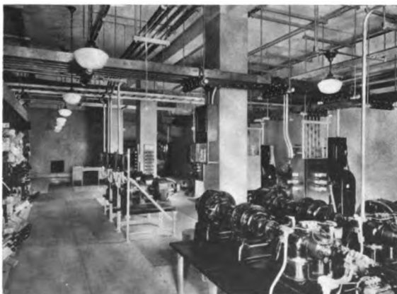
Power Machine Room.
