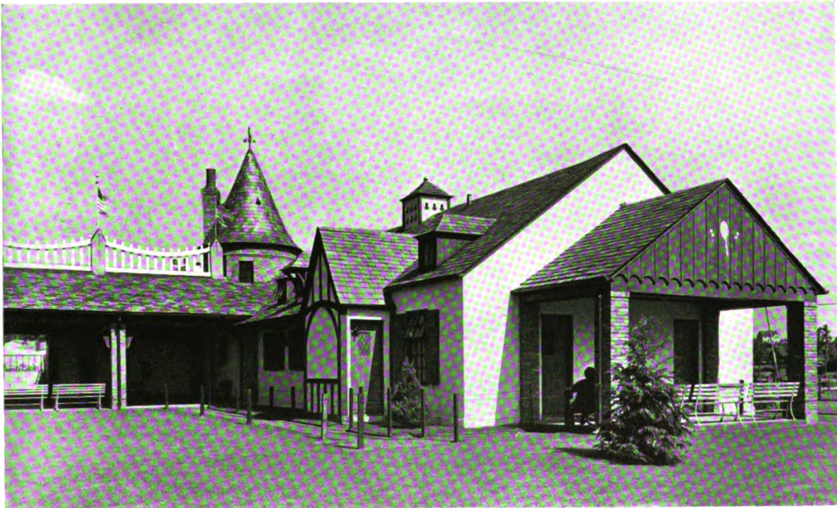
THE LOCKER ROOMS FROM THE ENTRANCE PLAZA
