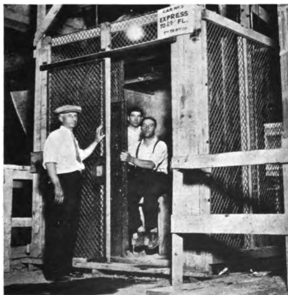
Mine shaft car used for temporary service. Note heavy gauge wire which encloses the shaft, and the safety gate which prevents car motion if open
