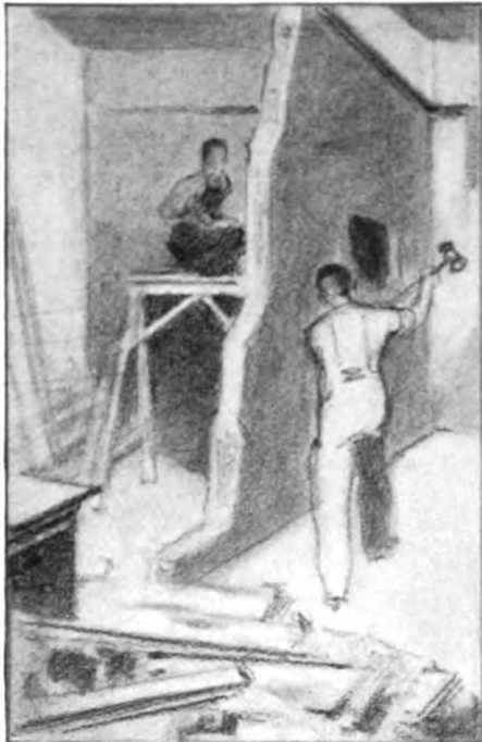
TENANT A MOVED OUT . . . New tenant required entirely new layout. Down came plaster walls . . . a total loss to the building. If they had only used modern movable partition! More beautiful, too, in rich American walnut.
