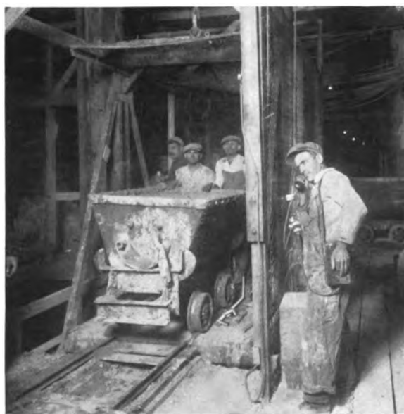
Mortar-filled rocker dump car ready for ascent. Note that signalman has all controls on his person, and that safety dog had not yet locked wheels
