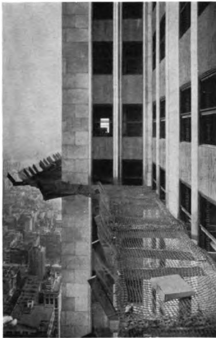
Rope net catch-all for light objects, located beneath the one on the right
