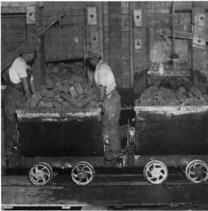
Tandem cars being loaded from hoppers. Note the water spray wetting down the brick on the right
