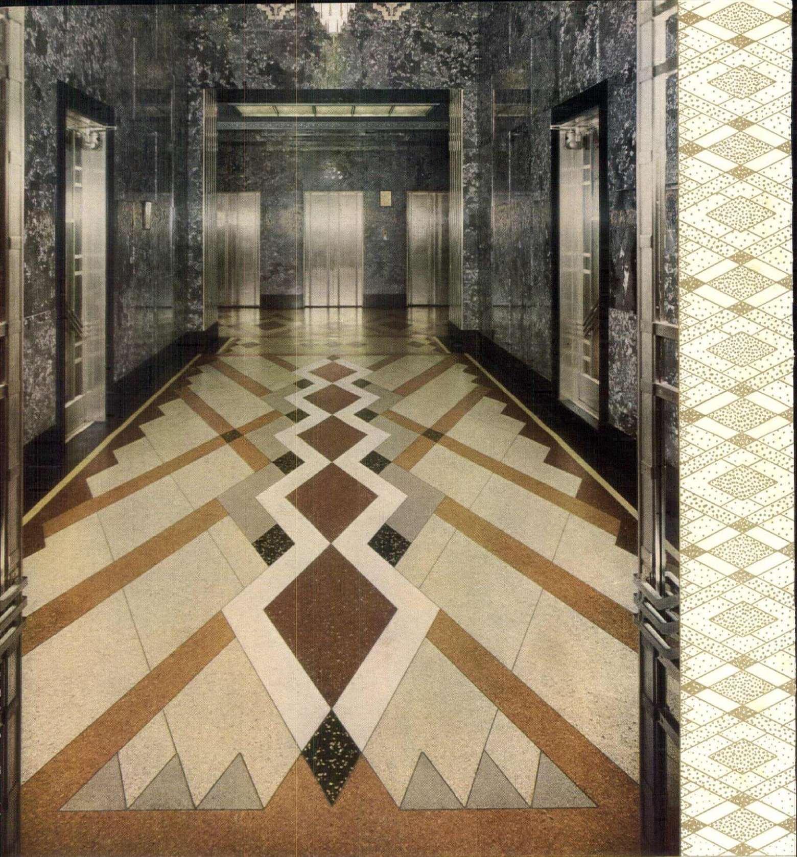
Terrazzo floor in the Medical Arts Bldg., Pittsburgh. M. Nirdlinger, architect; Patrizio Art Mosaic Co., terrazzo contractor, both of Pittsburgh. Atlas White portland cement used.
