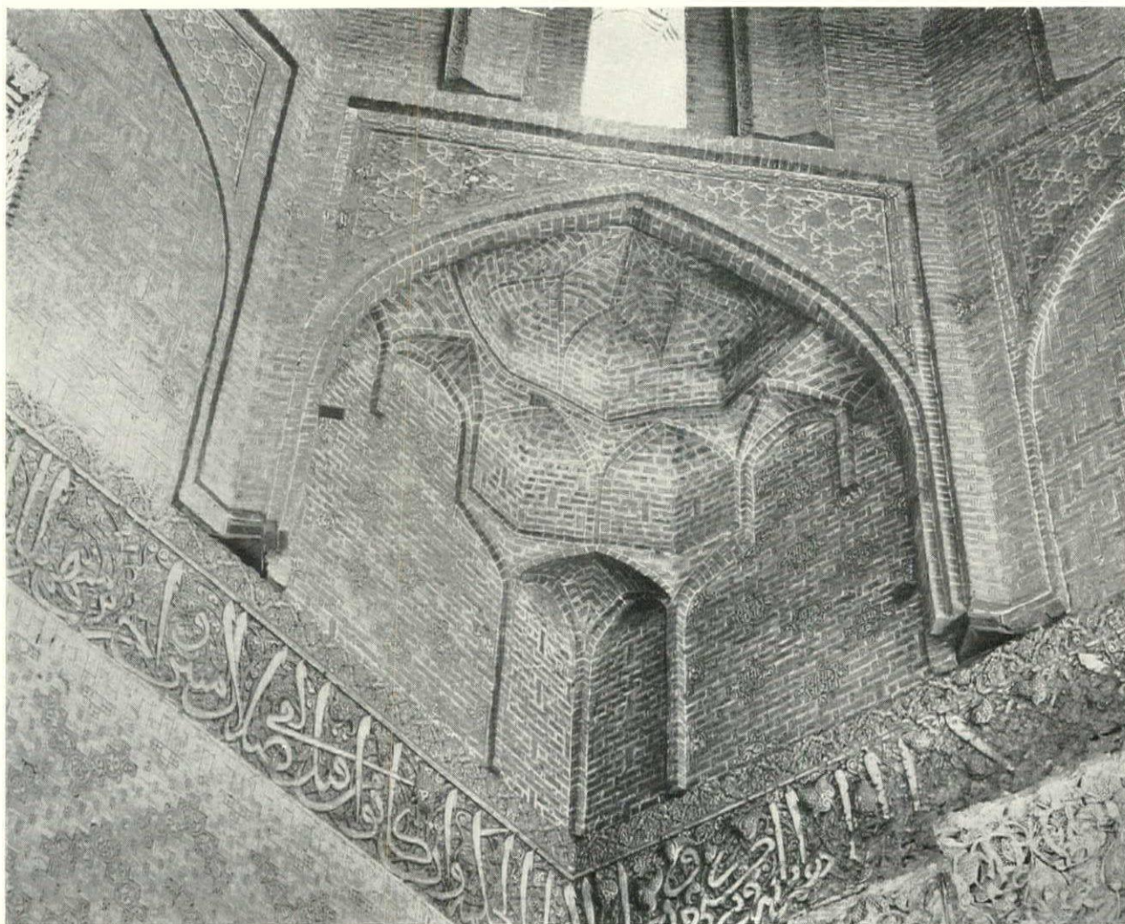
Above is a view of the dome of the Sanctuary in the Jume' Mosque in Varamin. The construction of the squinch, similar to the one shown below at the left, is typical of Fourteenth Century work. Below the squinch the Kufic characters spell a verse, probably from the Koran. At the bottom right is a detail of the southeast archway in the Jami Mosque, which although more elaborately patterned than the brickwork of today, is simple in comparison to the other examples shown. The squinch at the bottom left is in the great dome chamber of the Jami Mosque, Isfahan
