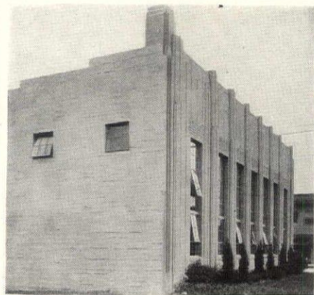
ONE SIDE WAS SHIPLAP—the other Douglas Fir Plywood! Observe the difference between the left sidewall of this bank building—and the smooth front wall obtained by the use of Douglas Fir Plywood. Douglas Fir Plywood is a perfect form material for flat surfaces, and an ideal backing for all kinds of pattern and reverse-mould work.
