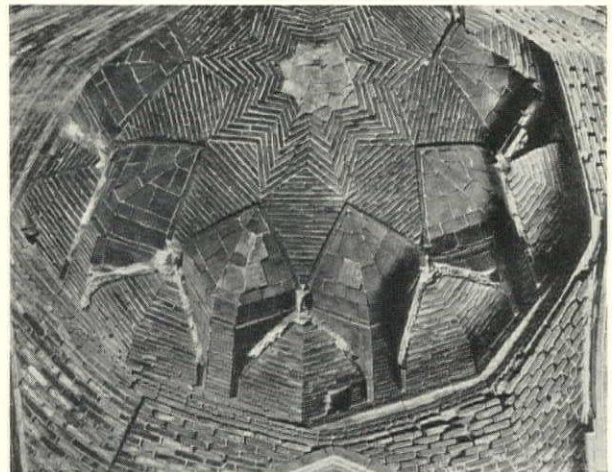
Another illustration of cusping, this one taken from the Jami Mosque. The center inlay has been destroyed
