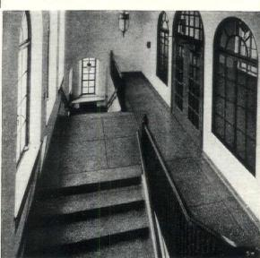
Terrazzo is ideal for stairs and hallways. Placed in a plastic condition, it can be shaped to any form. Or it can be pre-cast in special shapes and placed in units.
