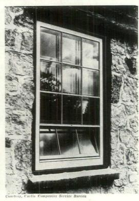
Left, inside winter window, metal frame, wood casement sash; right, outside winter window with vent, wood frame, double-hung wood sash
