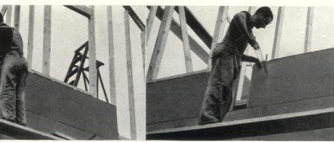
Eliminates mis-nailing-studs are in plain view always-don't have to be exactly centered.
