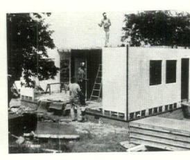
Ex-ray of the conventional houses' frame construction is presented above, left. Asphalt shingles were applied to shingle battens, separated only by a layer of tar paper. More substantial are the cross-braced and insulated plywood panels, right. Taken at 1:30 p. m., the picture indicates the speed with which the prefabricated houses were erected—seven hours earlier only the poured concrete foundations were in place.
