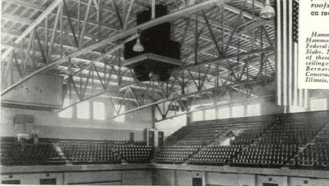
This is the modern, permanent roof-deck, of individual factory-precast concrete slabs — strong, dense, yet light in weight to save structural steel.
