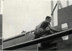
5 Tongue and Groove Joint makes it easy to slide short pieces into place.
