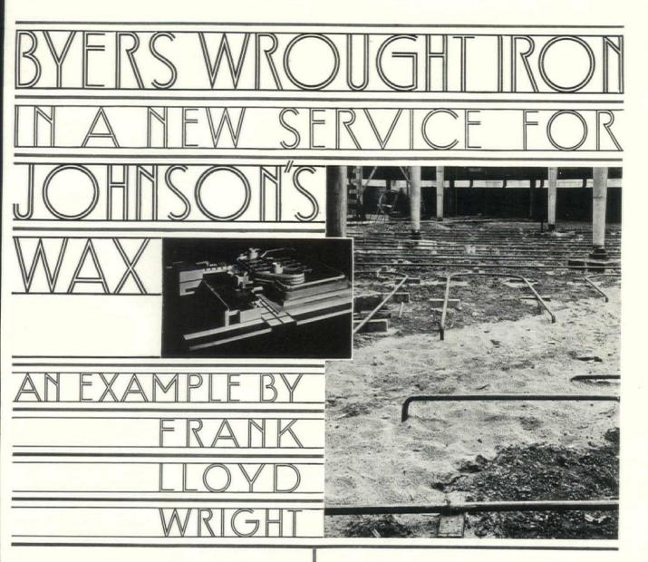
In heating, also, the modern office building of S. C. Johnson & Son, Inc., strikes a unique note. Steam pipes of Byers Wrought Iron imbedded in the floor combine with tempered ventilating air to warm the structure.
