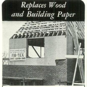
Why ask clients to pay for both insulation and sheathing? Fir-Tex provides both in one board, at one moderate cost.
