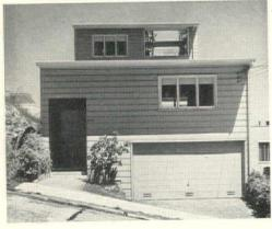
A workable solution of one of the vexing problems of the city house, where formal and service entrances must often be combined, the outdoor locker adjoins the vestibule and provides space for meters, refuse, etc., accessible directly from the street and yet out of sight.
