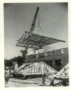
Rocf framing is meanwhile assembled on the ground, raised into place in four sections by a giant crane.
