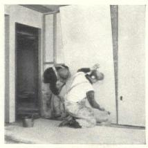
Putting Mengel Bord sheets in place. Edges glued to strips on stud.
