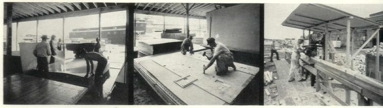
2. 3. Picture 1 shows Homasote sheets being wet down before use, in order to swell sheets so that subsequent shrinkage will stretch material on frames. 2 shows precutting of openings for electric outlet boxes, 3 precutting of studs and other framing lumber outside the plant.
