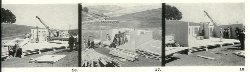
16, 17, and 18 show successive stages in the erection of wall panels on the floor platform. Assembly is handled in two stages, with a fifteen minute intermission (during which the crew shifts to the next house in the row) for the installation of prefabricated plumbing.
