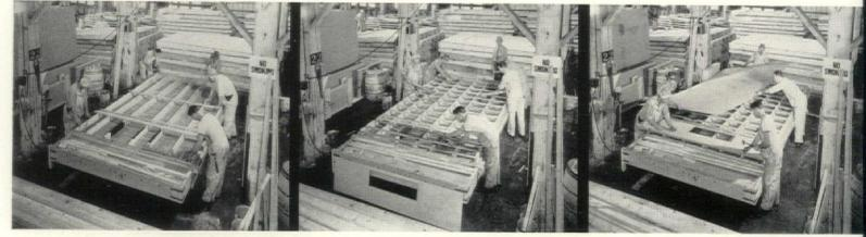
7. 8. 9. 7, 8, and 9 show fabrication of a roof panel, complete with overhang and screened vent. Homasote ceilings are applied to furring strips on the bottom of the rafters, tops of rafters canted to receive sloping roof at Job. Four such panels, plus seven smaller units, roof one house.
