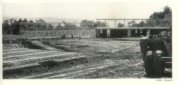
construction. An orderly plan has been related to a panel system of field fabrication in which the members are nailed together on the floor platform and then raised as a unit. When the stud panels are fastened together the end studs are doubled to form four-inch posts. This is clearly illustrated in the photograph at the left and in the structural details below. Brick is used as a veneer on some of the first-floor walls. Construction cost per unit averaged \$3.098.
