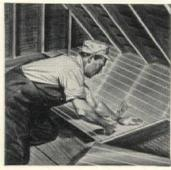
Steel Insulation made from U.S.S rustresisting Copper Steel terne plate. Thoroughly proved in hundreds of installations. Reflects 95% of radiant heat.
