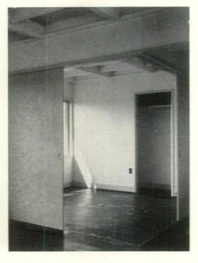
Interior photographs (left) show the attractive appearance of the underside of the exposed roof beams. Sliding doors open the corner of the bedroom into the living room, doubling its apparent size. Details below show still another panel roof construction, as well as horizontally-sliding windows and closet details, and kitchen cabinet doors.
