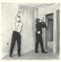
Sanding off glue at joints of Mengel Bord, and applying trim before papering and painting.
