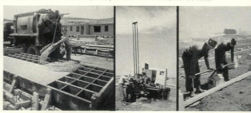
SITE PREPARATION. Picture 11 shows form for casting foundation piers in batches of 84 piers. 12 shows hole-boring apparatus for drilling foundation holes, and operation of setting piers.
