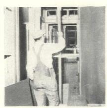
Applying glue to Mengel Bord strips on studs, before installing Mengel Bord sheets.
