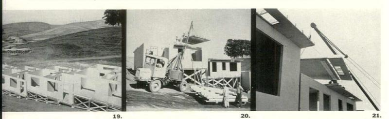
19 shows completed walls, ready to receive roof panels, which are lifted into place by a light traveling crane (20 and 21), covered with roofers in the conventional way, and surfaced with roll roofing (22). 23 shows application of trim, the larger picture below completed houses.
