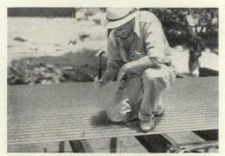
Nailing corrugated sheets to Stran-Steel floor joists. This forms a working deck during the early stages of construction. Later, concrete will be poured over the metal sheets, forming a safe, silent, fireproof floor.
