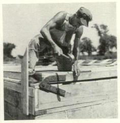
Floor-wall hinge aligns prefabricated wall section, facilitates its erection, is later removed.
