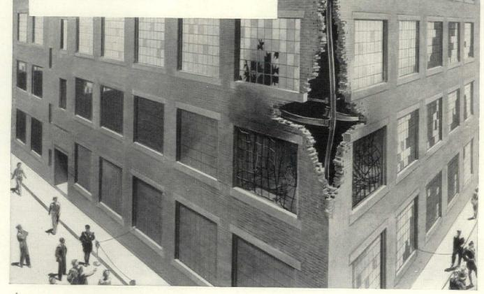
Anyone who confuses a non-combustible with a truly fireproof building needs only to see what havoc can result from a localized fire in a so-called non-combustible building. Small fires that raise temperature to only 1000° F. may cause 9½ inch expansion in a 100-ft. steel truss . . . enough to wreck brick walls or dangerously distort columns. Even at 900° F., some steel columns may be seriously impaired in load-bearing ability!
