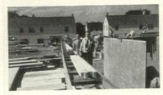
Conveyor at 538-unit Newport, R. I. USHA project delivers pre-cut lumber to Jig tables where wall frames are fabricated.
