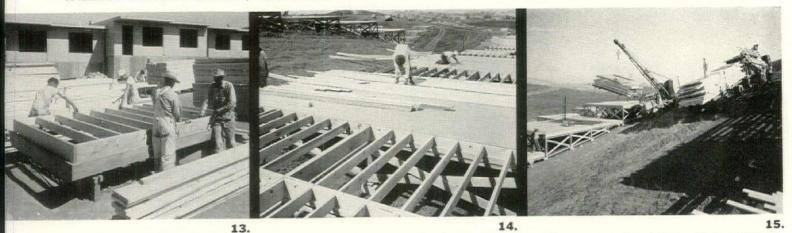
Pictures 13 and 14 show site-assembly (on a special jig table) of floor framing panels and erection on post foundations. Single thickness flooring is laid in the conventional way. Picture 15 shows traveling crane unloading wall panels from trailer truck.
