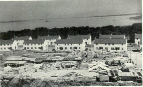
Completed buildings on the attractive Rhode Island site form a backdrop for the site-prefabrication machinery. Long convas-covered platform is a huge Jib table. Architects: Howe & Prout of Providence. Contractor: M. Spinnelli & Sons of Boston.
