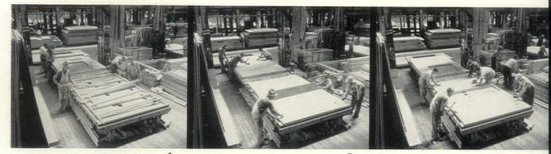
4, 5, and 6, show assembly of a typical, room size wall panel on a "Jig table" marked off in modular units. Door opening is cut after the sheet is applied, using plywood template and skill saw; sheets are glued and nailed to 2 x 3 studs, using mechanical glue spreaders.
