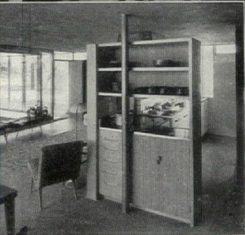
L-SHAPED PARTITION consisting of fireplace and cupboard unit screens kitchen from dining area without expense of door and full-height walls. Living area can be curtained off to provide extra sleeping space.
