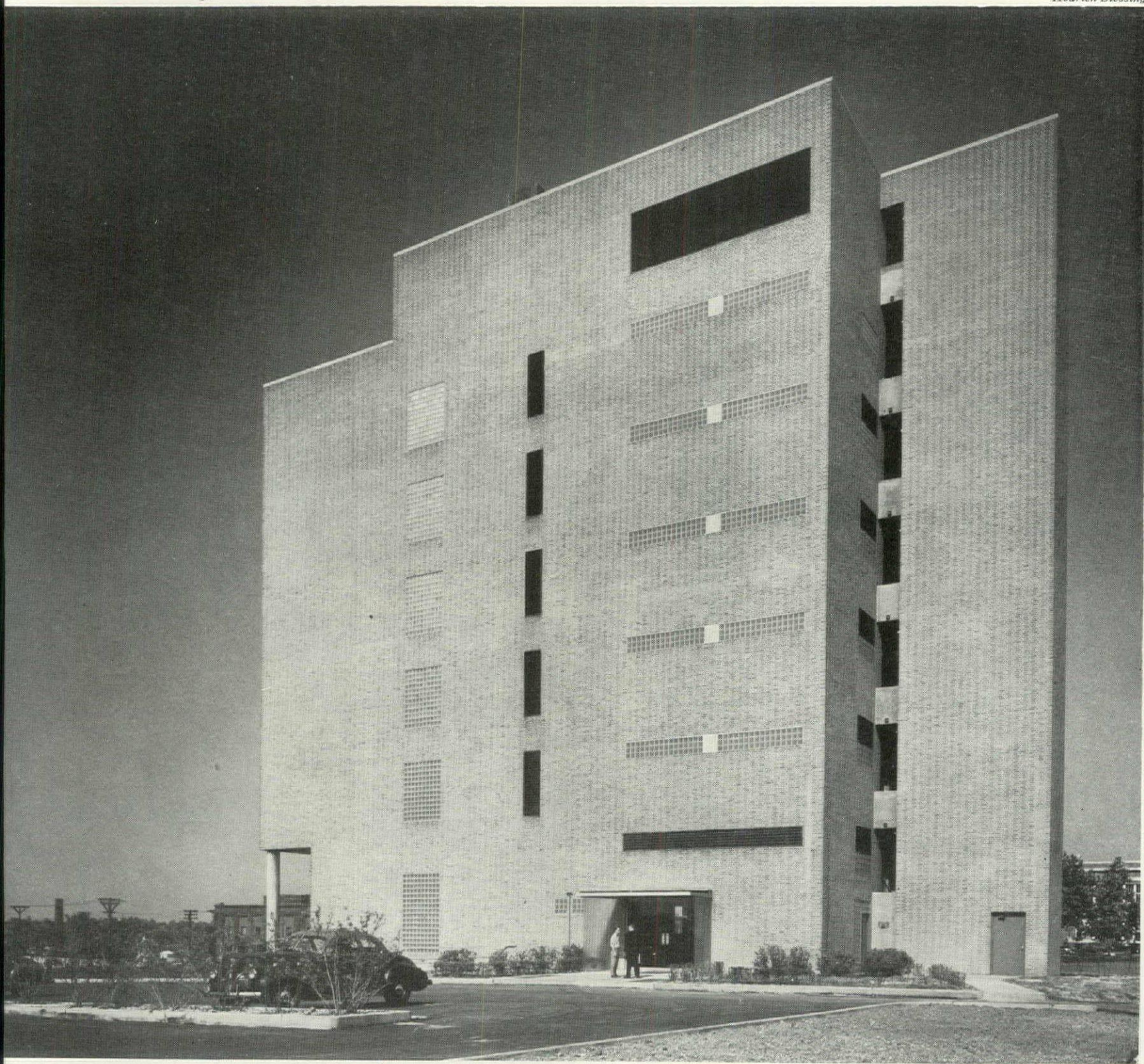
WEST EXPOSURE, ABOVE, IS BLANK, AS IS EAST EXCEPT IN SHOWROOM; NORTH AND SOUTH SHOW DIFFERENCE IN LIGHTING TECHNIQUES
