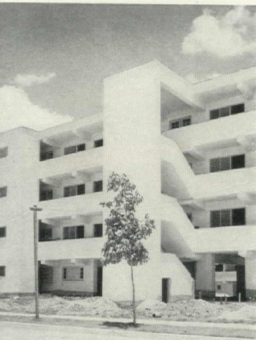
EACH APARTMENT BUILDING cost $155,000, has 30 two- and three-room units. Windows have only built-in wood blinds; balmy weather, absence of mosquitoes made glass and screens unnecessary.
