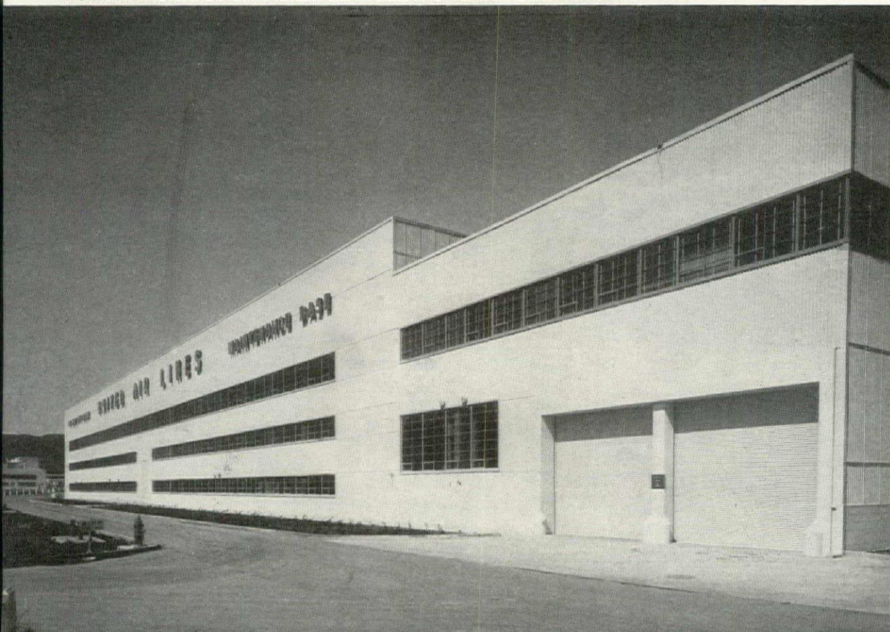
HORIZONTAL BANDS OF PROJECTED STEEL SASH EMPHASIZE LENGTH (485 FT.) OF MAINTENANCE SHOP
