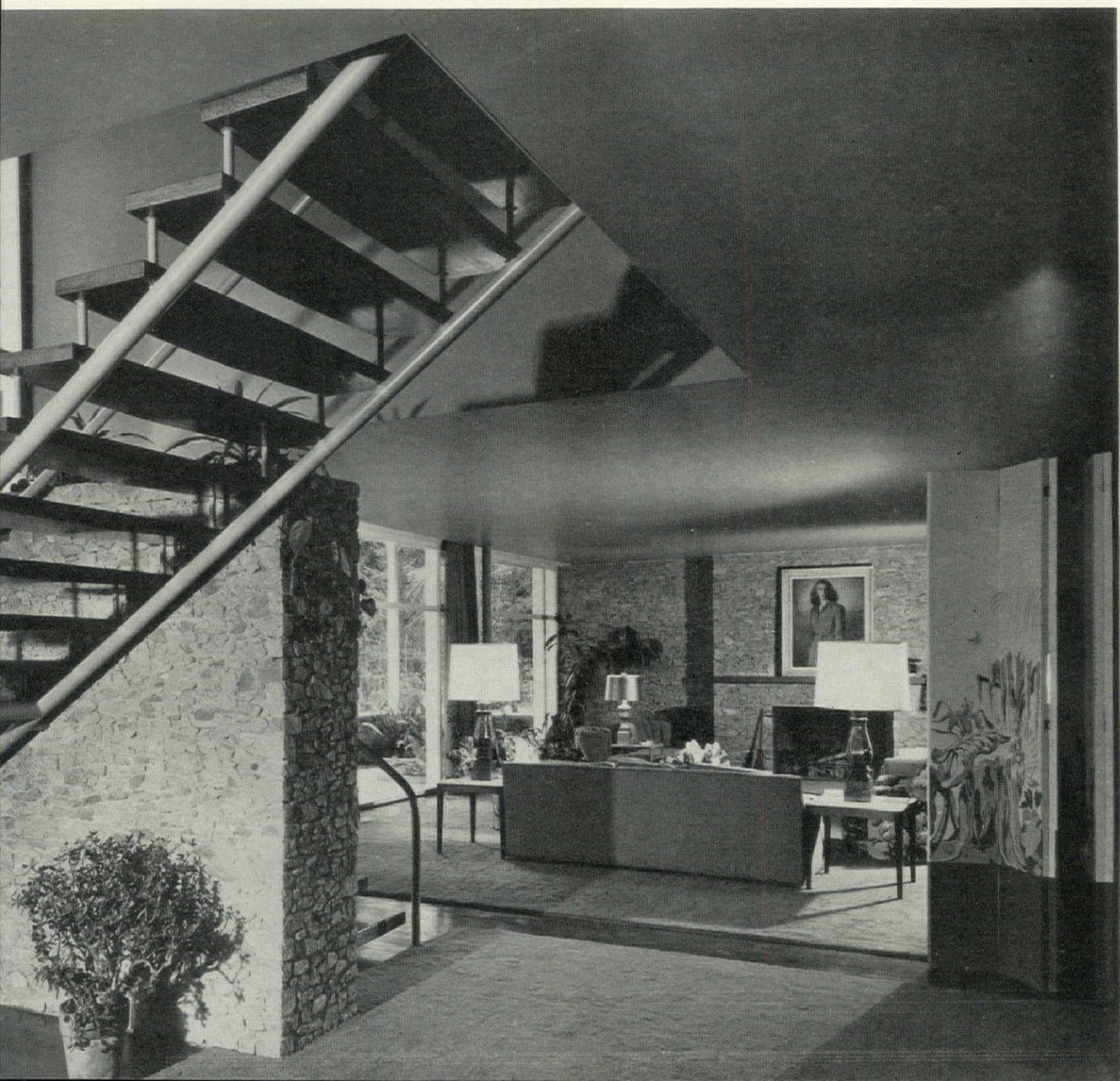
ING ROOM WITH SCREEN FOLDED BACK. UPPER STAIRS WHICH COULD NOT BE CANTILEVERED, MAKE USE OF SLENDER PIPE SUPPORTS
