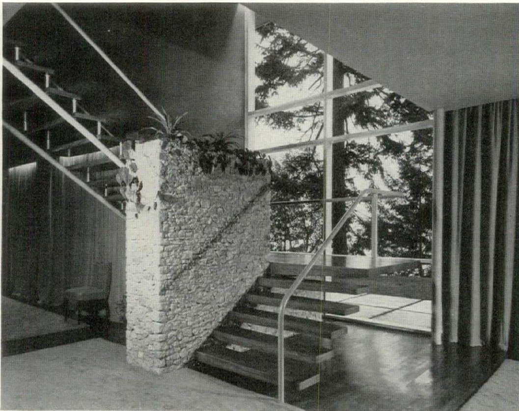
LOWER FLIGHT OF STAIRS IS CANTILEVERED FROM A CENTRAL BLOCK OF MASONRY
