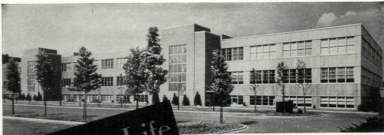
New building addition to Country Life Press, Garden City, N. Y., containing 110,000 sq ft of floor space with electrical raceways always quickly and conveniently available.
