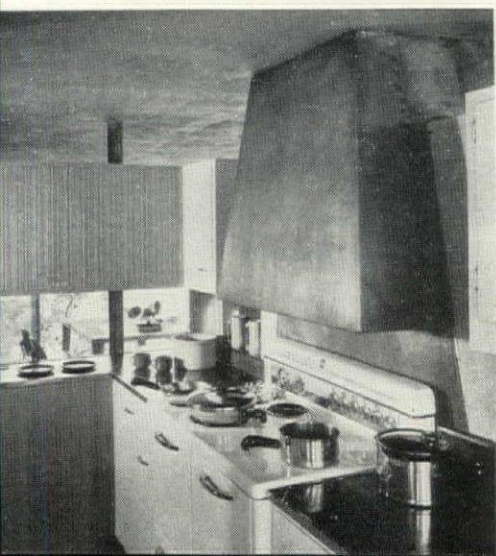
DOUBLE DUTY COPPER HOOD serves both fireplace and kitchen stove, carries cooking odors up the chimney. It also acts as a radiant heater, providing an estimated increase of 40 per cent in the heat supply. To right of hood is serving window for convenient passage of food and drinks to living room.
