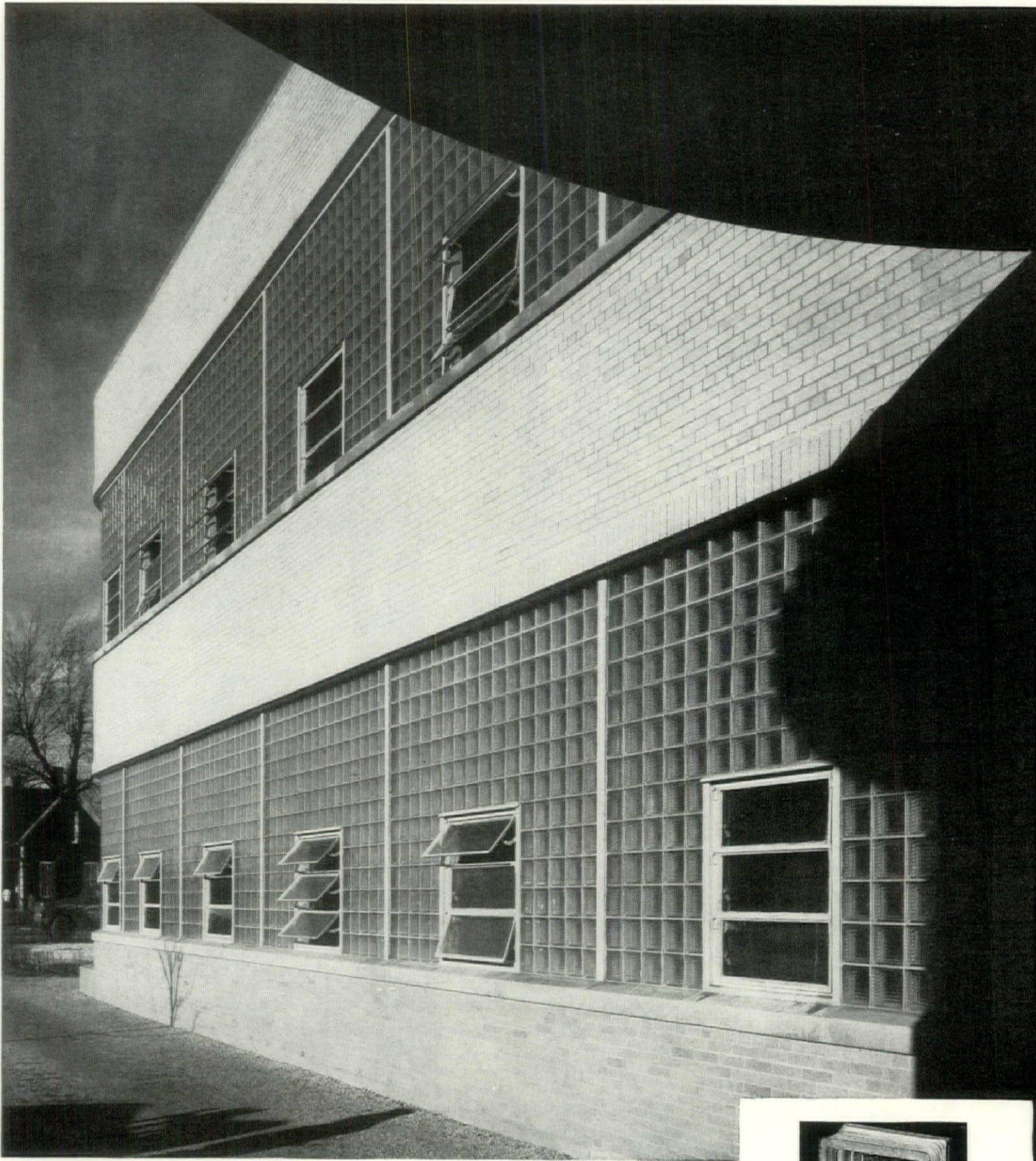
DEAN MILK COMPANY, HUNTLEY, ILLINOIS. ARCHITECT: VICTOR L. CHARN, CHICAGO. CONTRACTORS: RAGNAR-BENSON, INC., CHICAGO.
