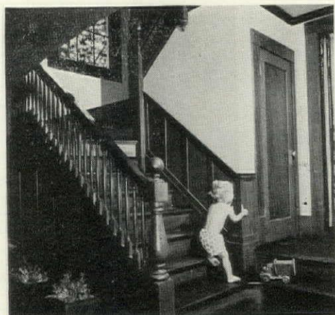
BRANCH: "Door frames and wainscoting serve as protectors against children and moving men. In the farmhouse the youngest child runs his greasy hand along the wall as he comes downstairs. Result: no damage."
