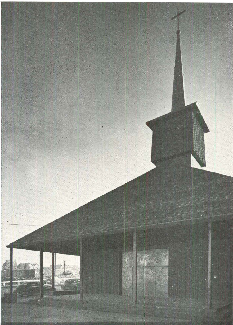
The trim spire emphasizes Zion's presence on its corner site. The entrance door—of copper sheeting decorated with a repoussé design of angels by sculptor Frederic Littman—is inviting behind the broad porch.
