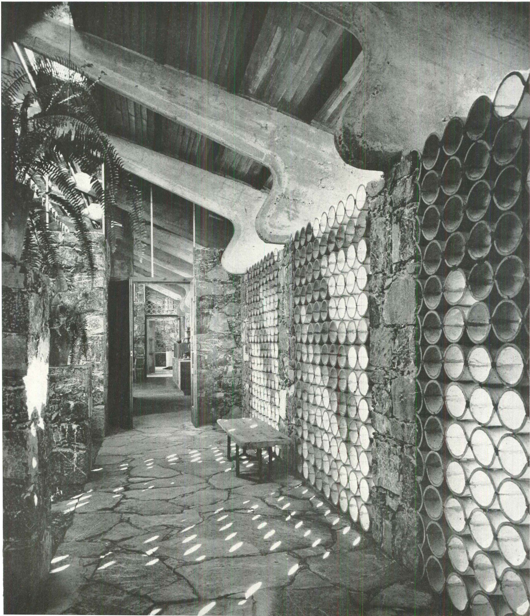
Dining terrace is screened by a grille of tile. Retort-shaped concrete girders cover entire length of main wing, rhythmically articulate the unorthodox structure Maynard Parker
