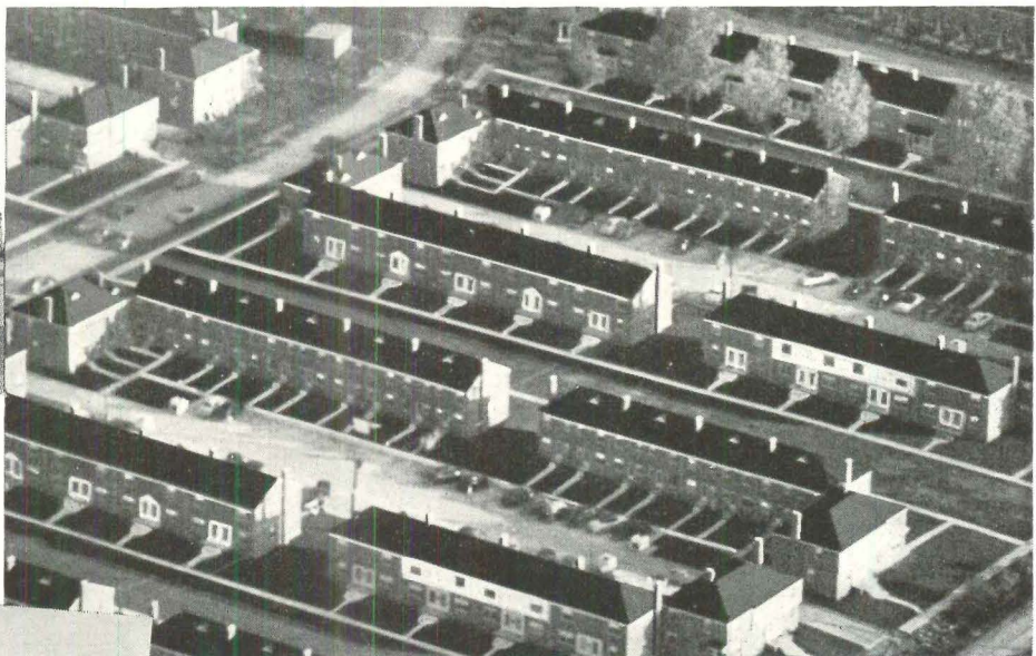
HUNTINGTON GARDENS, Oak Park, Michigan 374 Kelvinator Refrigerators installed! Theo. N. Barthel, Designer; Jos. E. Wassell, Engineer
