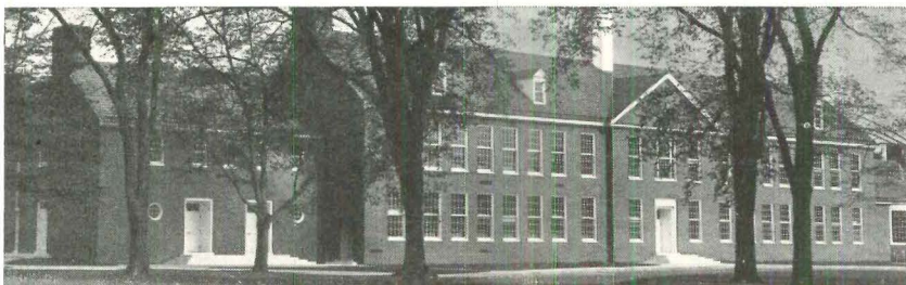
JULIAN CURTISS SCHOOL , Greenwich, Connecticut. Architects: W. B. Tubby, Coffin & Coffin, & Philip N. Sunderland, Inc., Associated Architects. Heating and Plumbing Contractor: Hauxwell & Smith, Inc. Wholesale Distributor: Center Heating & Oil Supplies Co.
