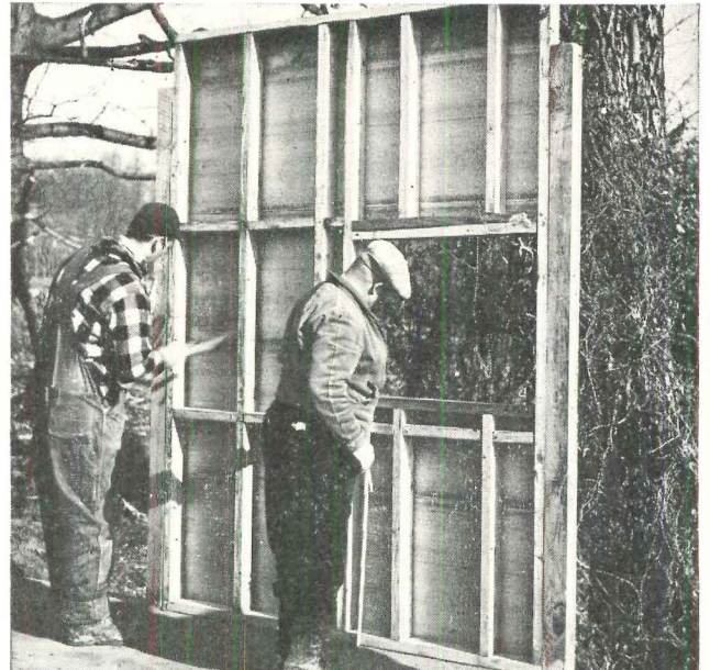
Prefabricated wall panels, with window openings framed-in and insulation attached, are spiked to posts (above). Panels, pre-cut rafters and roof planking go up in a day (below).
