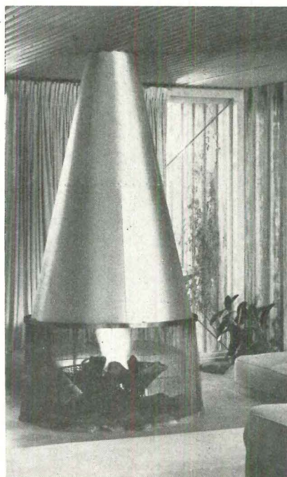
Copper cone flue in Architect Albert Frey's own house is also an effective radiator to counteract night-time chill.
