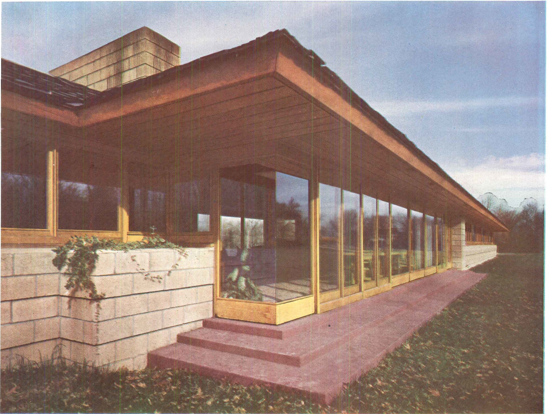
BENJAMIN ADELMAN HOUSE IN MILWAUKEE SHOWS WHAT SKILLFUL HANDLING CAN MAKE OF STANDARD CONCRETE BLOCK. LONG
