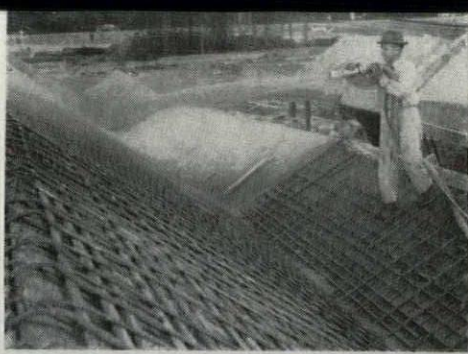
Concrete being gunned on canopy.
