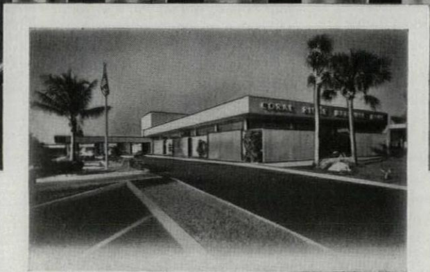
Anotec exterior installation Coral Ridge National Bank, Fort Lauderdale, Florida
