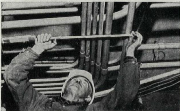
REPUBLIC RIGID STEEL CONDUIT offers highest degree of uniformity and ductility. Threads are clean, sharp, free-running. Welds are smooth, strong. Surface is fully protected by a hot-dip galvanized coating which will not peel, flake, or chip-off under normal bending. To learn more about Republic Rigid Conduit, send coupon.
