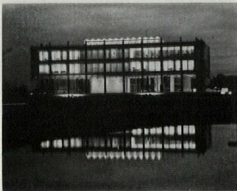
AN ALUMINUM SHOWCASE, which serves as the regional sales headquarters for Reynolds Metals in Detroit, was opened for business last month. It was designed by Architect Minoru Yamasaki.
