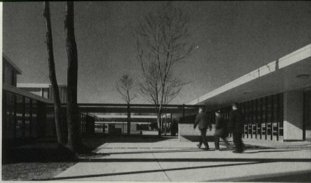
Sweetbriar Elementary School, Smithtown, N.Y. Architects: Ketchum and Sharp, New York City. SPECIAL FEATURES
