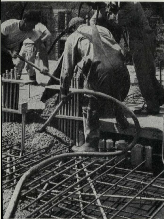
ELECTRUNITE'S tightly adhering galvanized coating protects against corrosion, won't peel, chip, or flake off during bending. Millions of feet have been successfully used in slab concrete installations over the past twenty-five years.
