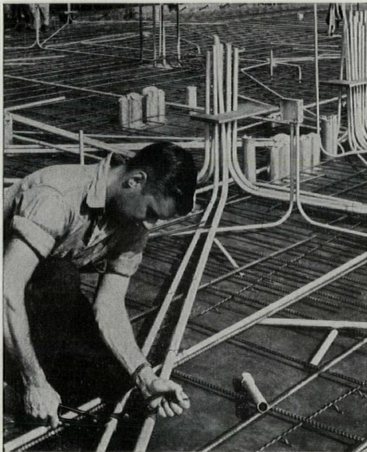
GOOD INSTALLATION PRACTICES call for tying Republic ELECTRUNIT E.M.T. to steel rebars. With steel conduit there is no danger of galvanic action.
