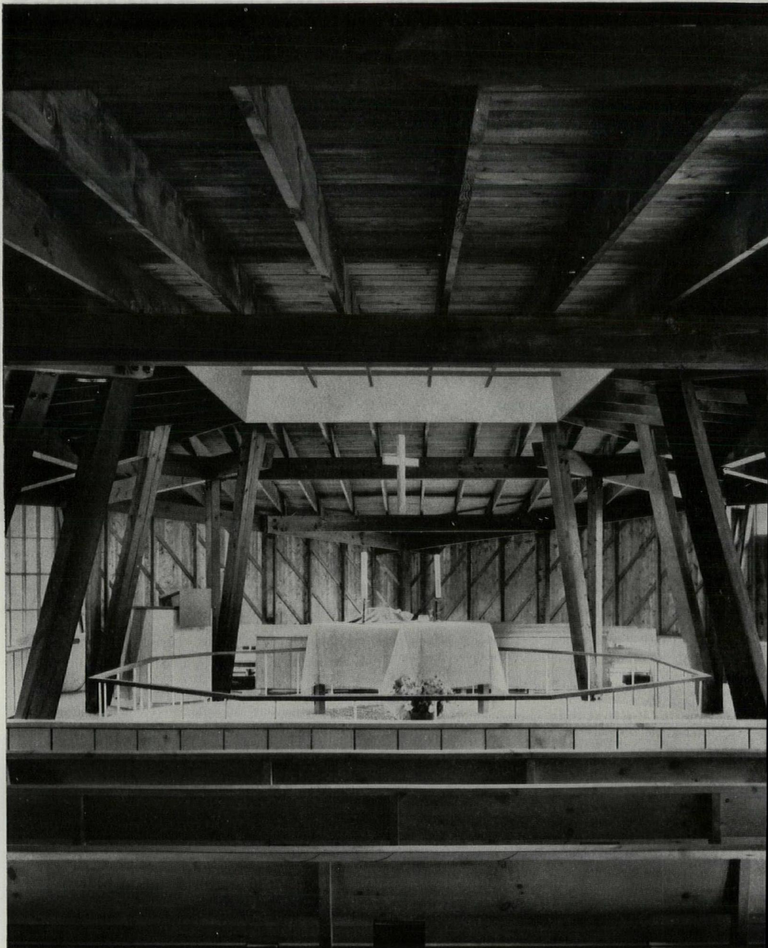
CHAPEL OF ST. JAMES THE FISHERMAN, Wellfleet, Mass.: Two design problems solved by wood's adaptability — the need for a structure allowing every worshipper to share intimately in the service — the desire to evoke something of the character of a stout wood ship. Exposed wood framing and siding suggest a ship's structural honesty — fenestration from above and at floor level creates a luminous atmosphere for devotion. Olav Hammarstrom, architect.
