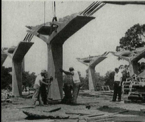
Columns are anchored on steel base plates.
