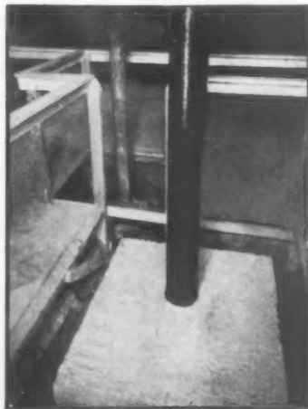
A concrete-filled iron column set in well mixed concrete ensures rigidity of walls and floors
