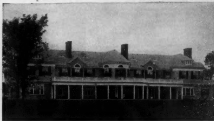
No new shingles, no new stains, no leaks in 36 years. Home of A. S. Bigelow, Cohasset, Mass. Built in 1892 and roof and sidewalls stained at that time with Cabot's Creosote Shingle Stains. All original shingles still in excellent condition.
