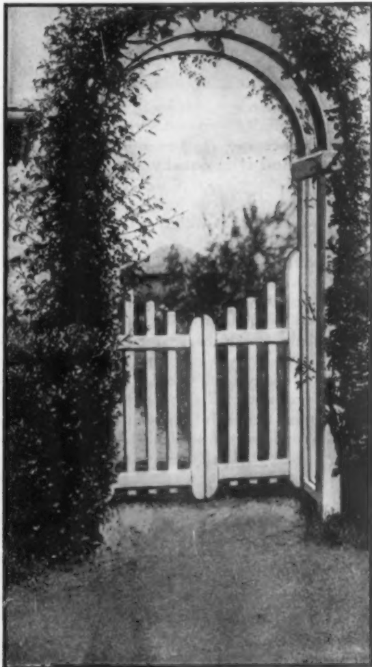
The arbor gateway is an example of heavy self-supporting trellis work with frame members of 2 x 4 inch stock
