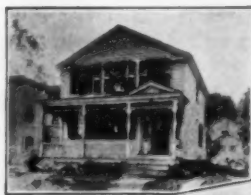
Bottom: the modernized home. Ask about this free Service, and let us tell you how easily WEATHERBEST Stained Shingles can be laid over old wood or stucco sidewalls to give new appearance and better insulation—at a cost less than two paint jobs.
