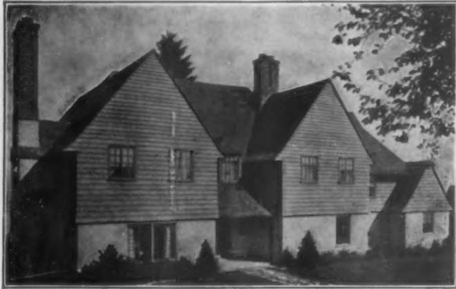
House on Hawthorne Terrace, Portland, Oregon. Architect, Wade Pipes. Contractor Nels Nelson. Cabot's Creosote Shingle Stains on Roof and Siding. Insulated with Cabot's Quilt and trimmed with Cabot's Collopalges
