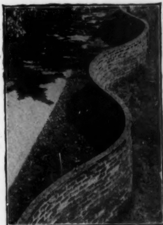
Some say it was because of economy of bricks, that Jefferson designed the single-brick-wide serpentine wall, for the gardens of the Professors at the University of Virginia. But it wasn't. Why don't you have your garden walls and walks made of those Old Virginy bricks of ours?
