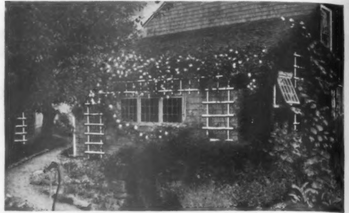
A simple vine support against the side of a house needs no heavy pieces. 1 x 1/4 inch strips may suffice
