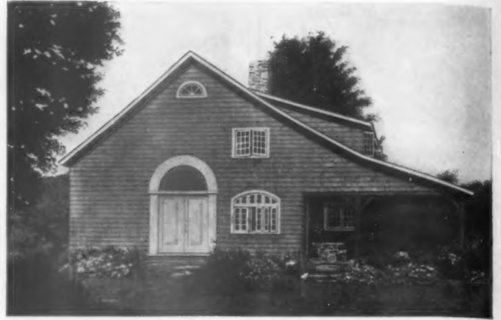
A full front view of "Wolf Pits" showing the carved lunette over the oddly fashioned entrance door. Here also may be seen the unusual roof line with hand hewn and pegged beams
