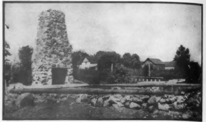
The sill logs and stone chimney, the beginnings of the construction
