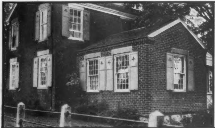
The modern, solid panel blinds which have been installed on this plain old brick house at Lyme, Conn., are really the most important feature of the exterior design.
