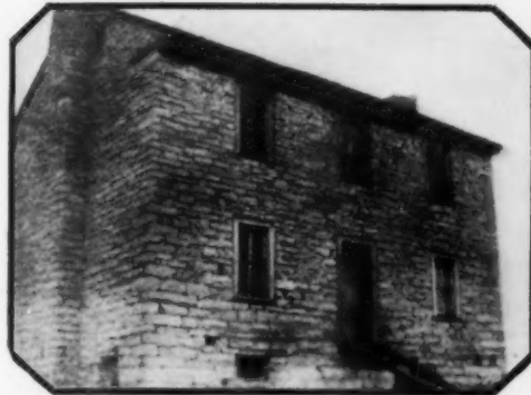
The farmhouse, two miles from Johnson City, Tennessee, as it appeared a year ago. Compare it with the finished house below
