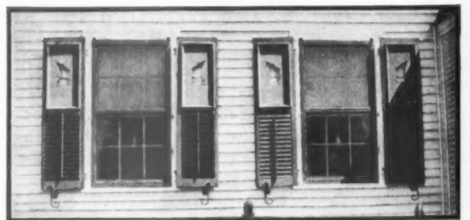
An easy alteration of old-style shutters: the upper section of slats has been removed and a panel inserted which is held in place by small moldings
