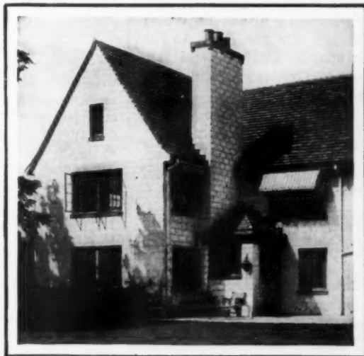
This fine house has exposed masonry walls built of concrete block made from sand and pebbles. Home of H. L. Wallace, Bloomfield Hills, Mich.; M. R. Burrows, Architect, Detroit.
