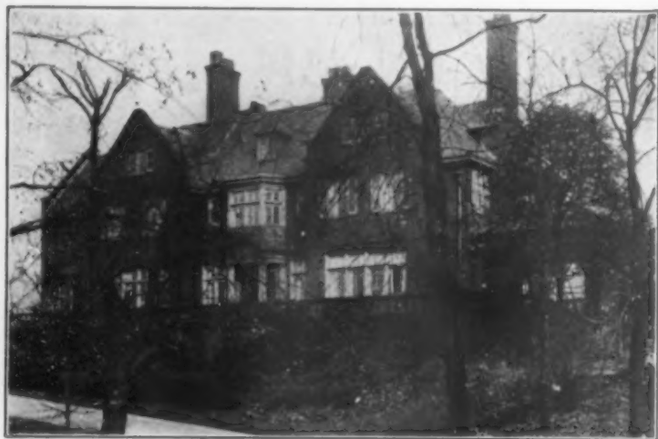
This house on Woodland Avenue, Pittsburgh, is an example of the large, dignified American home of the present day. No reasonable expense was spared, but no better insulator could be found than Cabot's Quilt. Ludlow & Schwab, Architects.
