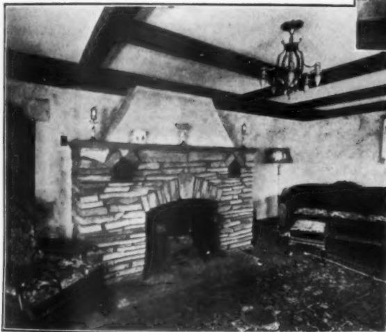
A Heatilator fireplace in the home of Mrs. T. A. Middleton, Pleasantville, N. J. Seward G. Dobbins, Architect. Here the grilles are in the sides of the mantel and cannot be seen from the front. Photo (c) Fred Hess & Son.
