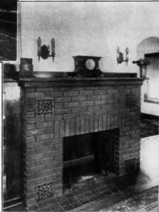
Above amply illustrates The Heatilator Grilles. The lower grilles draw in cold air; the upper grilles send out the same air, intensely heated. In ordinary fireplaces this heat is entirely lost in the masonry or up the chimney. In the Heatilator fireplace, even the direct heat from the fire is apt to be greater than in an ordinary fireplace, because of the scientifically correct design.
