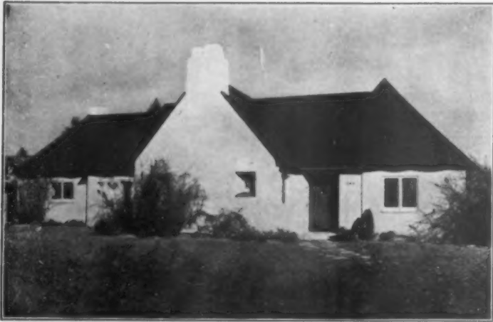
House at Beverley Hills, California. Witmer & Watson, Architects. Roof stained with Cabot's Creosote Shingle and Wood Stains, and walls finished with Cabot's Collopackes (DOUBLE WHITE).
