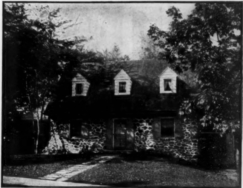
The home of Mr. Harry Steifle, of Summit, New Jersey. Designed by D. Wentworth Wright, Architect
