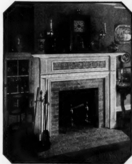
A restrained architectural note in a mantel which frames a row of old Dutch Biblical tiles in delft blue. These appear as a characteristic fireplace embellishment in some of the oldest of our houses
