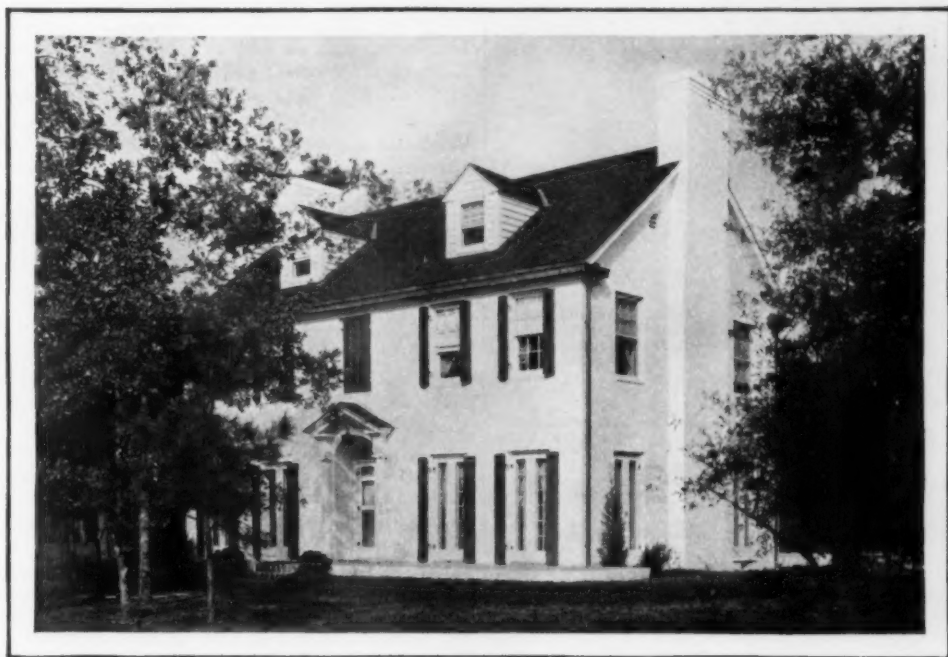
Home of W. W. Porch, River Oaks, Houston, Texas. Charles W. Oliver, Architect. Concrete masonry construction, with white portland cement stucco exterior.
