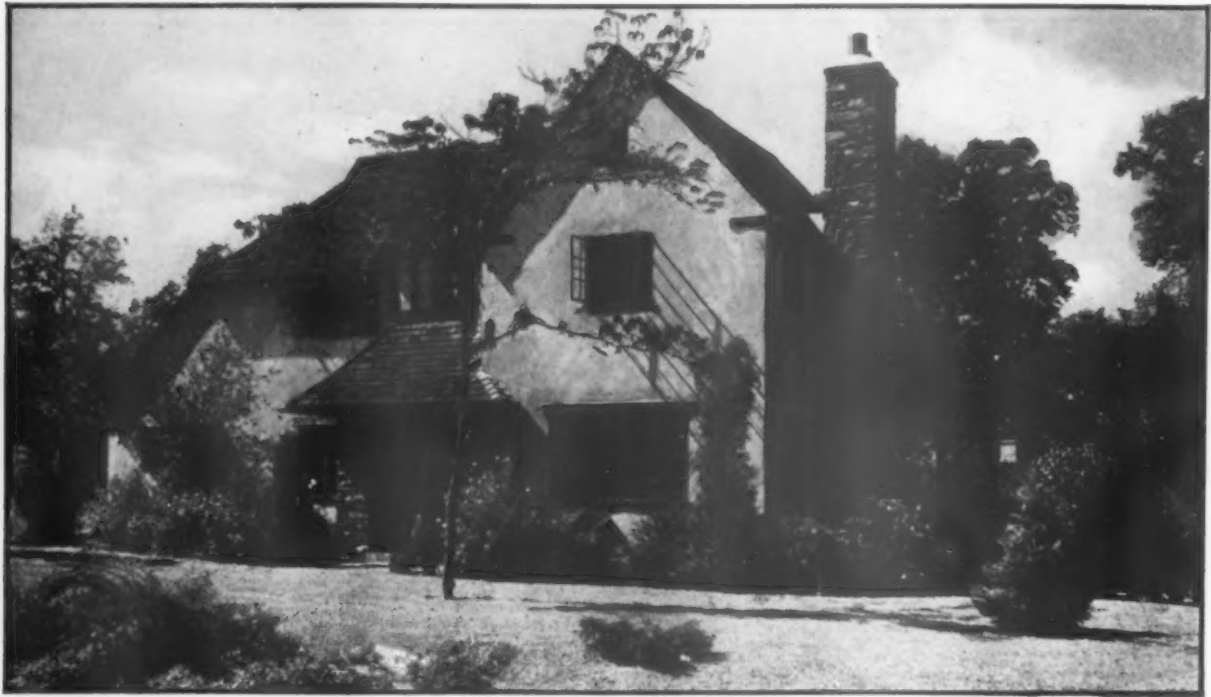
Mellow coloring and long roof lines make this lovely home of Mr. Foster Gunnison, of Bronxville, N. Y., merge into its well-planted surroundings. The stucco is buff-tinted; the window casements, dull red. The house was designed by Oscar Valet and cost $13,000 to build
