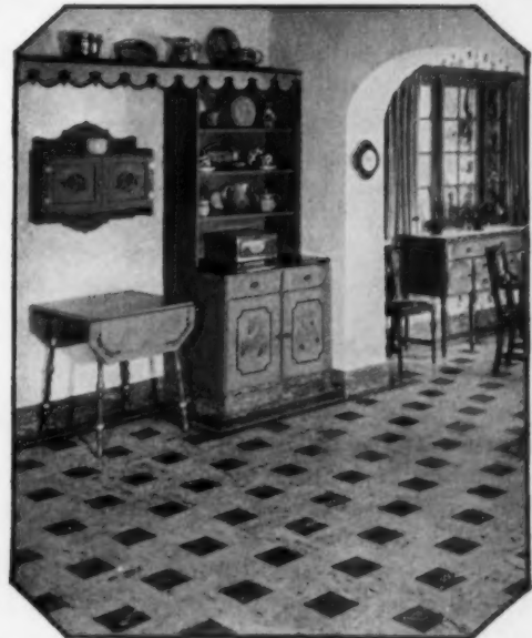
Rubber tiling, laid in individual tiles, can be worked out in pleasing designs. It is particularly resilient (Courtesy of Goodyear Tire & Rubber Co., Inc.)
