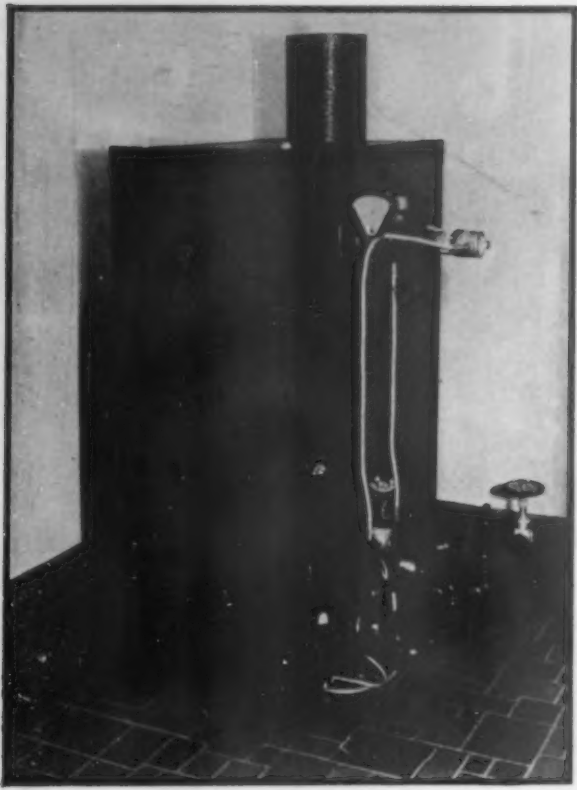
Experts are agreed that gas heating is efficient and practically automatic. In those sections of the country where gas rates are low, such a boiler as the one shown above, with a covering which completely hides the valves, is always popular
