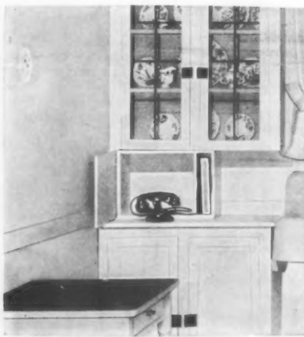
An additional line for the use of servants may conveniently be installed, with extension telephones in the kitchen, butler's pantry, and service quarters.
