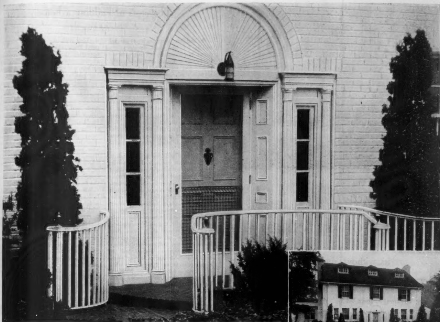
ENTRANCE TO THE HOME of Judge William E. Hirt, at Erie, Penn. Brick as well as wood homes are made more beautiful by painting with Outside Barreled Sunlight.
