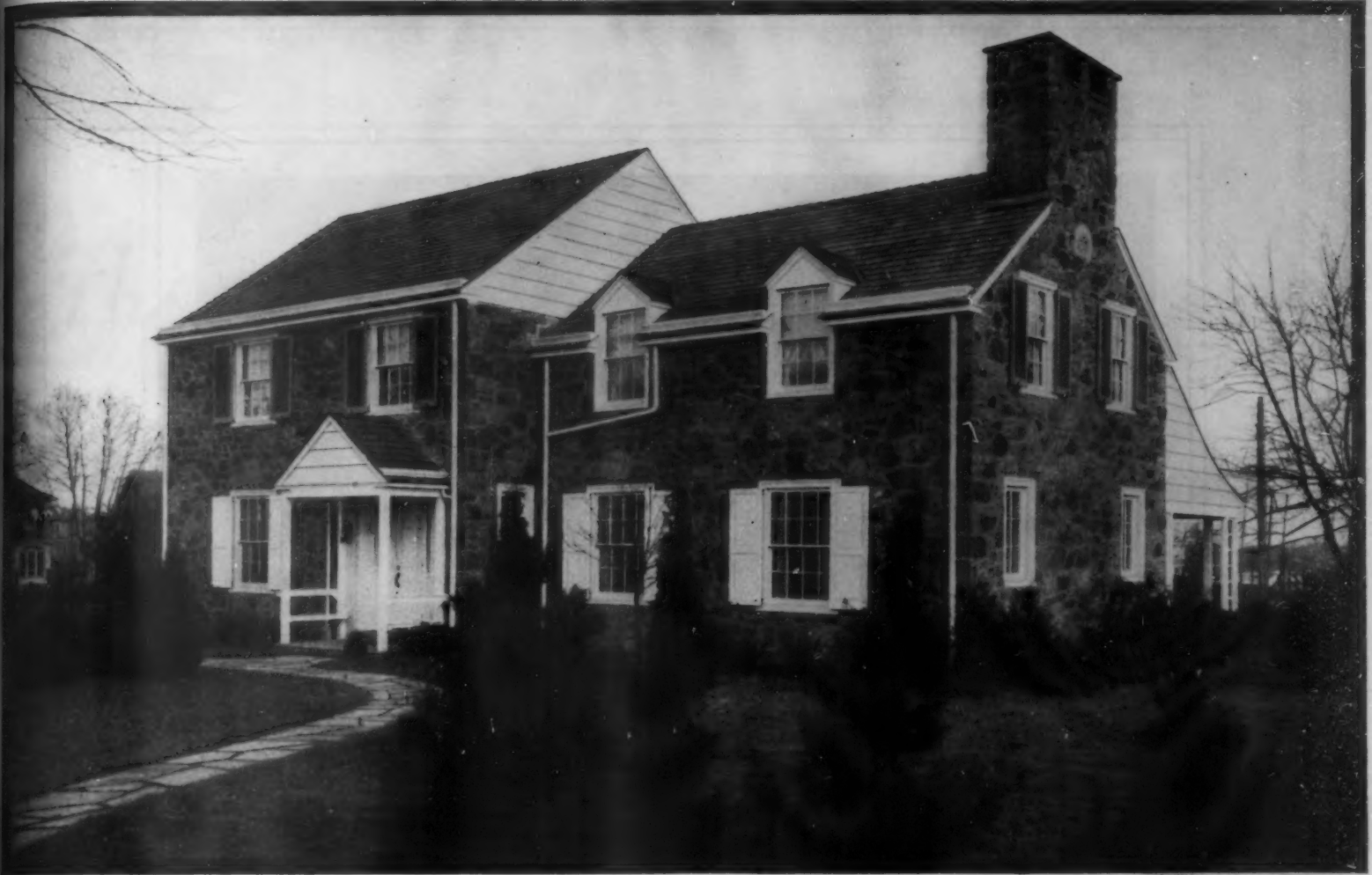
Among the authentic details which add charm to this Colonial residence is a complete equipment of Sargent Hardware. Richard W. Meeaskey, architect; J. Craig Janney, associate, Philadelphia.
