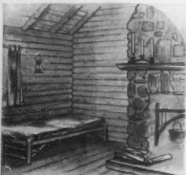
The year 'round lodge of the Hennepin County Girls Scouts is built with Shevlin Log Siding. Edwin H. Hewitt, Minneapolis, architect. Libbey & Libby, contractors.
