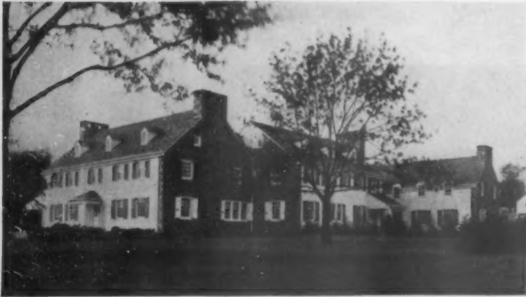
New country house in Penn Valley, Pa. Builder, Frank H. Mancill, Philadelphia. Cabot's DOUBLE-WHITE, Old Virginia White, and Green Gloss Collophane on all exterior woodwork. Insulated with Cabot's Quilt in walls and roof.
