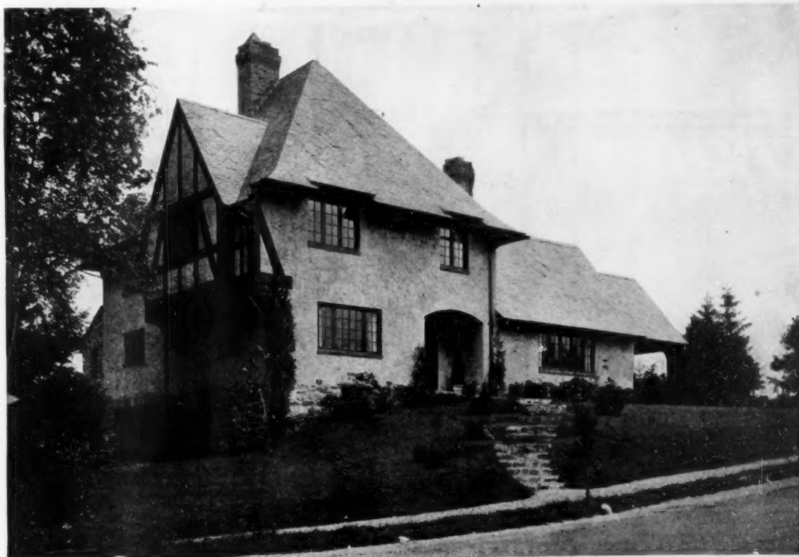
Two views of a residence in Sunny Ridge, Harrison, N. Y. Walls of concrete masonry, with portland cement stucco exterior. Julius Gregory, New York City, Architect.
