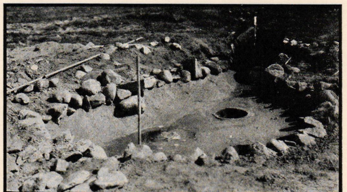
Semi-formal type of pool in the author's garden near Grand Rapids, Michigan, built according to the details explained herewith. The photograph below shows the stage of construction when the walls had set and the first row of stones were in place
