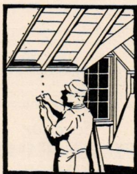
Item 83 on page 356 suggests the use of insulating boards or plaster for lining an unfinished attic space, thereby creating an extra bedroom or recreation room
