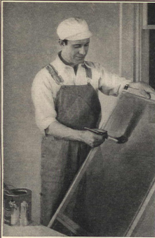
SCREENS THAT RUST . . . require frequent painting.
