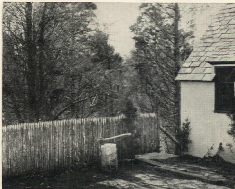
The woven rustic fence is made up of chestnut or cedar saplings placed side by side and held by wire woven in and out of the saplings. This type of fence insures privacy and adds a decorative note to a country home. (DuBois Fence and Garden Co.)
