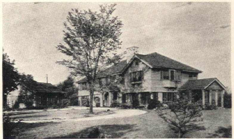
Residence at Fox Point, Wis. Furber Libby and Alfred Gillman, Architects, Milwaukee. Roof and walls stained and preserved with Cabot's Creosote Shingle and Wood Stains.
