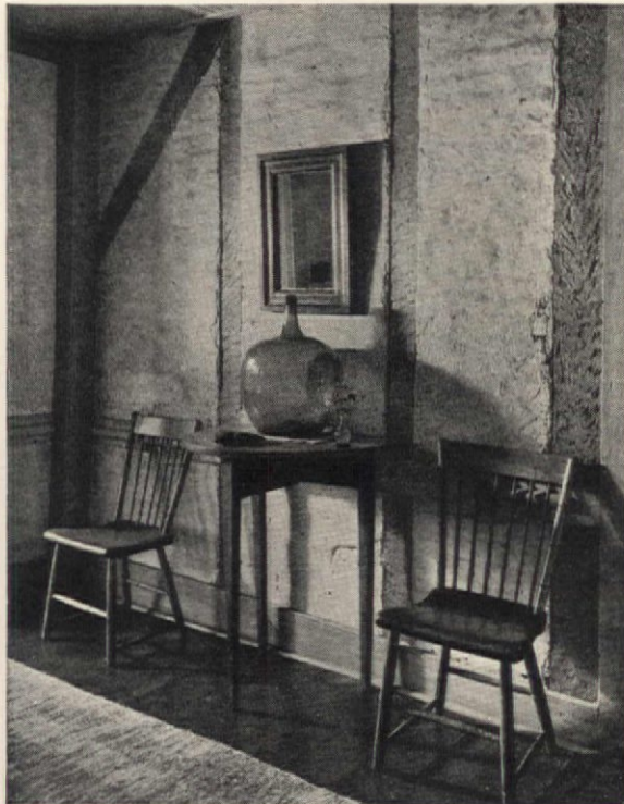
Left: The hallway, which shows the black walnut framing of the house, brick filled, and accounts for the sturdiness of our two-century-old house
