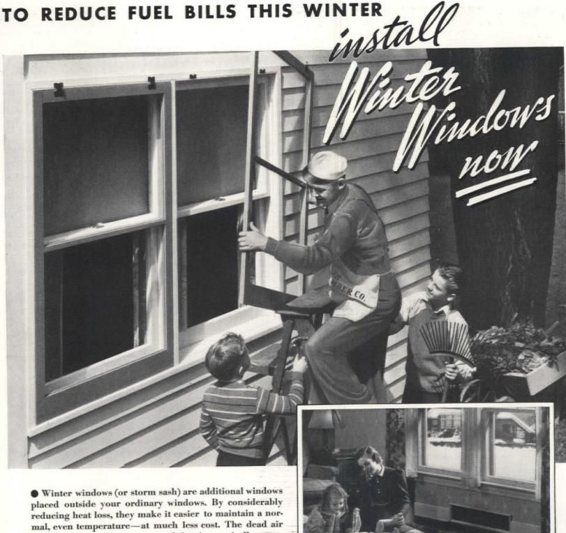
formed between the two panes of glass is practically a nonconductor of heat. . . Thus, the scientific principle of the thermos bottle is applied to your home.
