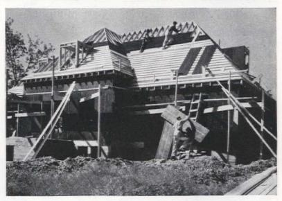
This house is sealed with Fir-Tex inside and out! It is the residence of W. W. McCready in Forest Grove, Oregon; D. W. Edmundson, architect. Above: Fir-Tex Sheathing is nailed to the walls and roof; notice the asphalt coating, which keeps out rain and moisture. Below: Plastering over Fir-Tex insulating lath in the McCready home. This solid base prevents lath marks, plaster cracks are minimized. Fir-Tex insulation drastically reduces heat bills.
