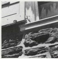
LIMBING vines can cover a multitude of architectural faults but don't let them run away with the house. Particularly when it's a stone house and they get strong enough to pull out mortar from between the stones. Look out for crevices and fissures caused by shrinking, drying window frames, too, before they need expensive caulking and repointing and before they're large enough to cause real heat loss in the house.
