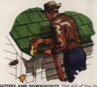
CLEAR GUTTERS AND DOWNSPOUTS. Get rid of the debris that interferes with proper drainage. Cover downspout openings with wire mesh to keep channels clear of rubbish. Where repairs are needed, call in your local sheet-metal man to put them in shape.
