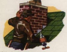
WHAT ABOUT FLASHINGS? Are they tight? Is the pointing gone or crumbling? Any danger of leaks? Check up ... and if flashings are loose, push them back into place and repoint them with elastic roofing cement or caulking compound. Look particularly at flashings around chimneys.
