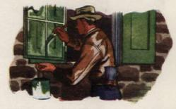
TAKE CARE OF STEEL CASEMENTS. With a little attention, they'll serve you faithfully for life. Wherever moisture or seepage threaten deterioration, clean with a wire brush, paint with red lead followed with a good house paint. Caulk
