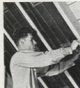
And here's how neatly KIMSUL is installed in sloping attic roofs. Stays put, too, once properly installed. Rows of strong stitching run through KIMSUL blanket, prevent sagging, sifting, settling.
