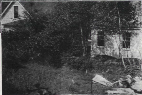
1 YEAR saw this change from a rough, rocky hillside to a concreted picnic terrace beside a wading pool—all within 50 feet of the house
