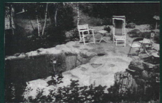
The Higginsholm wading pool is unique in that it was erected, not excavated! A rim of boulders was built on the ledge; the resulting depression was filled with concrete
