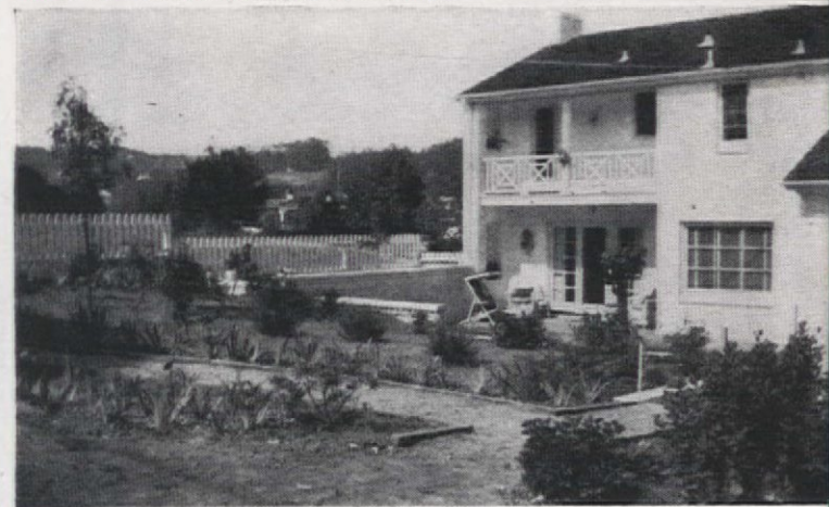
These three views toward the rear of the house show what happened between March, 1958 and 1941
