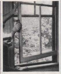
For stubborn sash, remove from frame, and plane both upright edges-if trouble still persists, paint edges with linseed oil or rub up and down with candle stub
