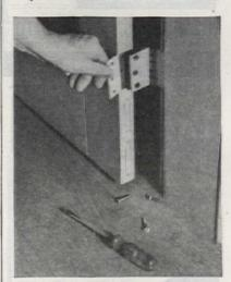
If door hangs unevenly, loosen proper hinge-insert heavy piece of cardboard to take up slack
