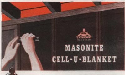
Cell-U-Blanket comes in various widths to fit spaces between studs or rafters. Lengths are cut with shears, stapled or tacked in place, can be overlapped to make a complete heat and vapor barrier that will not shrink or settle. Cell-U-Blanket is available for your new or remodeled home — in addition to its many war jobs.
