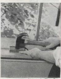
Tap on flat block of wood with hammer along side strips and sill of window if old or new paint is cause of the sticking sash
