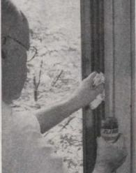
Proper method for applying oil or slipping compounds to sash grooves. If forcing sash with hammer or chisel, always work from outside so that any marks will not be visible on the room side
