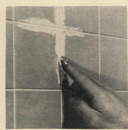
"Grouting" between tiles beautifies and waterproofs joints. Grout is a thin mortar made with cement. Clean out mastic between tiles with a thin stick or putty knife. Apply grout to joints with fingers, press firmly to avoid air pockets beneath surface. Do only one or two tiles at a time. Remove excess with a damp sponge or soft cloth. Wipe diagonally across tiles
