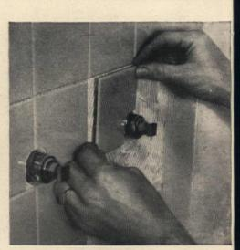
Cut tile to fit around pipe and fixtures. Use a coping saw for plastic tile; a hack saw for metal tile. As fixtures and pipes usually have a chrome ring around them, accurate fitting is not essential
