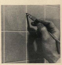
Run rubber eraser on a pencil down between tiles. This makes grouting clean and even. With a damp sponge, remove any excess eraser may work up to surface. Be very careful not to mar grout line
