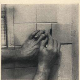
You'll have to cut tiles for corners. To mark tiles for cutting, place one tile squarely on top of last set tile near corner. Place another tile over this loose one, but move it out to butt against corner. Top tile acts as a straight-edge guide for marking cutting line on first loose tile placed over set tile. Use tile cutter, coping saw, or electric jig-saw to cut tile
