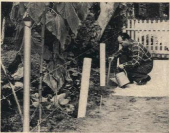
Determining our property line, we stretched two cords along it, the upper one to mark height, the lower one to insure alignment of the 4 x 4 cedar posts which we set 8 ft. apart on centers in holes dug with rented two-handled scoop. Soil was soaked and tamped firm
