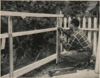
To align tops of pickets, we let each one touch a 9 ft. 2 x 4 guide frame, one end of which rests on picket last nailed in place, the other end on a picket nailed, temporarily, at proper height 9 ft. away. Loose picket hanging in foreground is "spacer" (see text)
