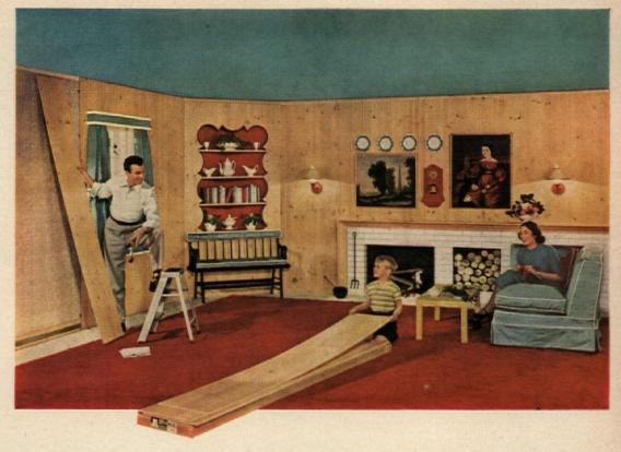
height in 161/4" width. Panels are factory-finished... no painting or staining is needed. Concealed metal clips hold Plankweld to any interior wall... plaster, wood or wallboard... without visible nailing.
