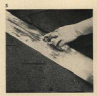
Remove excess roofing cement from valley flashing, for it will form a small dam and allow water to back up under roofing
