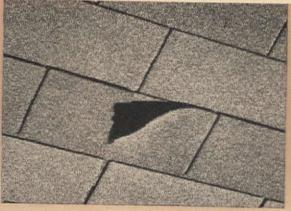
Torn shingles can be caused by the same factors that account for loose shingles or by heavy objects such as branches falling on roof. They should be repaired at once, for strong winds will make them worse
