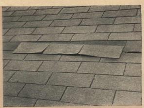
Improperly or inadequately nailed shingles can be pulled loose by a driving wind or an accumulation of ice and snow. Working on the roof in hot weather when the shingles are soft will also tear them loose
