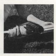
Life of downspouts can be lengthened if inside is swabbed out with cloth saturated with asphaltum paint
