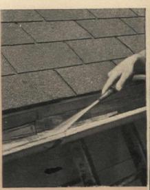
Gutters should be hosed down from time to time to remove thin deposits of soot that become highly corrosive to metal when damp. This also gives you a chance to check gutter for proper pitch
