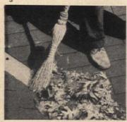
Sweep valleys clean and inspect them for signs of rust and holes. Repair these with a thin coat
