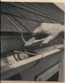
utters should have uniform slope towards ownspout. They can be adjusted by ending hangers. Make sure that outside dge of the gutter is lower than the utside edge of the roof
