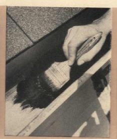
Asphaltum paint makes a good protective finish for both wood and galvanized-iron gutters. Aluminum, stainless steel, and copper gutters don't require this kind of protective finish
