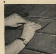
Leaks in wood-shingled roofs can be easily fixed by slipping a piece of copper up under the shingle at point of leak
