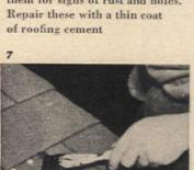
Replace rusted nails with roofing nails that will not corrode. Coat head of nail with a dab of roofing cement
