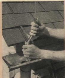
Clogged downspouts can be cleaned out by a coil spring-steel auger of the type used for clearing obstructions in the house drainage system. Flush downspout with hose after removing obstruction
