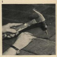
Wood shingles that are loose or have warped should be nailed into place with galvanized shingle nails. Coat nail head with cement
