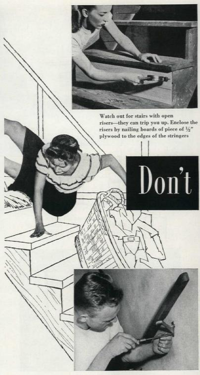
All stairs should be equipped with a handrail, and it should be on the right as you descend. Make sure that the rail is securely fastened with screws to the wall studding
