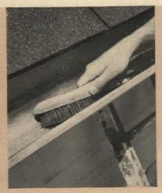
Dirt and rust, etc., can be removed by brushing gutters with a stiff wire brush. Galvanized-iron gutters won't rust if the inside is painted with a metal primer followed by outside paint
