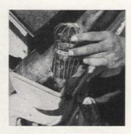
Downspouts should be fitted with a small metal strainer where they enter gutters—this will keep solid matter from getting into them
