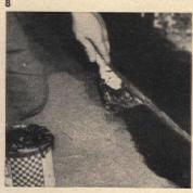
Inspect the edges of flat roofs where roofing joins metal trim, and apply roofing cement where
