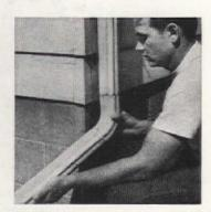
Extend downspout to underground clay pipe to carry water from the house to a dry well or storm sewer
