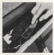
When patch is in place, apply a thin coat of roofing cement to the surface and smooth out with putty knife. Be sure compound covers edges of patch
