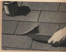
A tear or leak can be repaired by applying a thin coat of roofing cement to the shingle below, and then slipping a piece of copper or heavy roofing paper up the torn shingle
