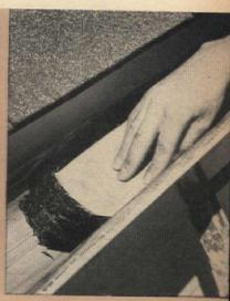
Cut a patch from canvas or heavy roofing paper. Make it more than large enough to cover damaged area, and force it into roofing cement on gutter
