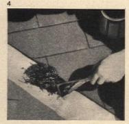
Leaks at seam between valley flashing and roofing can be closed with roofing cement applied under shingles
