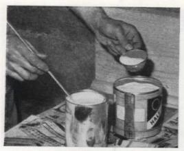
A flight of steep stairs can be made slipproof if the treads are painted with porch or deck enamel to which fine beach sand has been added. Keep paint well stirred during application
