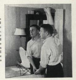
Push the clips on the top bracket up, and then set the bottom edge of the mirror in the felt-padded lower-bracket clips. Large-size mirrors should be handled by two persons. Push the top of the mirror against the wall, and then push down the two clips at the top
