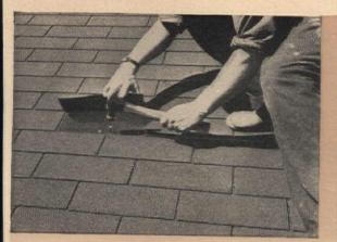
To renail the loose shingle, nails on the lower portion of the shingle above must be carefully removed. Push the loose shingle back into the correct position and then renail both shingles using asphalt shingle nails
