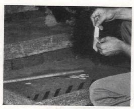
Outdoor steps are almost certain to become slippery when they are wet. An easy remedy is to lay strips of adhesivebacked non-skid tape over the treads
