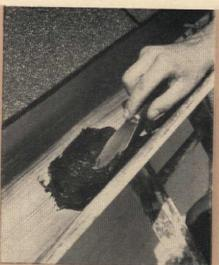
Leaks in a gutter should be patched immediately, for they cause stains to appear on the walls of the house. First, apply a coat of plastic roofing cement to the area around the leak
