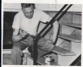
An inexpensive railing for stairs can be made out of 1½" galvanized or wroughtiron pipe. Plumbing-supply stores will cut and thread the pipe and supply the fittings
