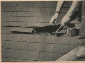
Shingle can be fastened in place by cementing it to the shingle below. Put a couple of dabs of roofing cement or compound on the shingle in the lower course and then press the raised shingle down into place
