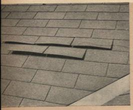
Asphalt shingles on low-pitched roofs may be ruffled up by driving winds that force rain and snow up under the roofing where they create leaks damaging to inside walls and ceilings
