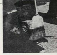
Wash broom clean with water. If bristles have become stiff, use kerosene, then water. Moisten primed surface with fine spray, but do not allow standing water to remain. Keep entire surface damp as paving material is applied
