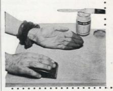
To locate rough spots that need further sanding, slip an old nylon stocking over your hand and run it lightly over the area you have sanded. Any spots that are still rough will snag the stocking and indicate the need for further sanding
