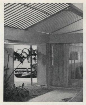
House makes own breezes. Passage formed by corners of house and garage is shaped to provide constant air flow; folding doors help control air volume and velocity. Slat roof shields living room and lanai from hot sun
